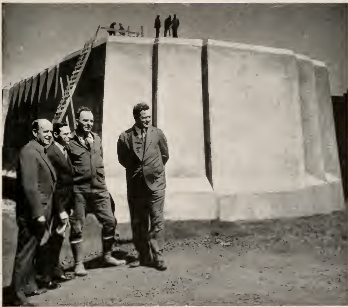
"Golden Gate" Cement used.
