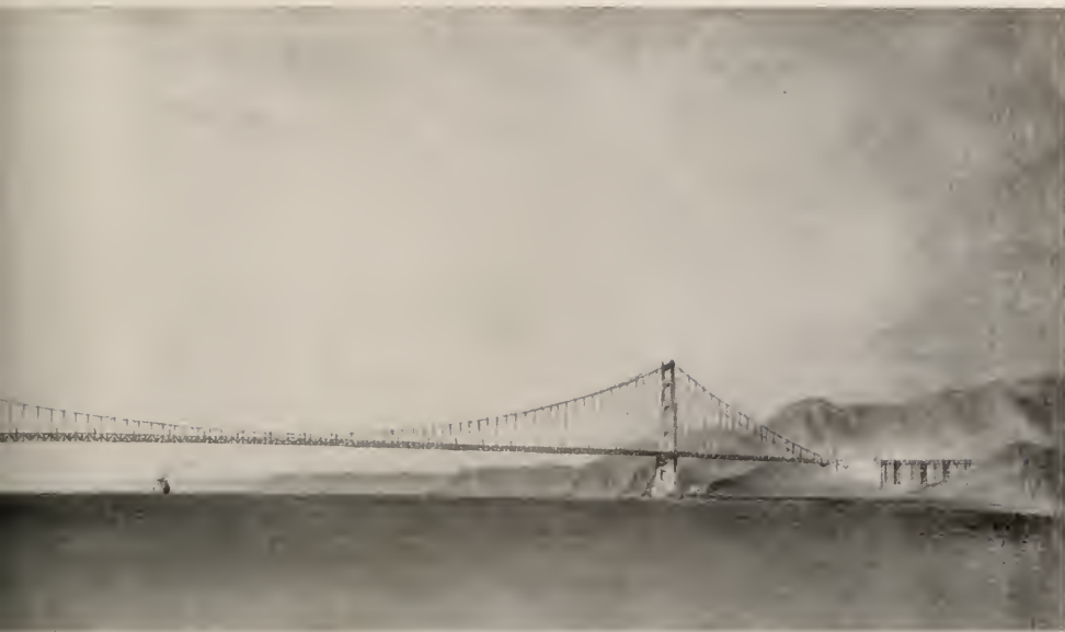
WITH A SINGLE CLEAR SPAN OF 4200 FEET, LONGEST SPAN IN THE WORLD
