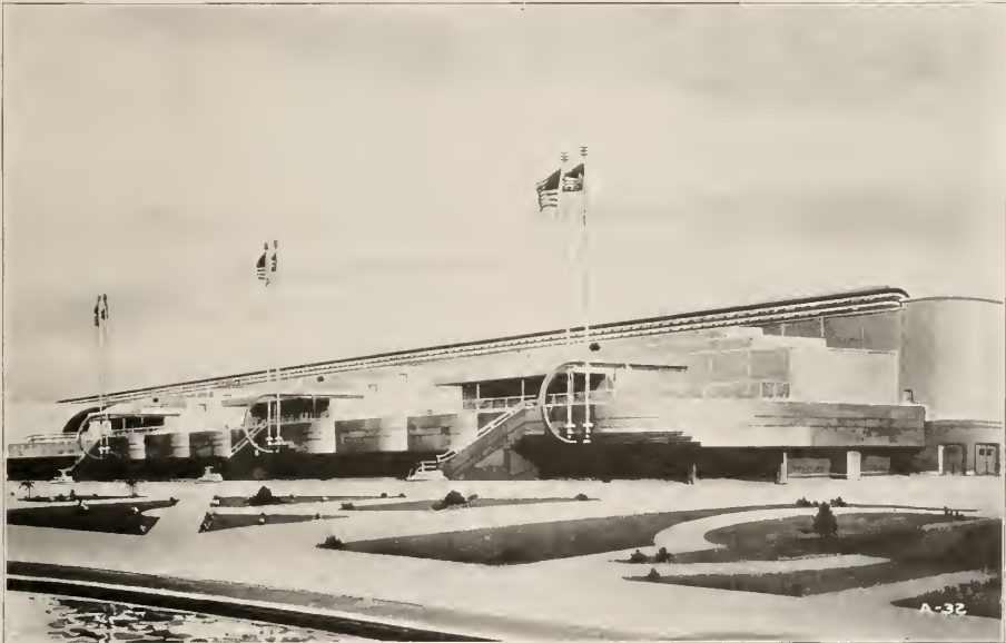
AGRICULTURAL BUILDING Edward H. Bennett and Arthur Brown, Jr., Architects
