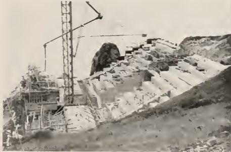
CABLE ANCHORAGE, MARIN SIDE, GOLDEN GATE BRIDGE
