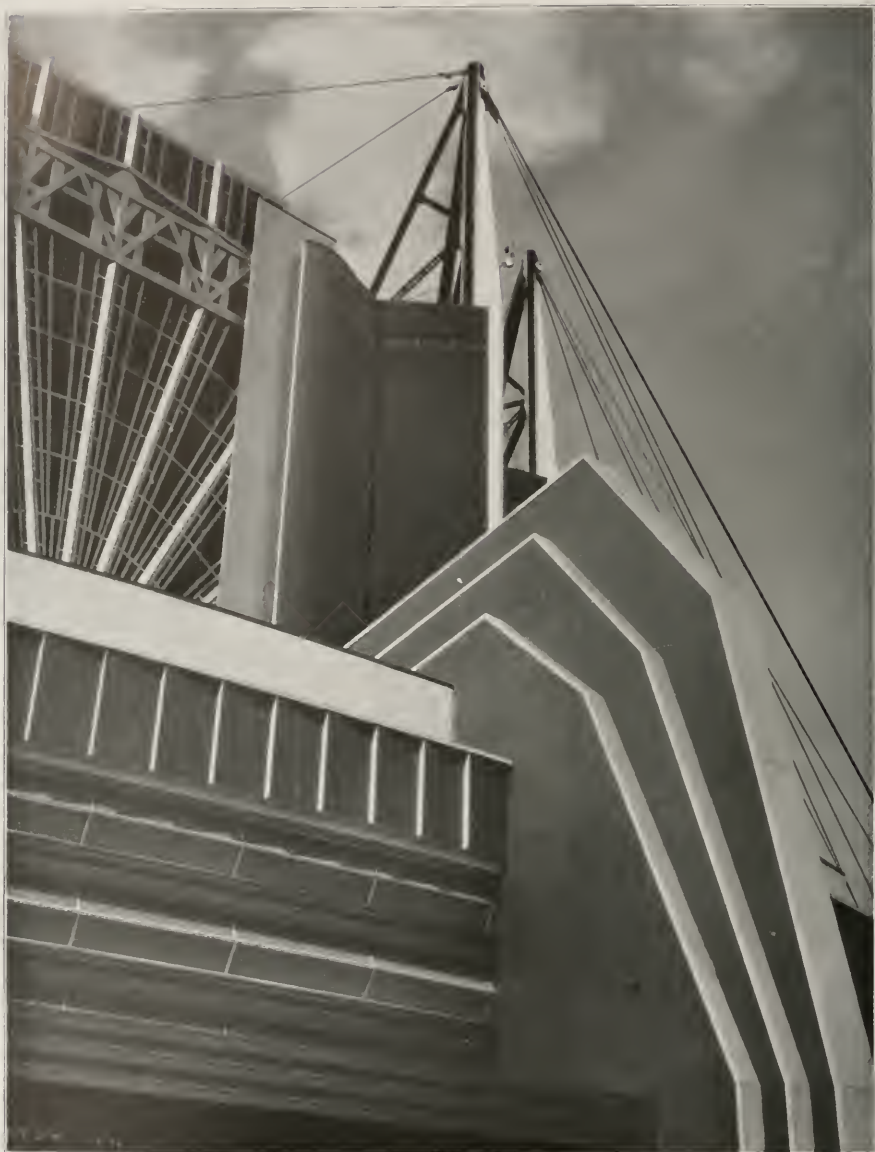
DETAIL OF TRAVEL AND TRANSPORT BUILDING EDWARD H. BENNETT, HUBERT BURNHAM AND JOHN A. HOLABIRD, ARCHITECTS
