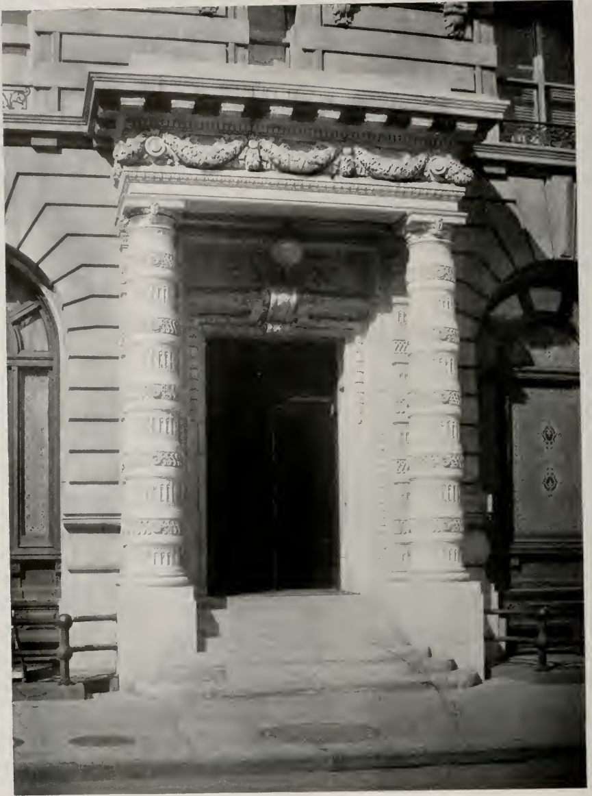
DETAIL OF ENTRANCE, HOTEL ESSEX, PARK AVENUE, NEW YORK HOWARD AND CAULDWELL, ARCHITECTS
