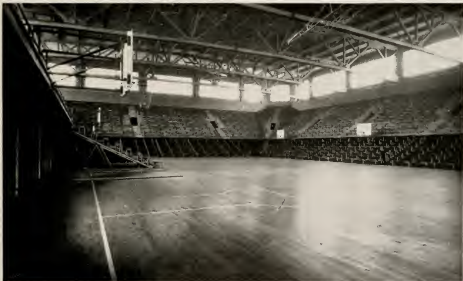
ARENA FOR BASKET BALL, GYMNASIUM FOR MEN, UNIVERSITY OF CALIFORNIA George W. Kelham, Architect
