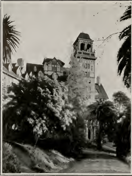
CLAREMONT HOTEL, BERKELEY, CALIFORNIA C. W. Dickey, Architect
