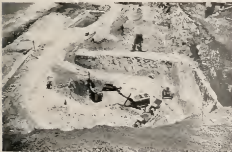
EXCAVATING FOR CABLE ANCHORAGE SAN FRANCISCO SIDE
