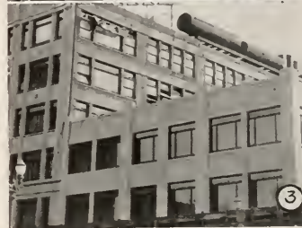
The three views above show a large -core building in which a 3-story wing has been reconstructed with reinforced concrete exterior walls and plaster finish, applied to blend in color and appearance with the exterior facing of the main building. (1) Walls being cast in the forms. (2) Removal of form. (3) Completed exterior.
