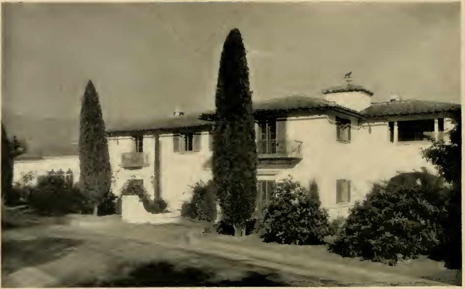
RESIDENCE OF C. B. PIPER, PASADENA, CALIFORNIA Robert H. Ainsworth, Architect
