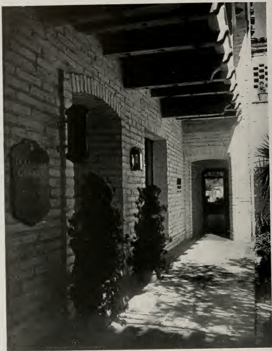
DETAIL OF PALMER SABIN BUILDING, PASADENA, CALIFORNIA PALMER SABIN, ARCHITECT
