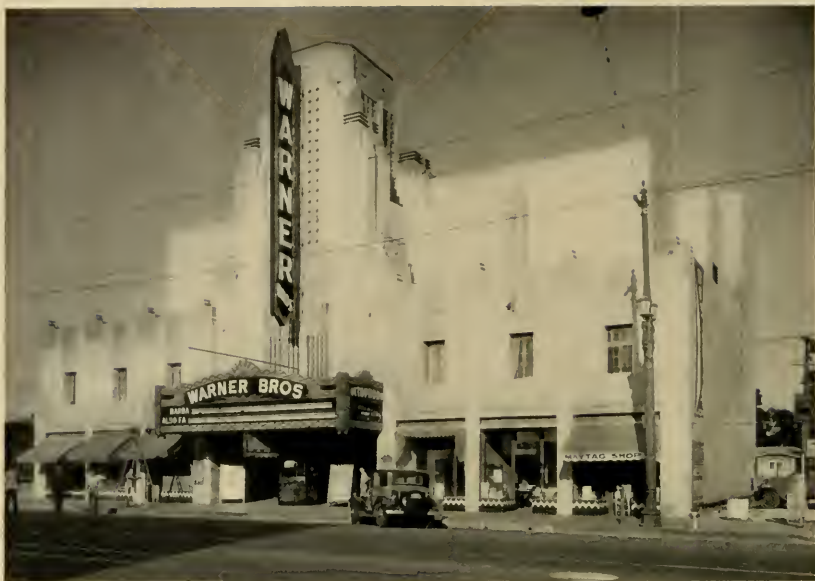
WARNER BROS. THEATER, HUNTINGTON PARK, CALIFORNIA Building is of reinforced concrete and was undamaged by the earthquake of March 10th, 1933. Signs in front announce auditorium safe for occupancy by order of Municipal Building Department. Photograph taken after the quake.
