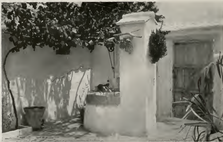
WELL HEAD IN PATIO OF SMALL HOUSE, PALMA DEL RIO
