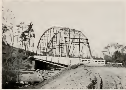
PRACTICAL ECONOMY IS REPRESENTED in this old Mad River Bridge moved to a new location, abolishing four railroad grade crossings.
