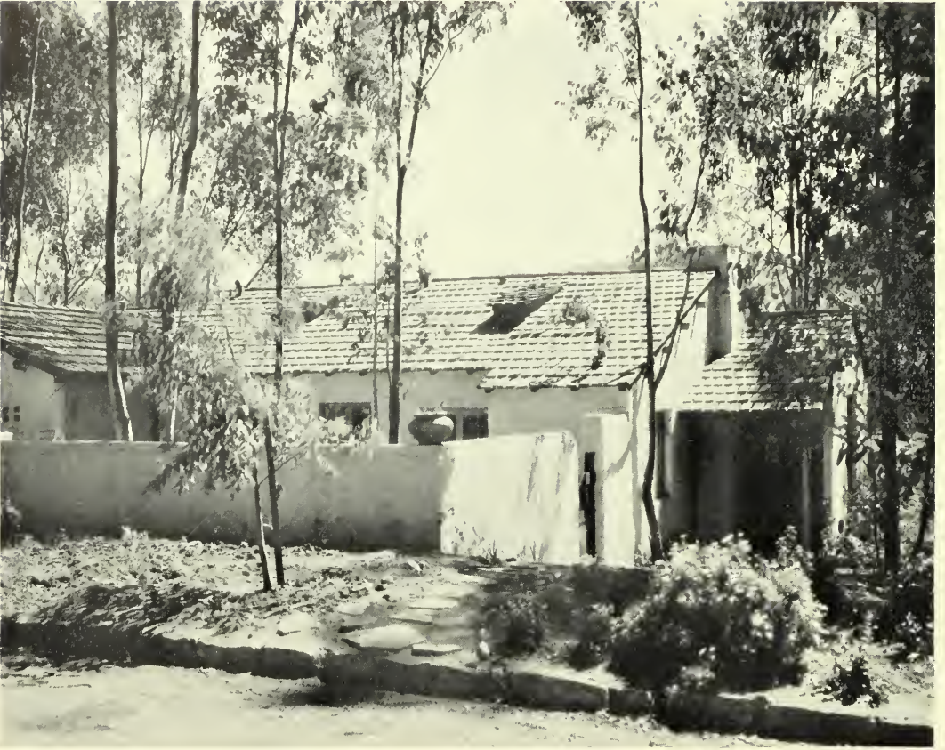
NORTH FRONT, RESIDENCE OF MRS. CAROLINE JOHNSON, PALOS VERDES ESTATES Arthur C. Munson, Architect
