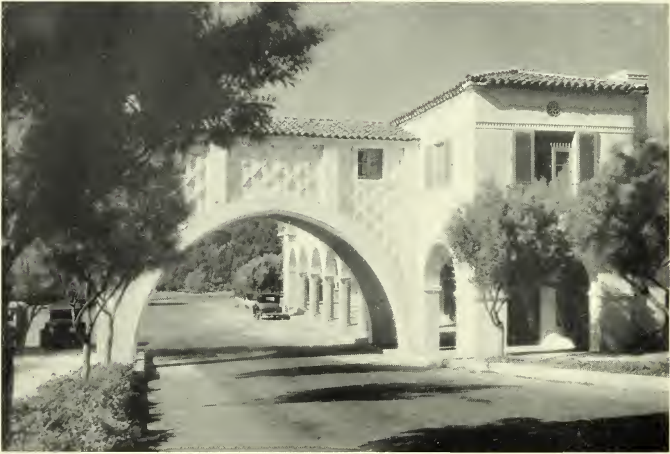
SALLY PORT OVER VIA CHICA AND CASA DEL PORTAL, PALOS VERDES ESTATES Webber and Spaulding, Architects
