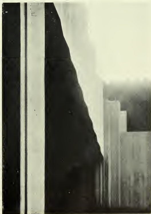
DETAIL, COURTYARD, STUDIO BUILDING, LOS ANGELES
