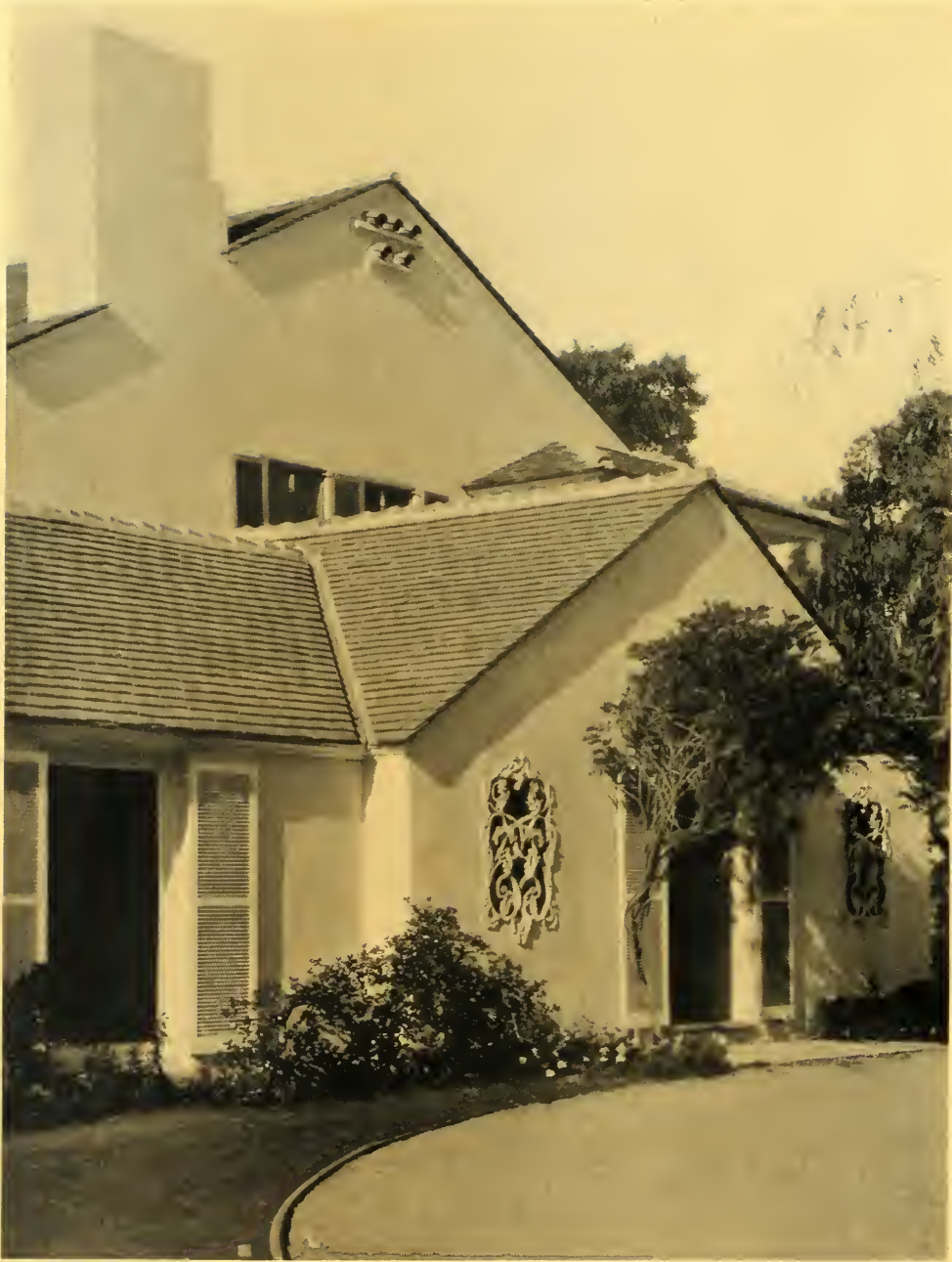
ENTRANCE DETAIL, HOUSE OF LITA GREY CHAPLIN, BEVERLY HILLS ROY SELDON PRICE, ARCHITECT
