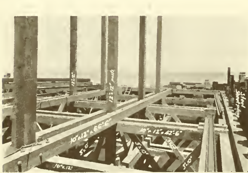
FIG. 3—INTERIOR BRACING AND STRUTTING
