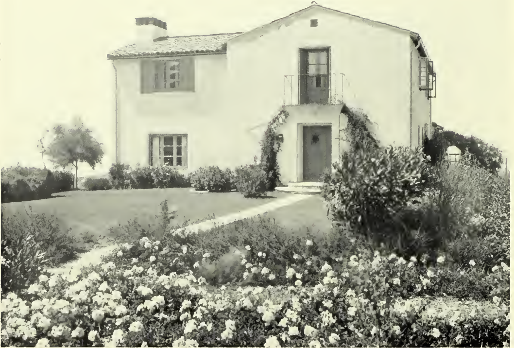
EAST FRONT, RESIDENCE ON GRANVIA LA COSTA, PALOS VERDES ESTATES Winchton L. Risley, Architect
