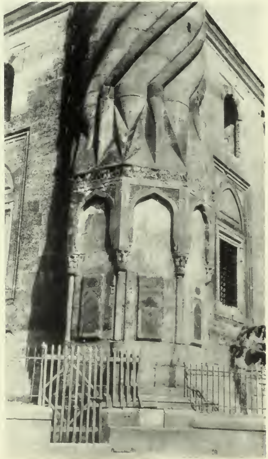
BASE OF MINARET
