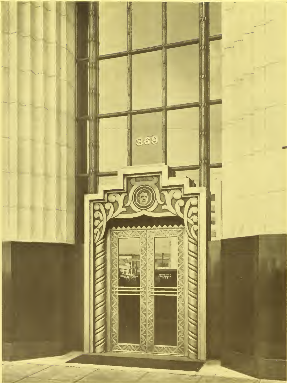
PRESENTING A SOLID FRONT, TESTIFYING TO THE SECURITY OF THE INSTITUTION, AND TO THE INTEGRITY OF THE FOUNDER; THESE IDEAS SEEM CLEARLY TO BE THE FUNCTION OF THIS CAST IRON PLATED DOORWAY TO CENTRAL BUILDING & LOAN ASSOCIATION, OAKLAND, WILLIAM E. SCHIRMER, ARCHITECT. JOHN STOLL, SCULPTOR.
