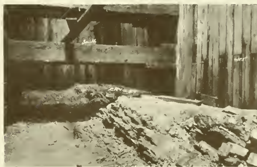
FIG. 4—BED ROCK IN COFFER DAM
