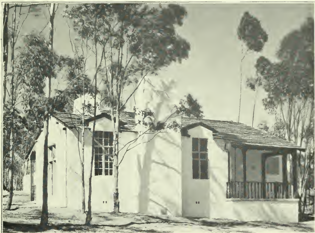
SOUTH FACADE, RESIDENCE OF MRS. CAROLINE JOHNSON, PALOS VERDES ESTATES
