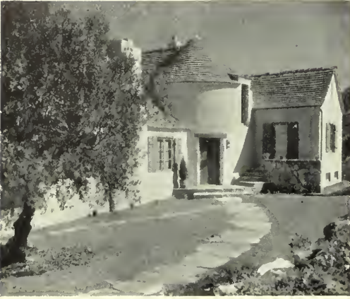
SOUTH FRONT, RESIDENCE OF GEO. C. KINCAID PALOS VERDES ESTATES
