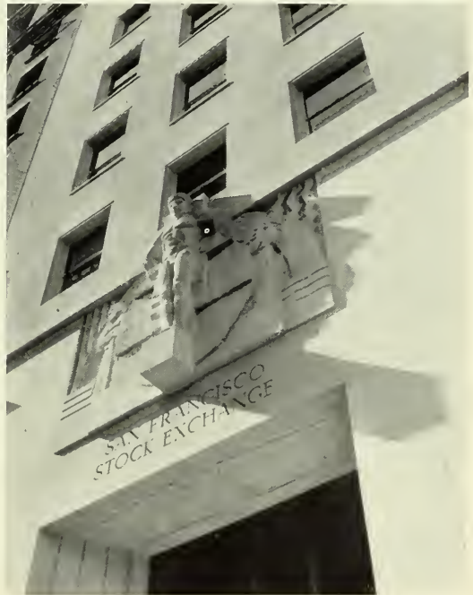
DETAIL, SANSOME STREET ENTRANCE, STOCK EXCHANGE, SAN FRANCISCO
