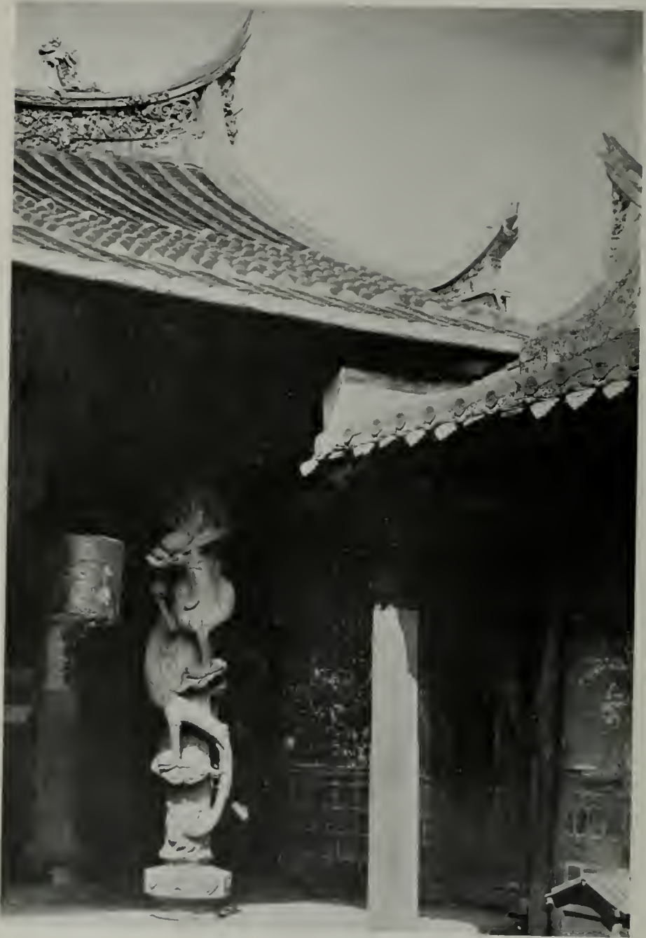
JUNCTION OF COLONNADE WITH ALTAR BUILDING, SHOWING ONE OF THE STONE DRAGON COLUMNS
