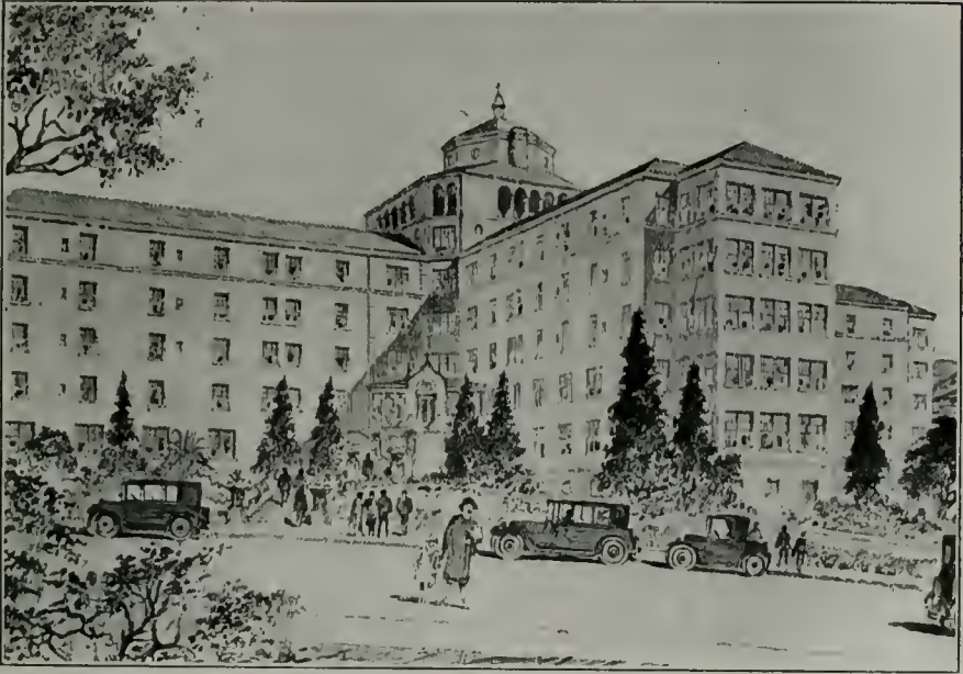
PROVIDENCE HOSPITAL, OAKLAND R. A. Herold, Architect, C. C. Cuff, Associate
