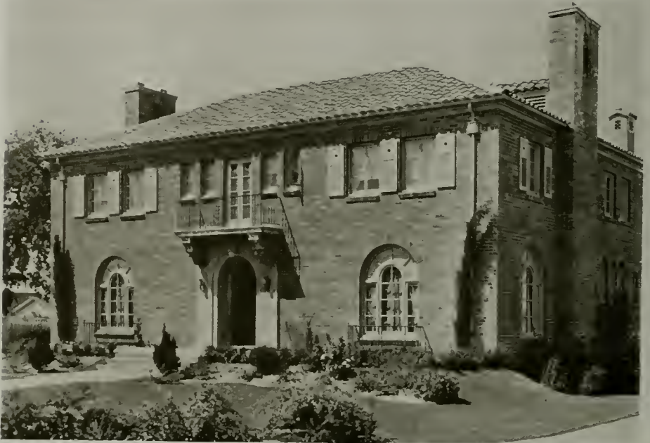
HOUSE OF MR. SIMON HORNSTEIN, SACRAMENTO A. R. Widdowson, Architect See Plan, Page 70
