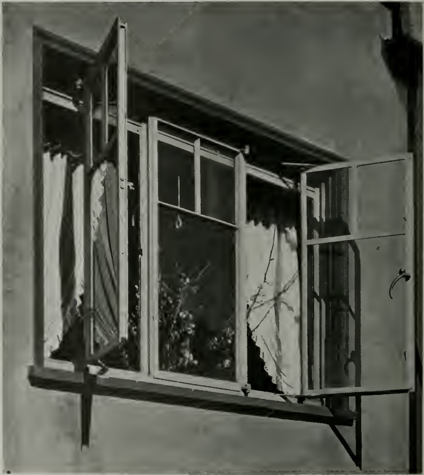
CLEANING SIMPLIFIED BY USE OF THE SLIDE HINGE IN BERKELEY HOME
