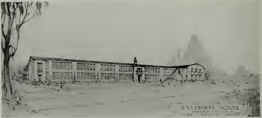
HAWTHORNE SCHOOL, OAKLAND
