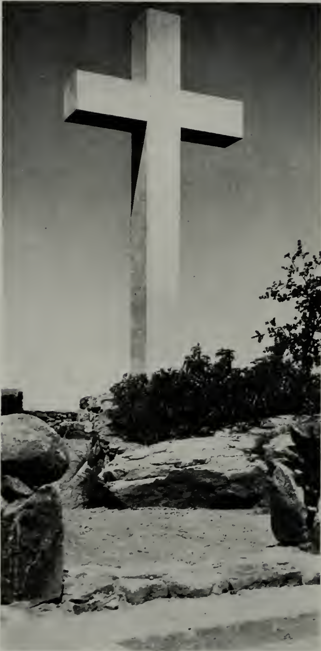
THE CROSS ON THE SUMMIT OF MT. HELIX, 1500 FEET ELEVATION, JUST ABOVE THE Mt. Helix Nature Theatre, near San Diego, California. This massive cross, entirely of reinforced concrete, is three feet square in section and stands 35 feet above the summit. A circular seat of natural stone gathered nearby entirely surrounds the cross which is lighted at night by means of six powerful flood lights.
