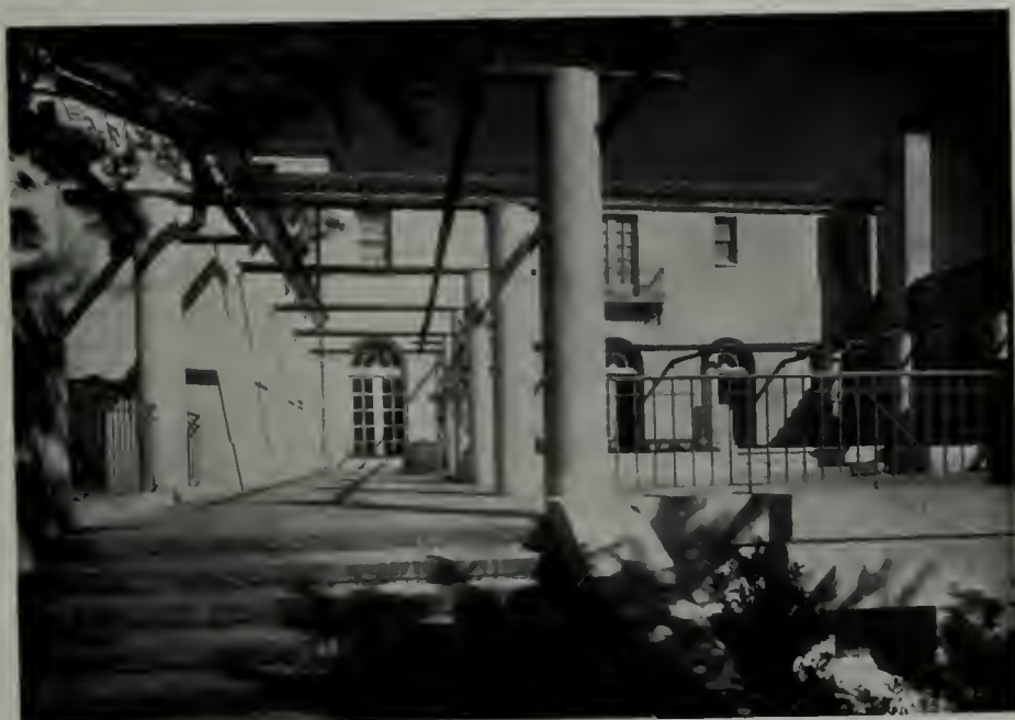
PERGOLA, OLYMPIC GOLF AND COUNTRY CLUB, SAN FRANCISCO Bakewell & Brown and Jno. A. Baur, Architects
