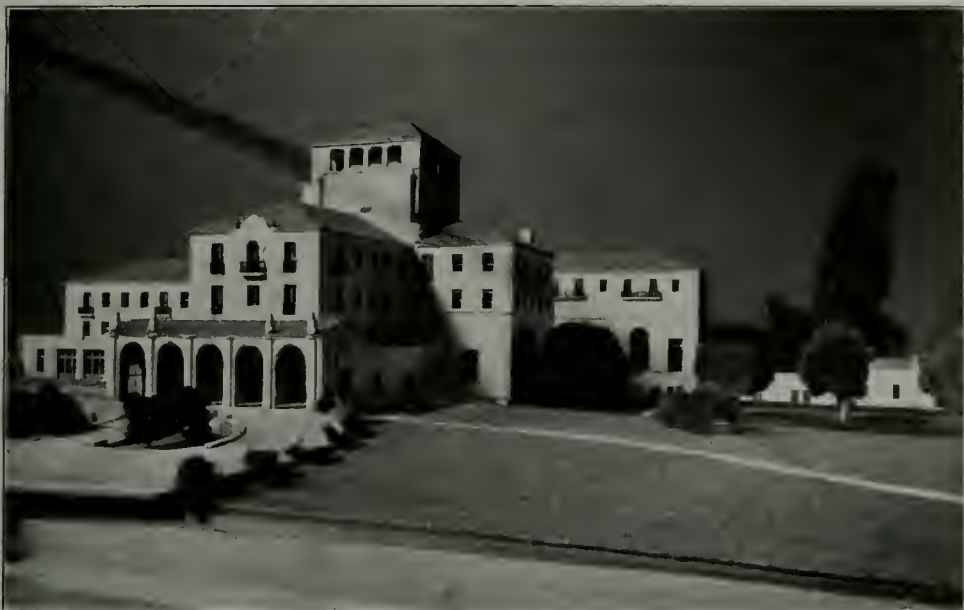
PHOTOGRAPH OF MODEL, NEW HOTEL DEL MONTE, MONTEREY Lewis P. Hobart and Clarence A. Tantau, Architects
