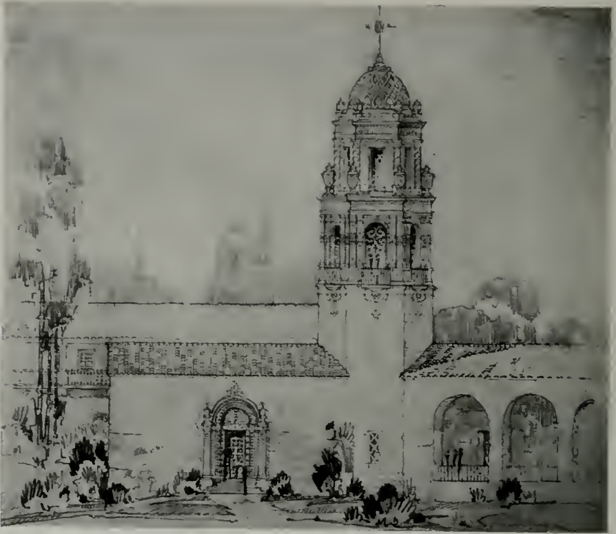
TOWER, FINE ARTS BUILDING, MILLS COLLEGE W. H. Ratcliff, Jr., Architect
