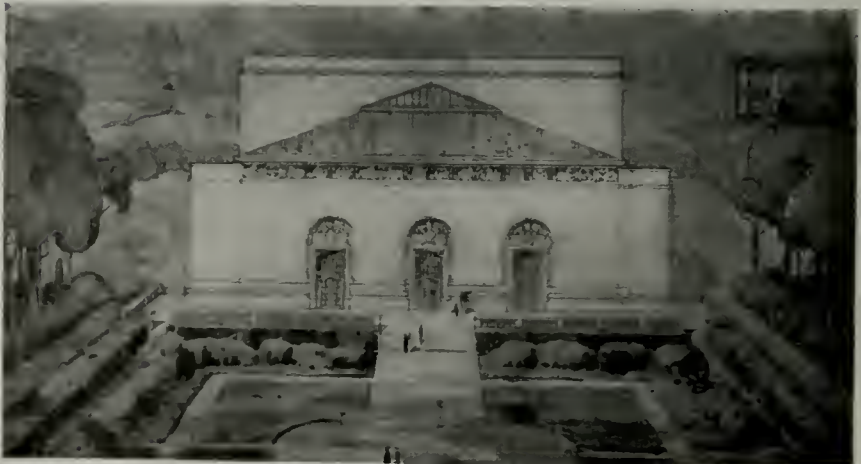
AUDITORIUM, MILLS COLLEGE W. H. Ratcliff, Jr., Architect
