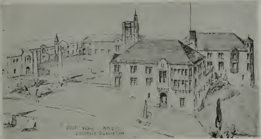
DORMITORY, PACIFIC SCHOOL OF RELIGION W. H. Ratcliff, Jr., Architect
