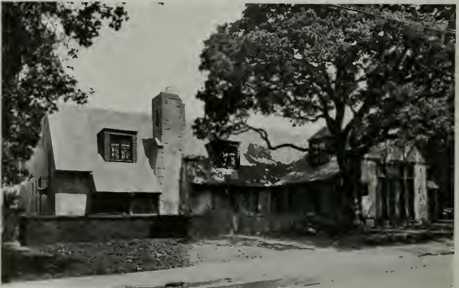
ROCKRIDGE WOMEN'S CLUB, OAKLAND Miller and Warnecke, Architects
