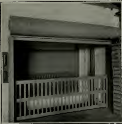
Safety Gate and Automatic Steel Rolling Door on Elevator Opening
