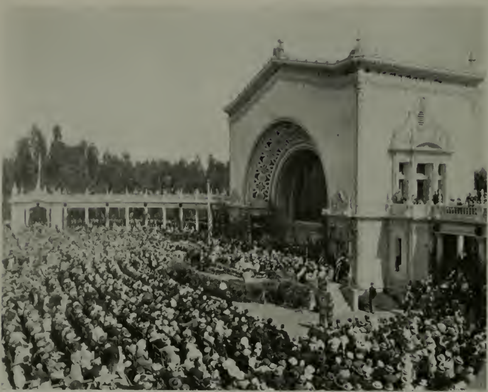
The Outdoor Organ in Balboa Park, San Diego. The only one of its kind existing. Built by John D. Spreckle's of San Diego and his brother Adolph, of San Francisco, for the Panama-California Exposition of 1915-16 and afterwards presented to the City of San Diego. Ever since maintained by these spirited citizens, free concerts being given daily throught the year. Serves the double purpose of an outdoor instrument and an open-air theatre. Used for community singing, celebrations and observances. The stage is large enough to accommodate 100 or more singers. Seating capacity 2500 with standing room adjacent for thousands more. Photograph, courtesy of San Diego-California Club.
