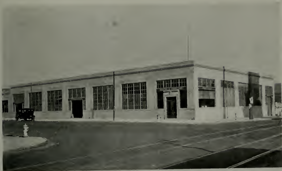
NEW BUILDING FOR JAS. A. NELSON, INC., SAN FRANCISCO
