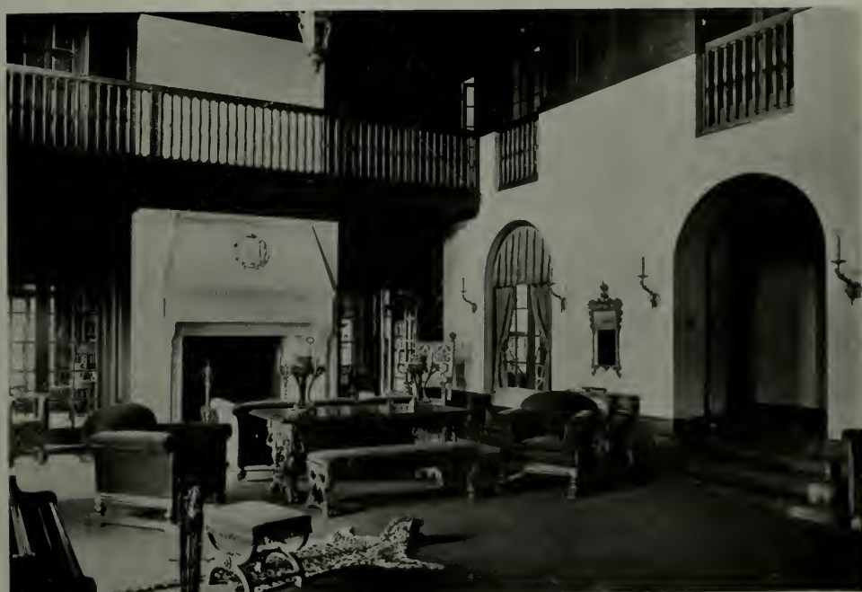
LIVING ROOM, HOUSE OF MRS. ROY CARUTHERS Morris H. Whitehouse, Architect
