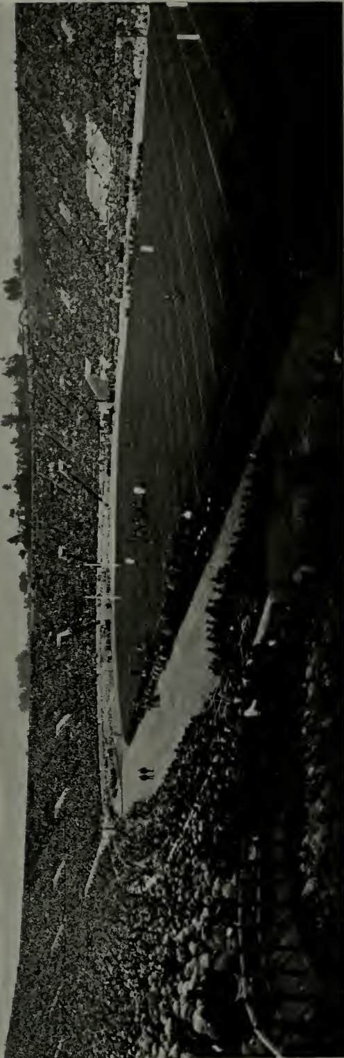
Tournament of Roses Stadium, Pasadena, California, Myron Hunt, Architect. Built 1922. Seating capacity 53,000. Can be enlarged to 75,000. Total width, 490 feet. Total length, 1000 feet. Acreage 15. Entrance to the Stadium is thru twenty tunnels running from ground level to half way up on the seats. Two large tunnels capable of handling autos run from ground level to playing field. The dressing rooms are alongside these larger tunnels. Photograph by Hiller, Pasadena. Photograph, courtesy of Chamber of Commerce and Civic Association, Pasadena.
