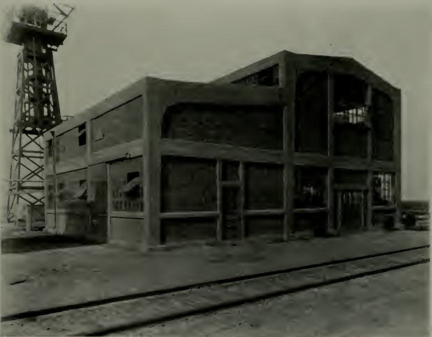
FIG. 4. SULPHUR DIOXIDE BUILDING, AVON, CALIFORNIA Villadsen Bros., Inc., Construction Engineers
