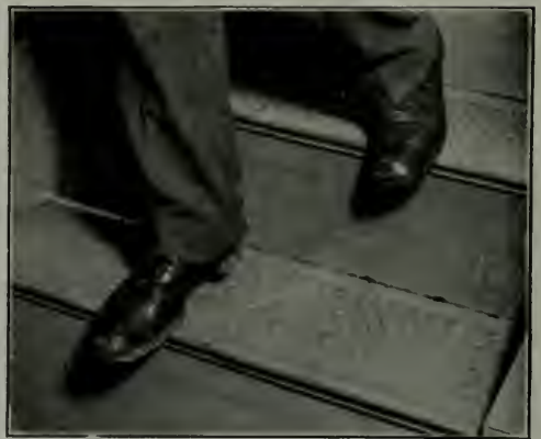
A person coming down steps usually carries his weight with the ball of the foot on the edge of the step which should be slip-proof for safety.
