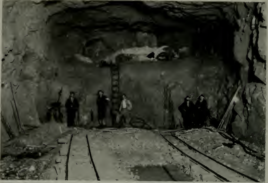
EXCAVATION ON TAILRACE TUNNEL, DON PEDRO DAM Photo taken August 5, 1922
