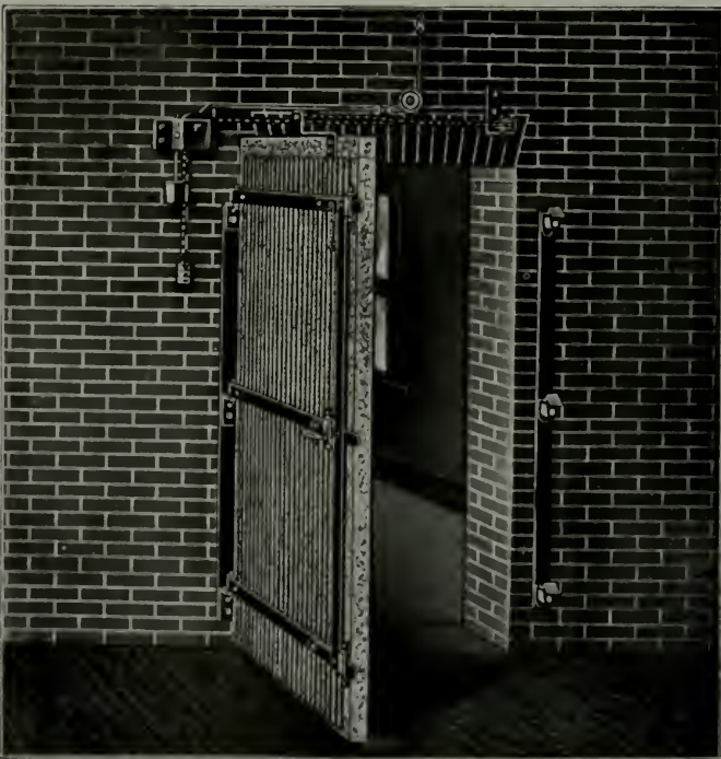
SWINGING TYPE FWER WALL AUTOMATICALLY CLOSING FIRE DOOR
