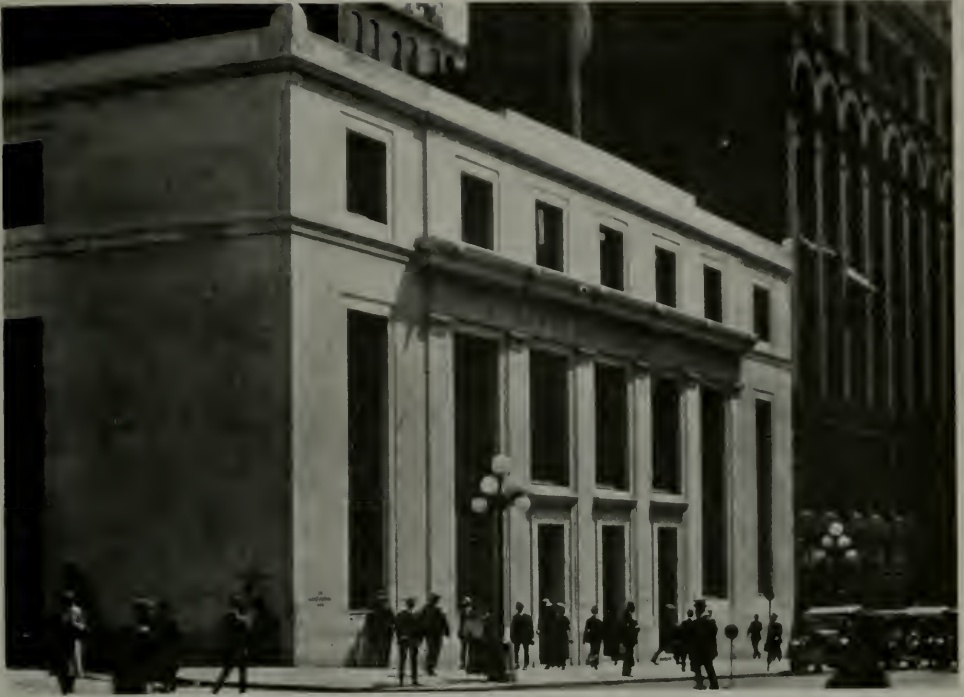
SEATTLE NATIONAL BANK. SEATTLE, WASHINGTON Doyle and Merriam, Architects
