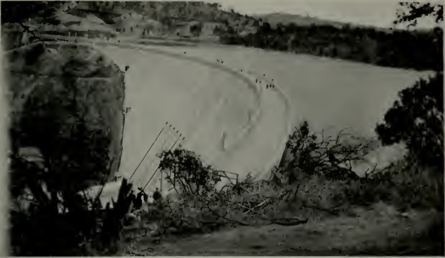
DON PEDRO DAM, NEAR LA GRANGE, CALIFORNIA
