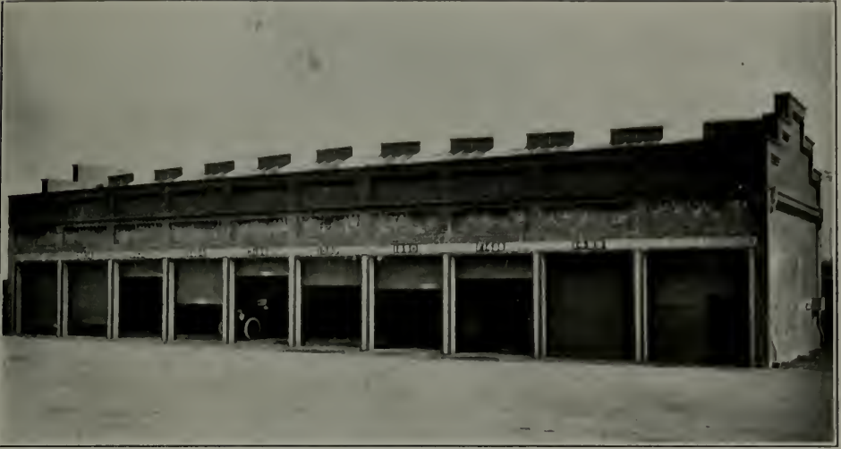
INDUSTRIAL OR CORPORATION GARAGE, SHOWING USE OF STEEL ROLLING DOORS FOR EACH TRUCK
