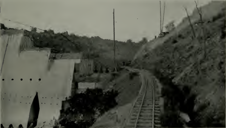
TEMPORARY RAILROAD FOR TRANSPORTING MATERIALS TO DAM SITE
