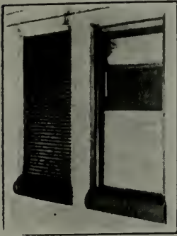
TYPICAL INSTALLATION OF UNDERWRITERS LABELLED FIRE SHUTTERS, PROTECTING WINDOW OPENINGS.
