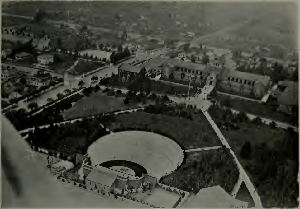
Memorial Open Air Theatre, High School group, Santa Monica, California. Allison & Allison, Architects. Built in 1921. Seats 3000. Construction of concrete and brick. Enriched with a pool before the stage. Airplane view. Photograph loaned thru courtesy of Allison and Allison.
