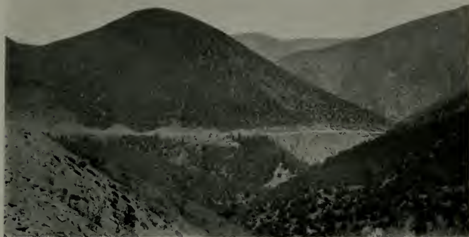
COMPLETED PORTION OF YOSEMITE VALLEY ROAD FROM THE SUMMIT TO BRICEBURG
