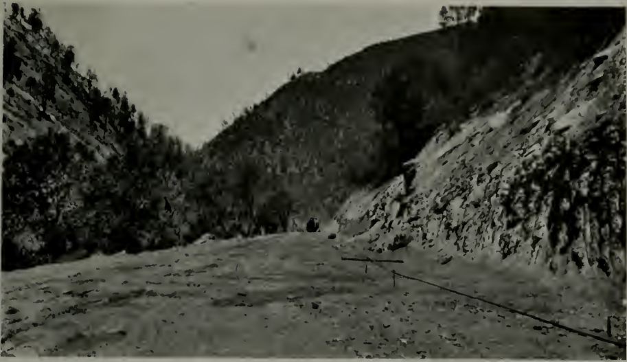
COMPLETED PORTION OF YOSEMITE VALLEY ROAD
