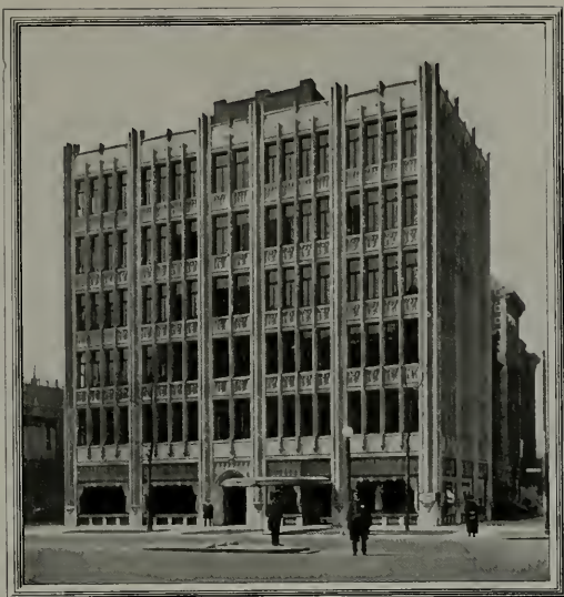
Building at Michigan and Chicago Avenues, Chicago—Entire Facing of Cast Stone Robert T. Newberry, Chicago, Ill., Architect. Ridenour & Erickson, Chicago, Contractor
