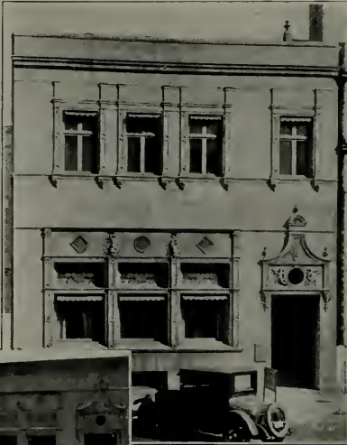
Milwaukee Art Institute Building. Remodeled in 1921. Juddell & Bogner, Architects.
