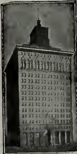
MATSON BUILDING San Francisco, Cal. Bliss and Faville, Archt's
