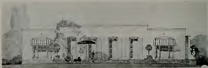
HOUSE AT PEBBLE BEACH Lewis P. Hobart, Architect
