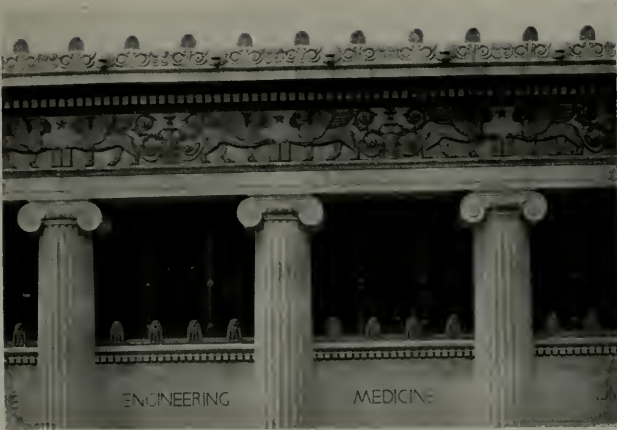
Detail of Entablature, Wilmington Public Library, Wilmington, Delaware. E. L. Tilton and A. M. Githens, Architects. Frieze and cornice in polychrome Terra Cotta. (Colors, deep yellow buff, gray and blue. Cornice repeats limestone coloring.)
