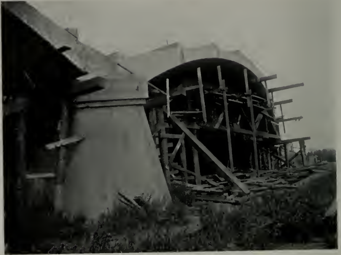
FIG. 2—VIEW TAKEN UNDER CURVED ARCH, BRIDGE AT SCHENECTADY, NEW YORK
