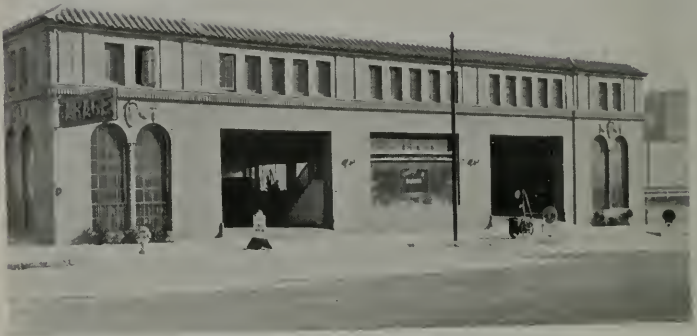
GARAGE FOR MR. FRANK CLARK, SAN FRANCISCO Baumann and Jose, Architect and Engineer
