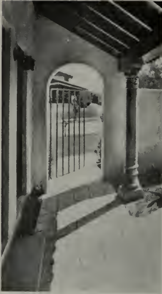
Detail of Entrance Porch, House at 149 St. Andrews Place, Los Angeles. Ernest Irving Freese, Architect
