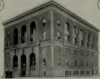
FRESNO BEE BUILDING, FRESNO, CAL.
