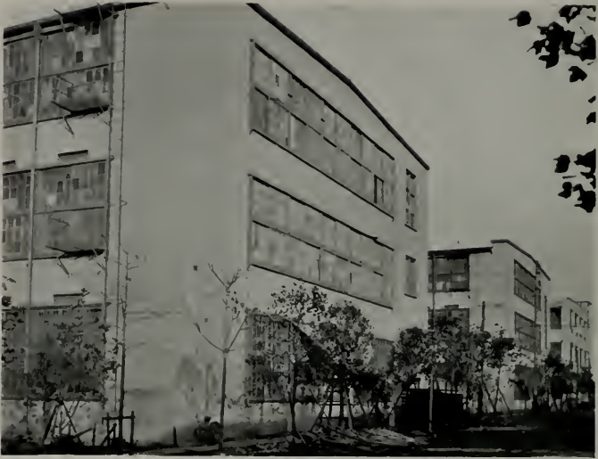
LAMP FACTORY BUILDING, KAWASAKI, OF WOOD CONSTRUCTION. UNDAMAGED.
