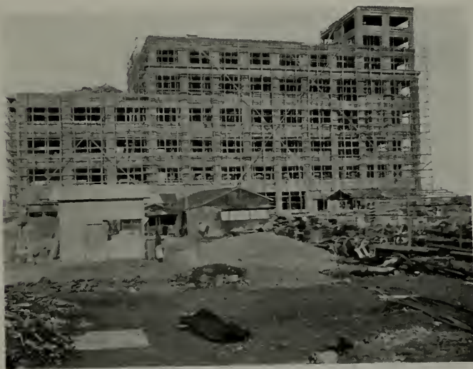
REINFORCED CONCRETE FLOUR MILL UNDER CONSTRUCTION. First story columns slightly damaged.
