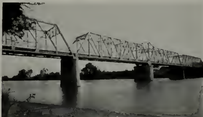
Woodson Bridge over Sacramento River, near Corning, Cal.
