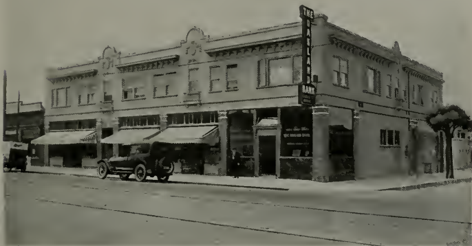
STORES AND APARTMENTS FOR MURPHY HAMILTON, OAKLAND Designed by Hutchison and Mills
