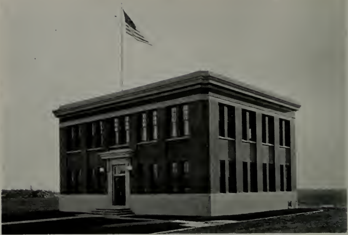
RADIO BROADCASTING STATION, OAKLAND
