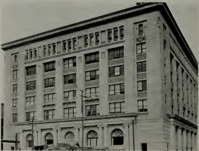
INDUSTRIAL BANK OF JAPAN, TOKYO Structural steel frame and reinforced concrete wall construction. Undamaged.
