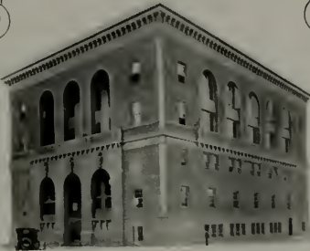
FRESNO BEE BUILDING, FRESNO, CAL.
