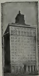
MATSON BUILDING San Francisco, Cal. Bliss and Faville, Archt's
