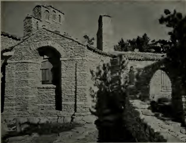
HOUSE OF MR. D. L. JAMES, CARMEL HIGHLANDS, CALIFORNIA C. Sumner Greene, Architect
