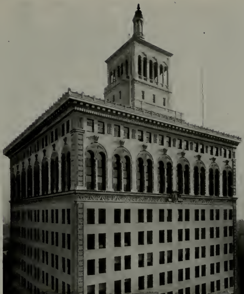
Upper stories of Matson Building, San Francisco, California. Bliss & Faville, Architects. Entirely finished in warm gray matt glazed Terra Cotta with background of ornamental features in blue green.
