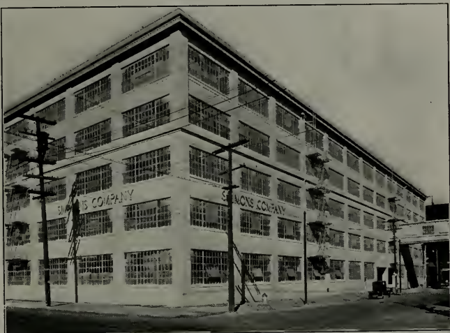
MANUFACTURING BUILDING — SIMMONS CO., SAN FRANCISCO, CALIF.
