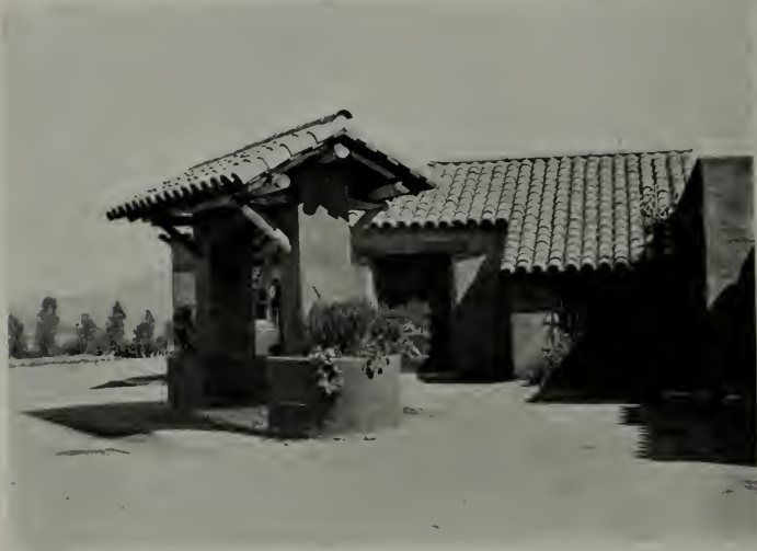
GASOLINE FILLING STATION, RANCHO SANTA FE Requa and Jackson, Architects
