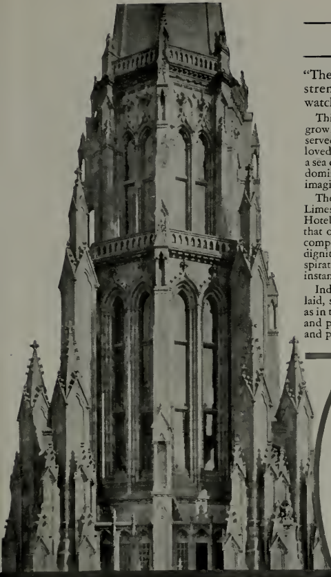
Temple Building Tower, Chicago, Holabird & Roche, Architects.
