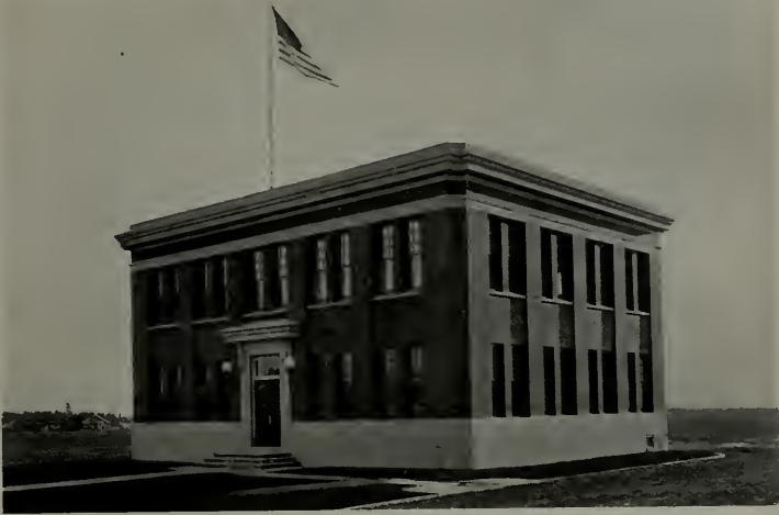
RADIO BROADCASTING STATION, OAKLAND
