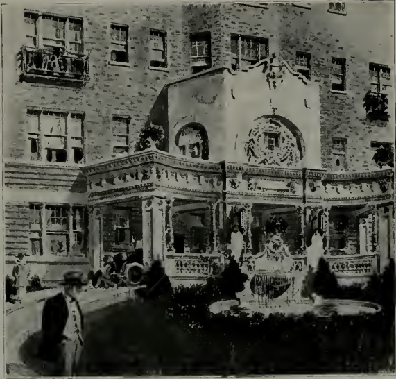
ENTRANCE, APARTMENT HOTEL, WASHINGTON, D. C. Sonneman & Justment, Architects F. W. Fitzpatrick, Consulting Architect
