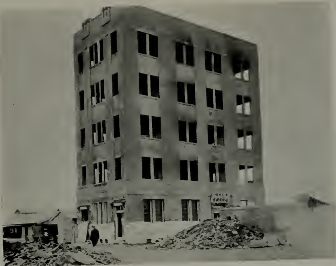
SMALL BURNED OUT, REINFORCED CONCRETE BUILDING, TOKYO. UNDAMAGED.
