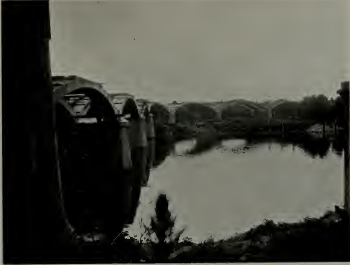
FIG. 1—CURVED ARCH BRIDGE, NEAR SCHENECTADY, NEW YORK Structure is 4436 feet long and will cost $3,000,000
