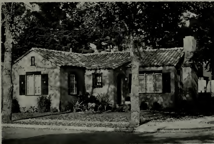
Residence of Ernest Ingold, 1100 Balboa Avenue, Burlingame, California. H. C. Bauman, Architect
