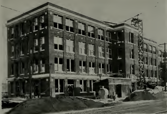
PROGRESS PICTURES, BUILDING FOR THE AMERICAN CAN CO., SAN FRANCISCO Lindgren & Swinnerton, Inc., Builders
