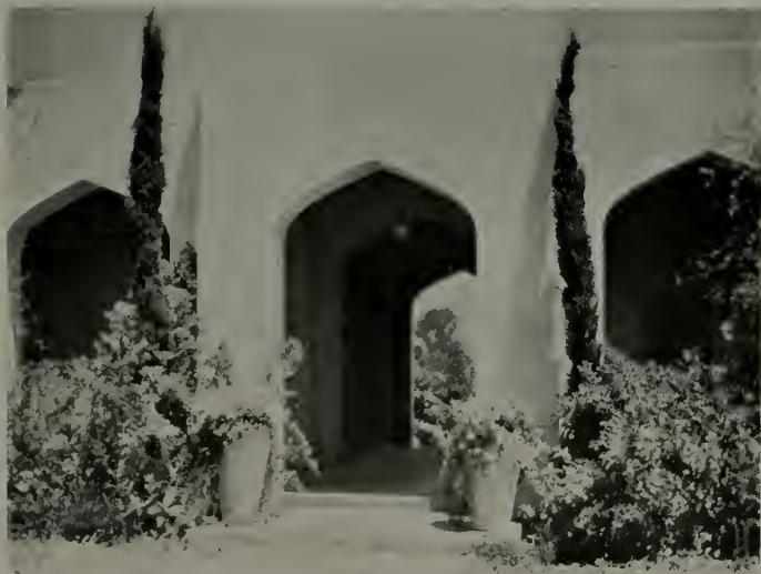
DETAIL OF CLOISTERS, SAMARKAND HOTEL, SANTA BARBARA Geo. A. Dennison and Chas. F. Ingerson, Designers
