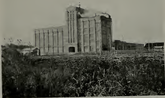
CASCADE BREWERY, TSURUMI, OF REINFORCED CONCRETE. UNDATED.
