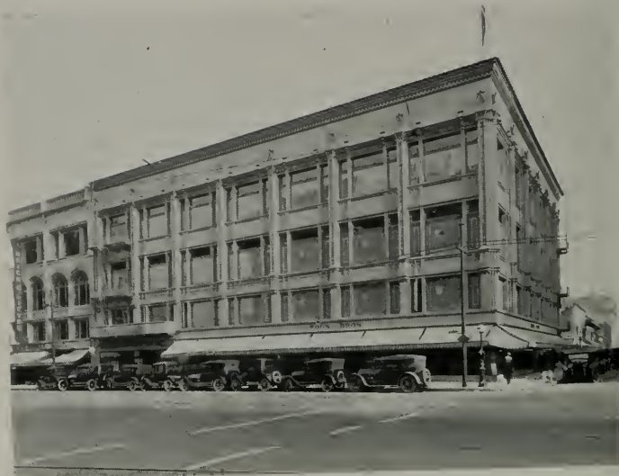
STORE BUILDING FOR ROOS BROS., OAKLAND Broadway Realty Company, Owners William Knowles, Architect and Contractor
