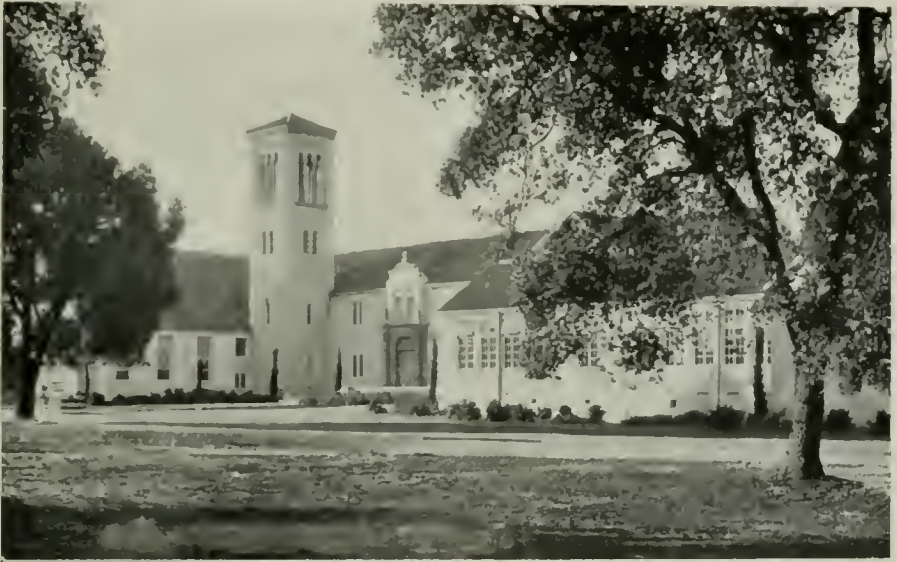
PALO ALTO UNION HIGH SCHOOL BUILDING
