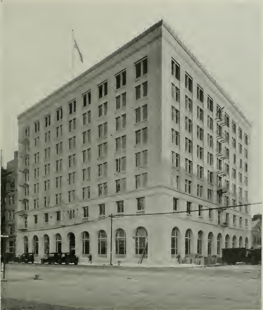
BUILDING FOR WALTON N. MOORE DRY GOODS COMPANY, SAN FRANCISCO Geo. W. Kelham, Architect Foundation Company, Builders
