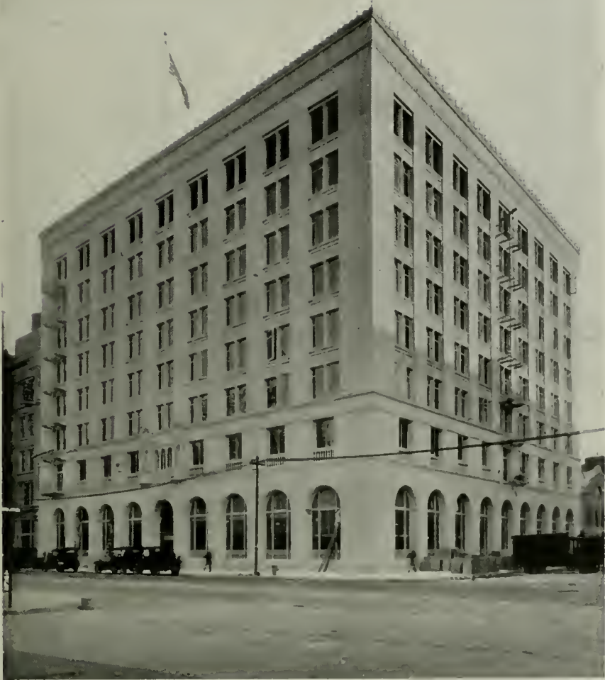
BUILDING FOR WALTON N. MOORE DRY GOODS COMPANY, SAN FRANCISCO Geo. W. Kelham, Architect Foundation Company, Builders
