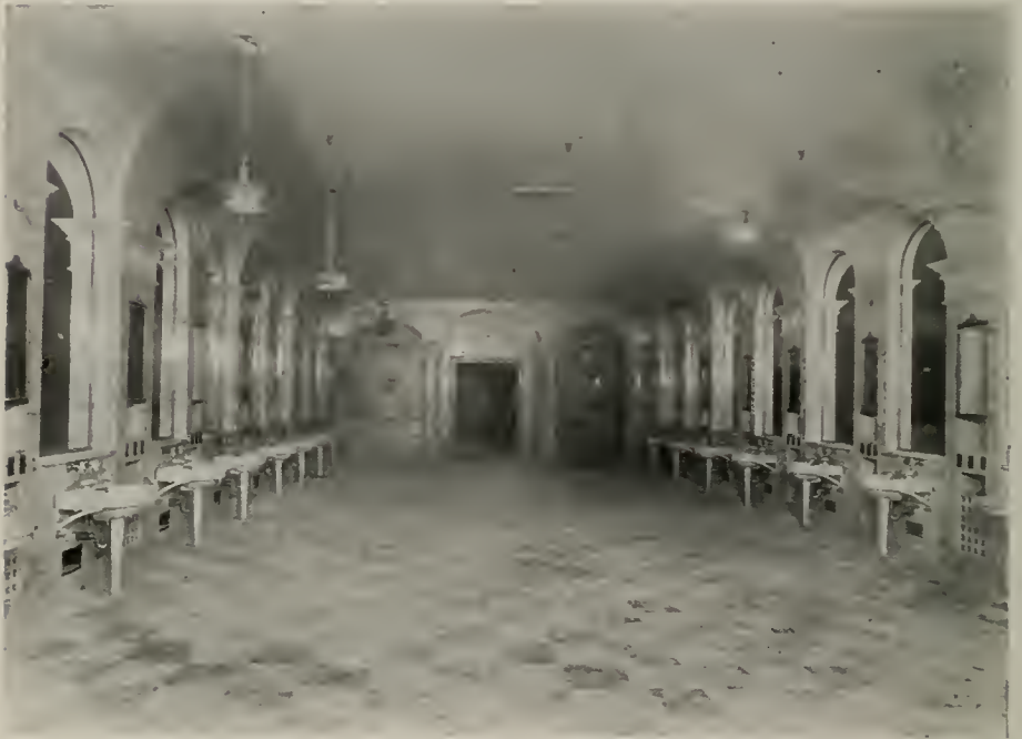
THE NEW BILTMORE HOTEL, LOS ANGELES, IS EQUIPPED THROUGHOUT WITH PACIFIC SANITARY MANUFACTURING COMPANY'S FIXTURES
