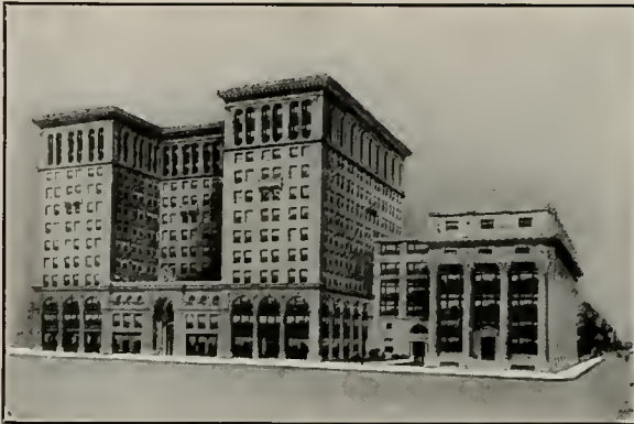
Pacific Mutual Life Insurance Building, Los Angeles, Cal. Wm. J. Dodd and Frank Richards, Architects
