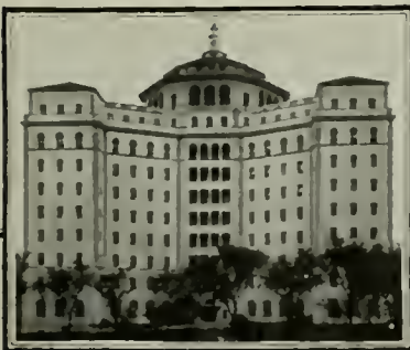
The largest single stucco job in the world, the Fifth Avenue Hospital of New York, for permanence as well as beauty chose Atlas White.
