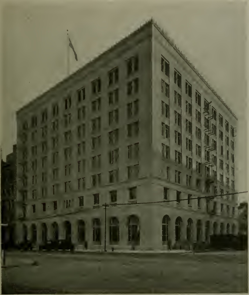
BUILDING FOR WALTON N. MOORE DRY GOODS COMPANY, SAN FRANCISCO Geo. W. Kelham, Architect Foundation Company, Builders
