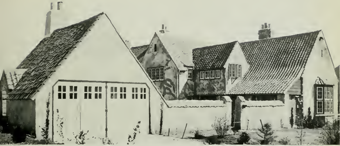
P. T. BURTIS RESIDENCE. SACRAMENTO, CALIF. Dean & Dean, Architects
