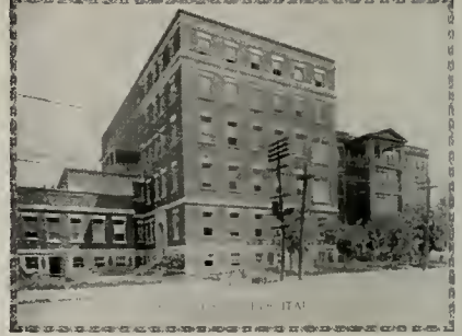
Joseph Sawyer, Montreal, Architect Century Electric Co., Montreal, Electrical Contractors
