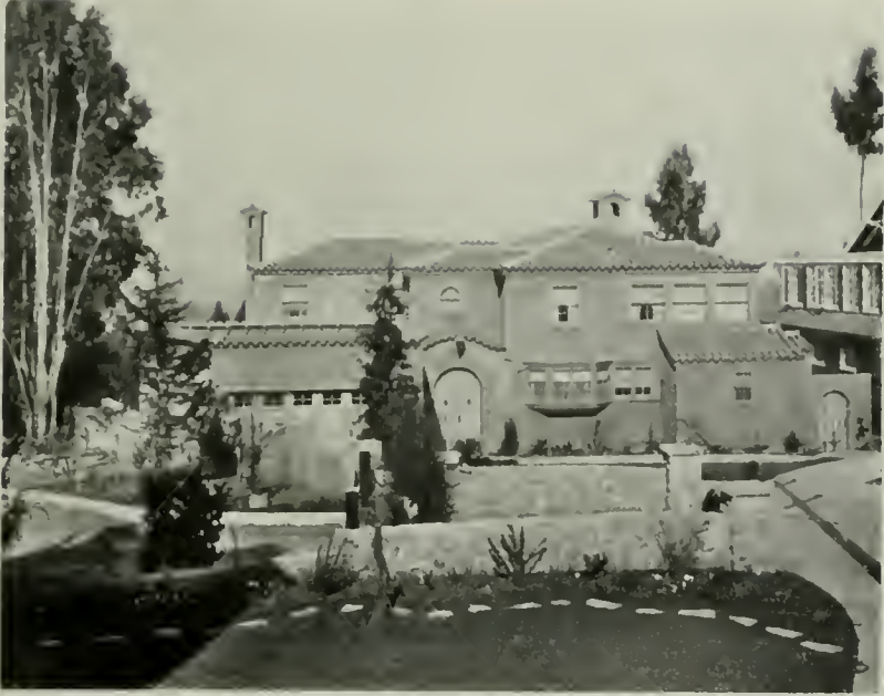
HOUSE OF MR. E. J. SCHNEIDER, CLAREMONT Albert Farr, Architect and J. F. Ward, Associate Horace George Cotton, Landscape Architect
