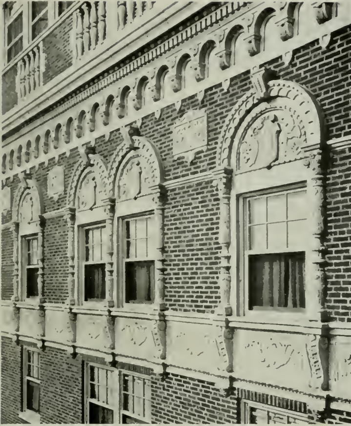
Detail of Terra Cotta, Upper Stories, Chase Hotel, St. Louis, Mo. Preston J. Bradshaw, Architect
