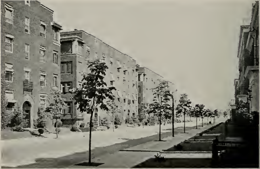
STREET VIEW, JACKSON HEIGHTS APARTMENTS Andrew J. Thomas, Architect
