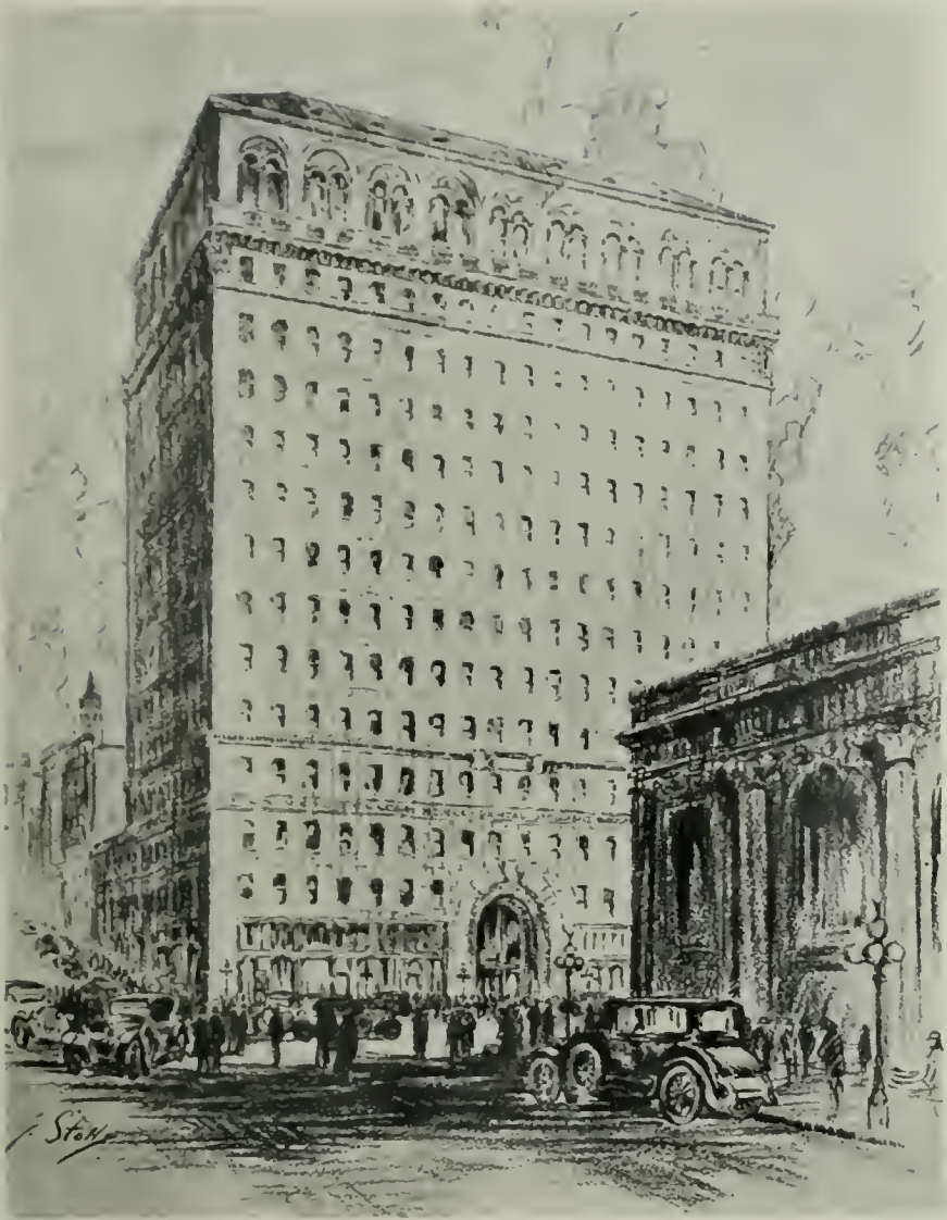
PHYSICIANS' BUILDING, SAN FRANCISCO Geo. W. Kelham, Architect
