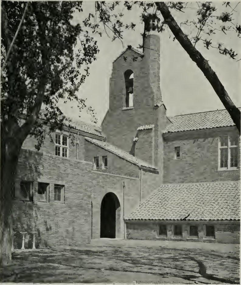
DETAIL OF TOWER, FREMONT SCHOOL, 24th and N Sts., Sacramento Hemmings, Petersen, Hudnutt, Architects; Dean & Dean, Designers and Successors K. E. Parker Co., General Contractors; White & Gloor, Masonry Contractors
