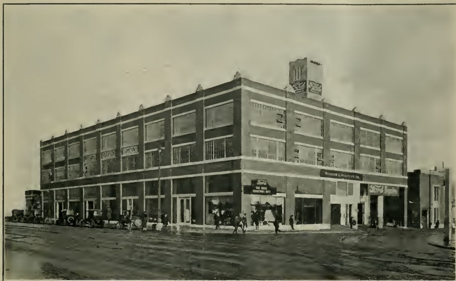
WM. L. HUGHSON BUILDING Market at Eleventh San Francisco W. L. SCHMOLLE, Architect
