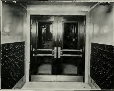
SECURITY BANK, ST. LOUIS, MO. (Entrance Vestibule)
