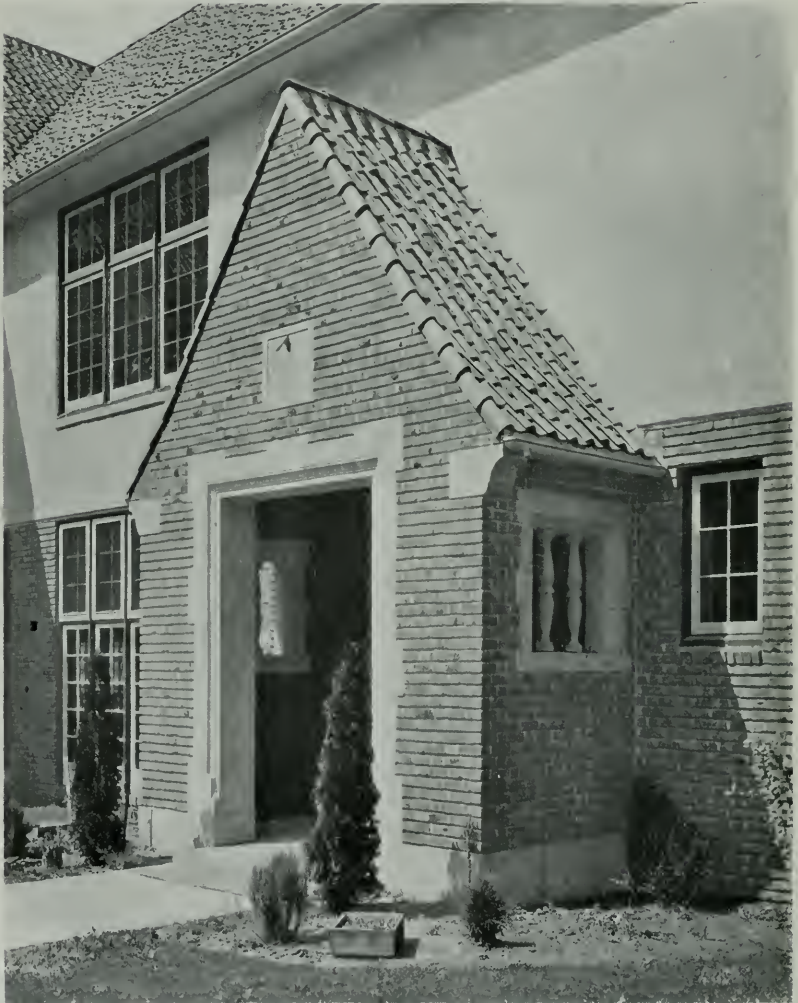
ENTRANCE DETAIL, JEFFERSON SCHOOL, SACRAMENTO Hemmings, Petersen, Hudnutt, Inc., Architectural and Engineering Commission Dean & Dean, Architects, Designers and Successors
