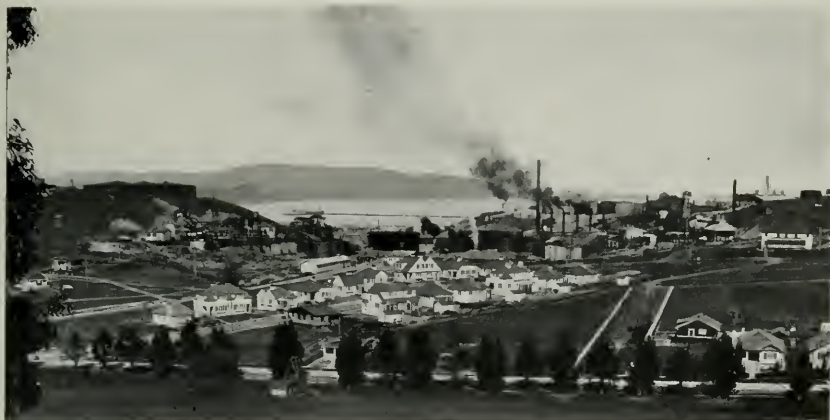
AEROPLANE VIEW OF SHELL OIL COMPANY'S EMPLOYEES' COTTAGES AT MARTINEZ, CONTRA COSTA COUNTY
