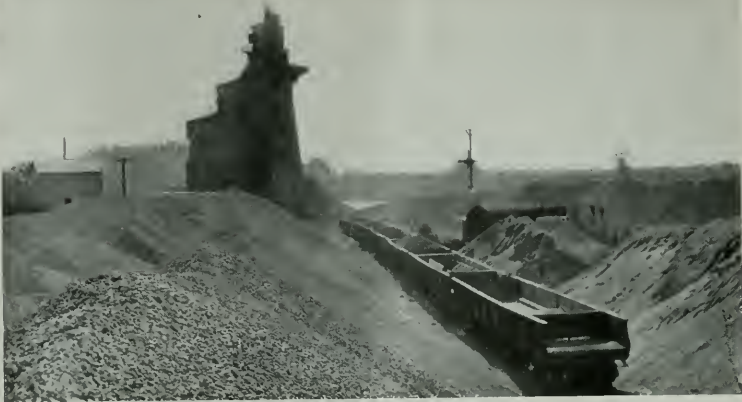
VIEW AT NILES PLANT
