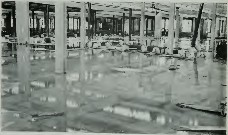
CONCRETE FACTORY FLOOR PROTECTED WHILE HARDENING BY "PONDING" A Method Often Used in Concrete Road Construction
