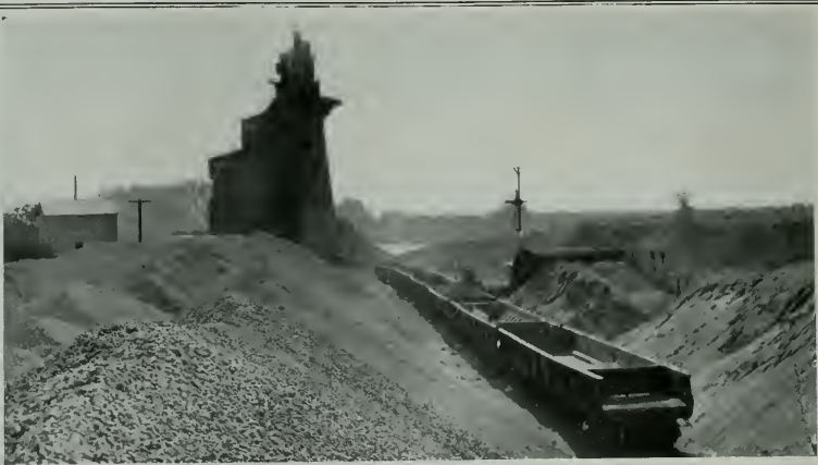
VIEW AT NILES PLANT
