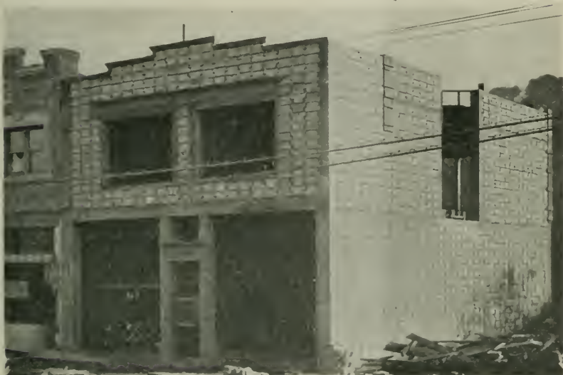
STORE AND APARTMENT BUILDING, SAN ANSELMO, CAL. (Sawyer System Pre-cast Unit Concrete Construction)
