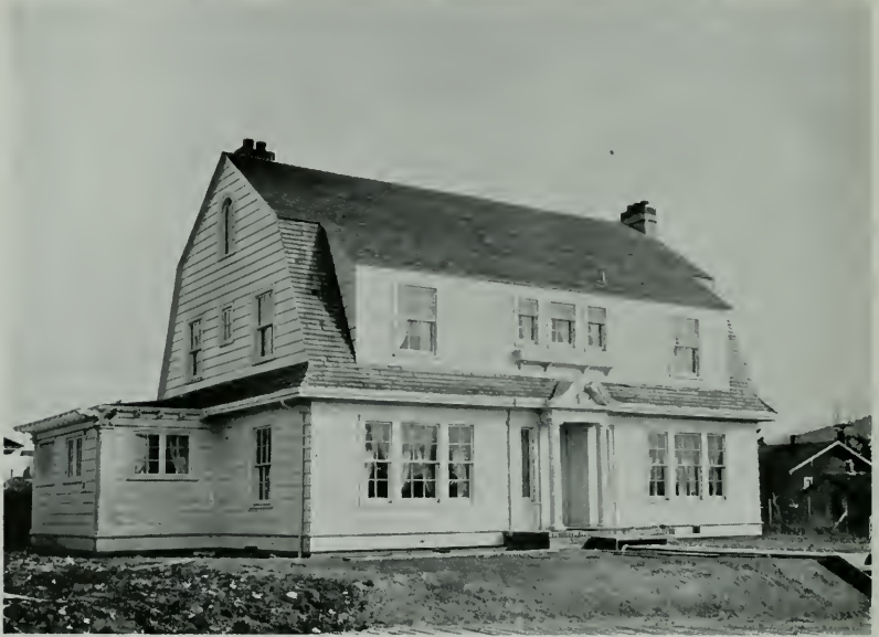
HOUSE OF MR. O. W. FISHER, JR., SEATTLE J. Lister Holmes, Architect
