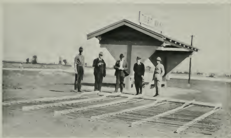
SPECIAL DEVICE FOR PLACING REINFORCING STEEL.
