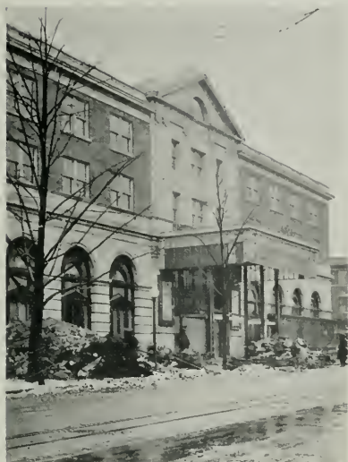
MAIN ENTRANCE, KNICKERBOCKER THEATER ON 18TH ST., N.W., WASHINGTON, D. C.
