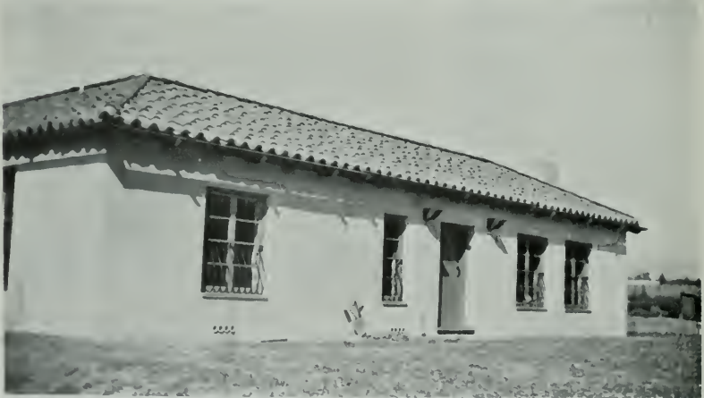
ADOBE HOUSE FOR MR. H. A. GORHAM, SANTA MONICA, CAL. John Byers, Designer and Builder
