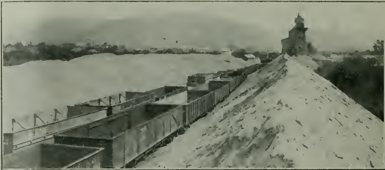
STORAGE FACILITIES AT NILES PLANT
