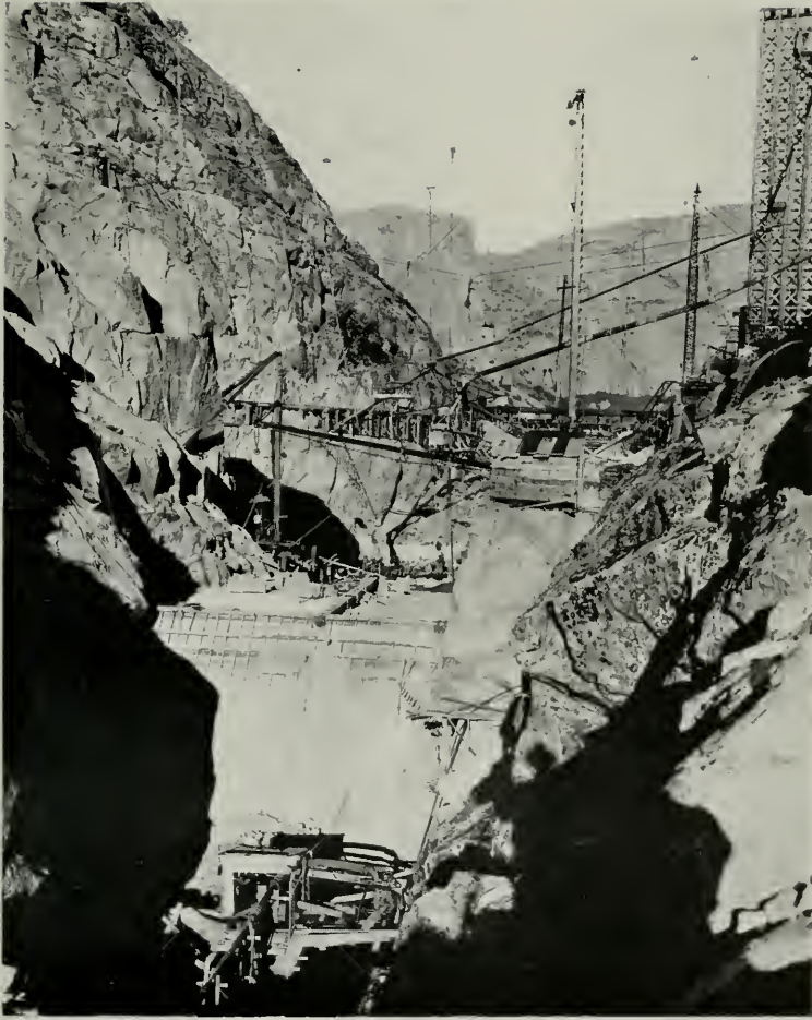
POURING CONCRETE IN HETCH-HETCHY DAM, NOVEMBER, 1921
