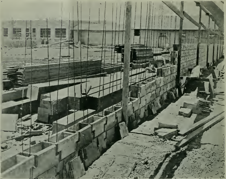
WALLS OF WINTER GARDEN, MODESTO, SHOWING METHOD OF CONSTRUCTION, SAWYER SYSTEM
