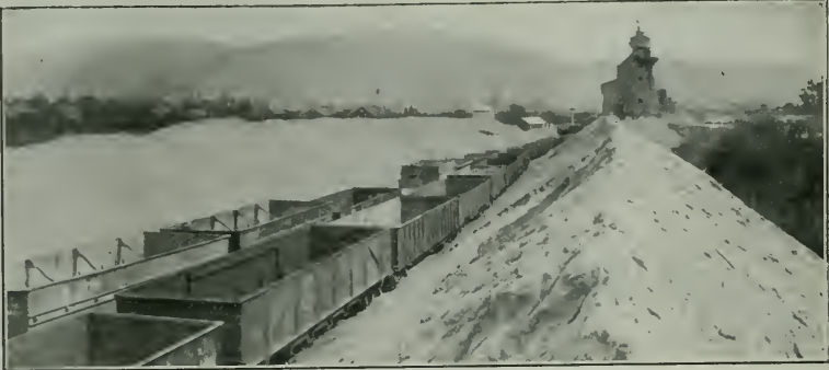
STORAGE FACILITIES AT NILES PLANT
