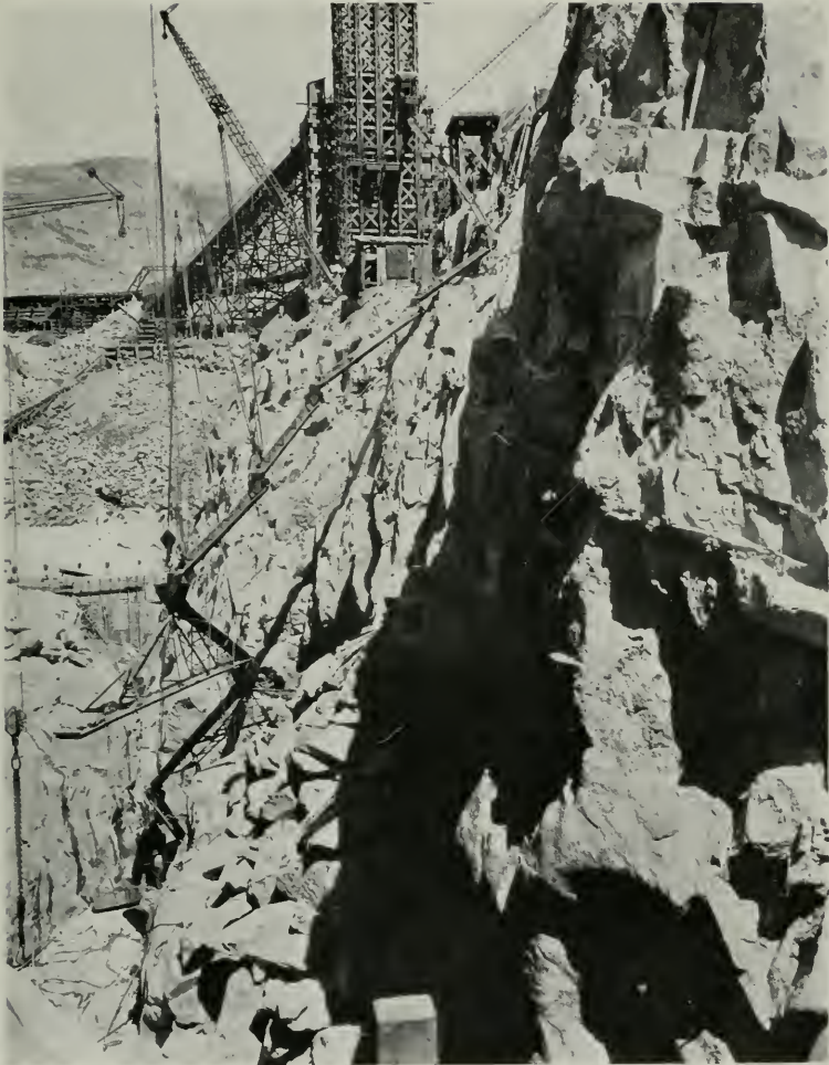
GENERAL VIEW OF SOUTH SIDE AND BOTTOM OF DAM SITE
