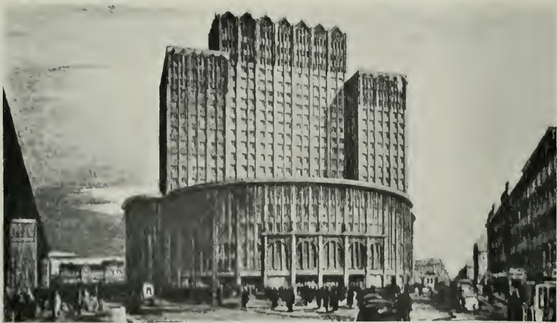
UNIQUE OFFICE BUILDING BEING ERRECTED IN BERLIN Courtesy Leslie's Weekly
