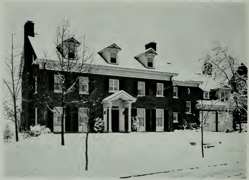
HOUSE OF MR. WILLIAM PIGOTT, SEATTLE Joseph S. Cote, Architect
