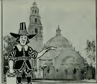
California State Bldg., San Diego, Calif.
