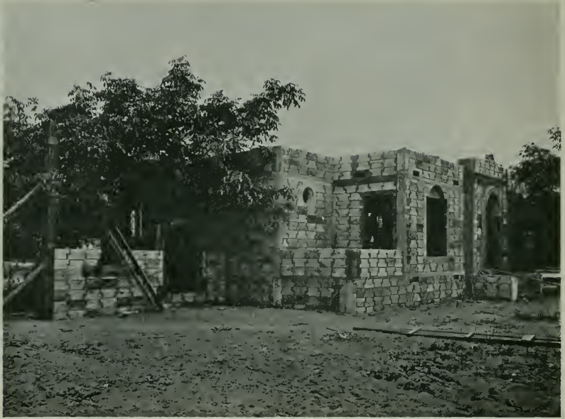
BUNGALOW BUILT IN SOUTHERN CALIFORNIA ACCORDING TO THE SAWYER SYSTEM
