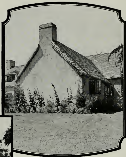
"Little Orchard Farm," residence of Mr. Samuel Heller, White Plains, N. Y., Mr. Frank J. Forster, New York, Architect.
