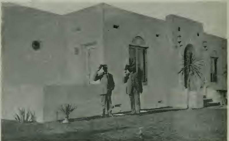
THE SAME BUNGALOW AFTER APPLICATION OF EXTERIOR CEMENT FINISH
