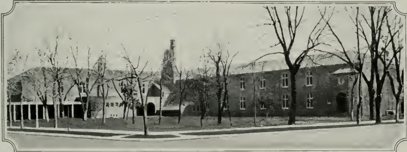
Jefferson School, Sacramento, California. James Dean, Architect Hemmings-Hudnutt & Petersen, Architectural Com. K. E. Parker, Contractor
