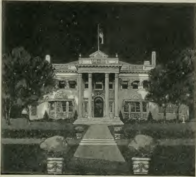
Residence of Mr. George E. Nicholson, Kansas City, Missouri. The walls are of 12-inch interlocking tile, and the stucco, made with Medusa Stainless White Cement and aggregates, is applied directly on the tile. It has a light body, finished with a dash coat of white quartz pebbles. Messrs. Wight & Wight, Kansas City, Architects.
