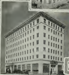
CITIZENS SAVINGS BLDG. PASADENA, CAL.
