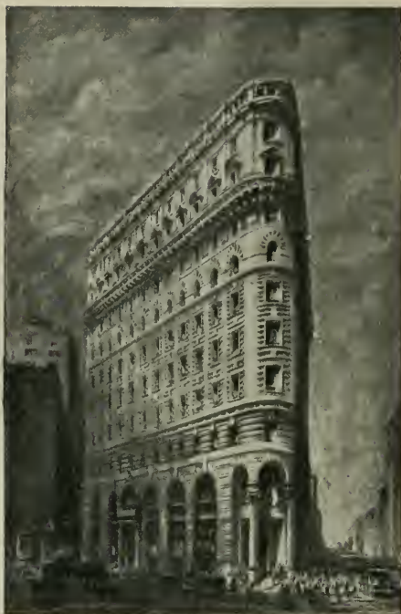
Copyright, 1922, by National Terra Cotta Society Drawing by Hugh Ferriss CROCKER BUILDING SAN FRANCISCO, CAL.
