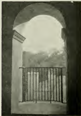
FROM THE BELVEDERE, LOOKING SOUTH OVER THE ROOF
