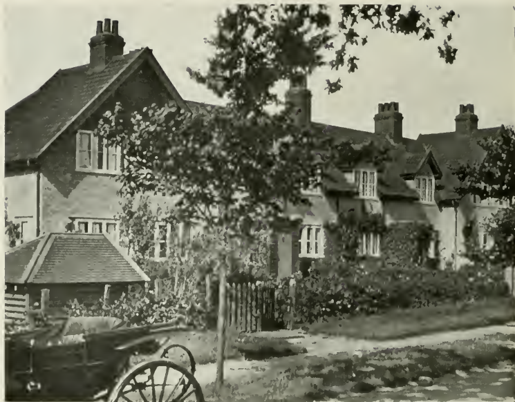
TYPICAL GROUP OF WORKERS' HOMES, BUILT FOUR TOGETHER, IN AN ENGLISH GARDEN CITY
