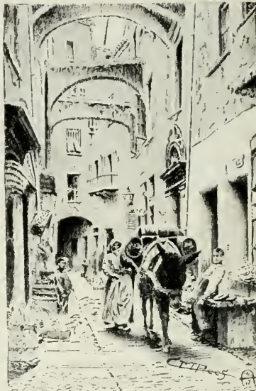
CONCRETE WALLS AND THE ARCHES BUILT IN 19 TH CENTURY
