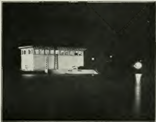
THE HALSEY POWER HOUSE
