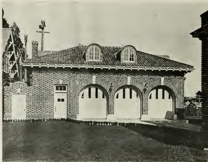
GARAGE, RESIDENCE OF MR. JUDSON C. RIVES, LOS ANGELES Alfred F. Rosenheim, Architect
