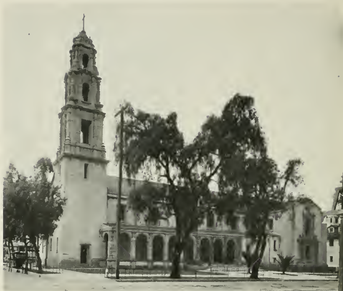
FIRST CONGREGATIONAL CHURCH, RIVERSIDE
