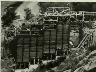
Part of an #1 & #6 Rock and Gravel Plant
