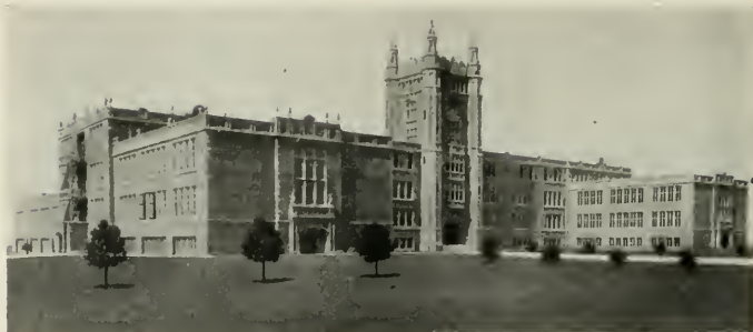
LOS ANGELES HIGH SCHOOL BUILDING
