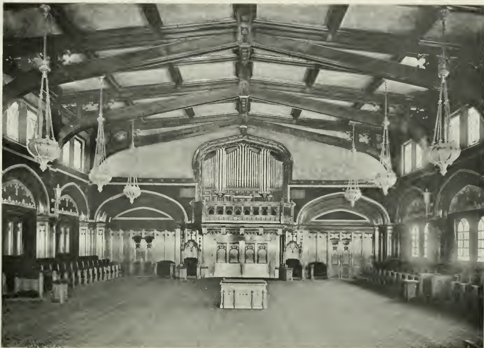
LODGE ROOM, BUILDING FOR SCOTTISH RITE BODIES, SAN FRANCISCO O'BRIEN & WERNER, ARCHITECTS
