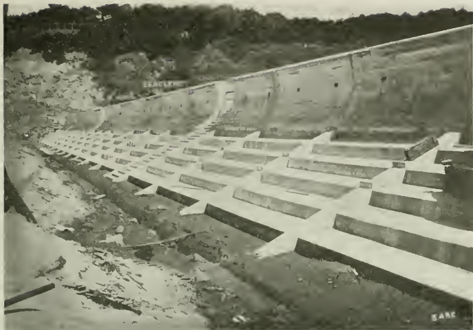
COMPLETED SECTION OF OCEAN BEACH ESPLANADE, SAN FRANCISCO M. M. O'Shaughnessy, City Engineer
