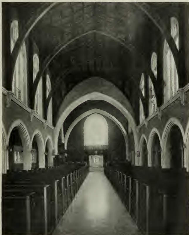
ST. PAUL'S EPISCOPAL CHURCH, OAKLAND, CALIFORNIA A good example of pressed brick work for interior finish BENJ. G. McDOUGALL, ARCHITECT
