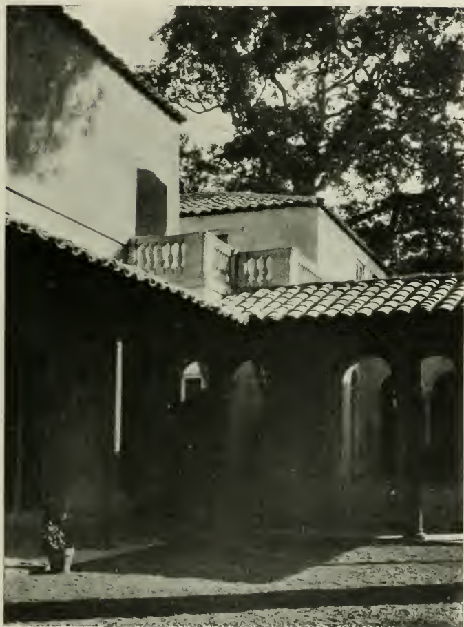
ANOTHER VIEW OF EXTERIOR TO PLAY ROOM FOR NEIGHBORHOOD CHILDREN, VILLA OF MR. CHARLES D. BLANEY, SARATOGA, CALIFORNIA. WILLIS POLK & CO., ARCHITECTS
