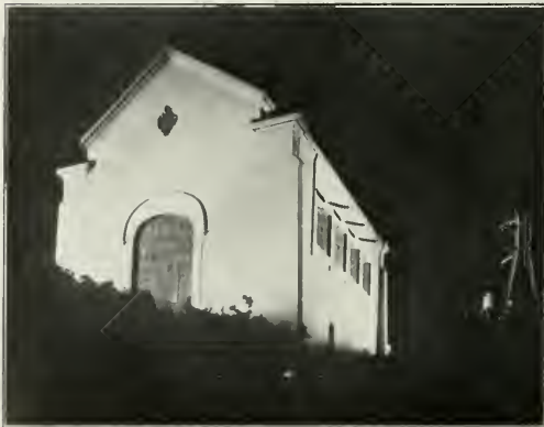
NIGHT VIEW, THE MARIN COUNTY SUBSTATION
