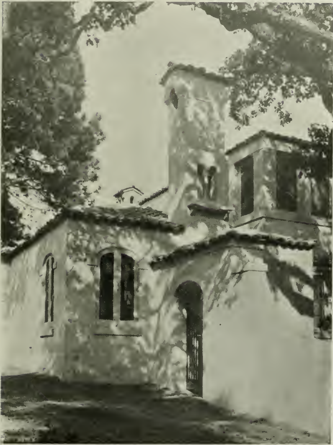
GATEWAY FROM WEST GARDEN TO KITCHEN YARD, VILLA OF MR. CHARLES D. BLANEY, SARATOGA, CALIFORNIA. WILLIS POLK & CO., ARCHITECTS
