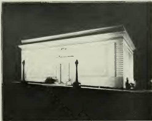
A CITY SUBSTATION
