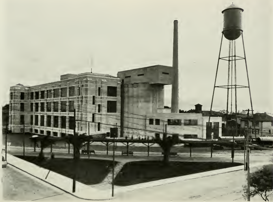
A FACTORY WITH THE MAXIMUM OF LIGHT AND AIR. PLANT OF PACIFIC COAST SHREDDED WHEAT CO., OAKLAND L. P. Hobart and Chas. H. Cheney, Associate Architects H. J. Brunner, C. E.
