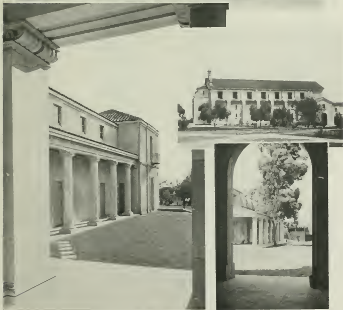
MAIN FACADE AND ELEVATION, MUSIC BUILDING, POMONA COLLEGE VIEW THROUGH DOORWAY SHOWS PORCH OF ART BUILDING
