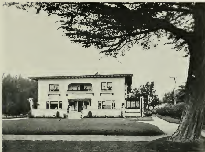
HOUSE FOR MR. F. H. DAVIS, SANTA CRUZ Chester H. Miller, Architect
