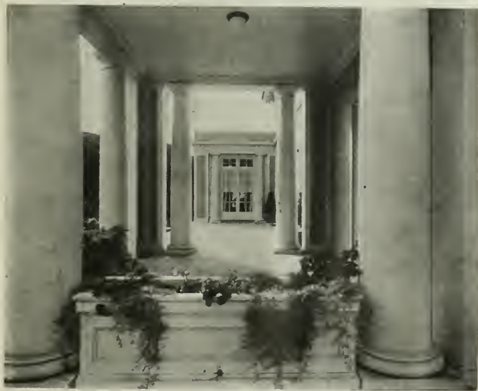
THE PORCH, RESIDENCE OF MR. H. T. JAMES, BURLINGAME HILLS Chas. Peter Weeks, Architect
