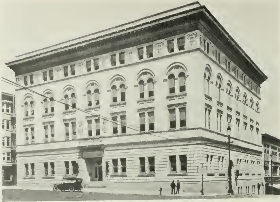
Exterior, Building for Scottish Rite Bodies, San Francisco. O'Brien & Werner Architects.
