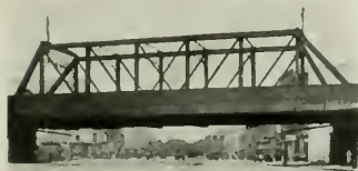
Former railroad bridge over a Philadelphia street, which it was proposed to duplicate to carry more tracks. The Art Jury refused to approve it.
