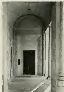
Cloister, Occidental College
