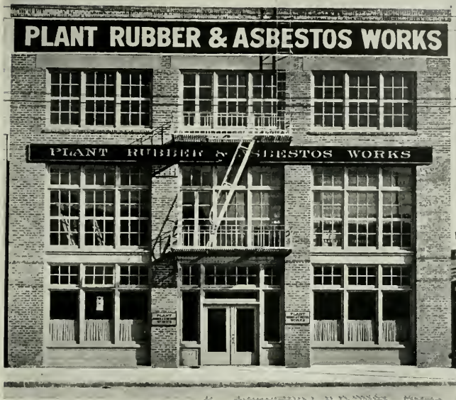
OFFICE AND FACTORY BUILDING, SAN FRANCISCO Coxhead & Coxhead, Architects
