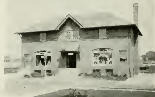
STORE IN AN EASTERN INDUSTRIAL SUBURB Ballinger & Perrot, Architects and Engineers
