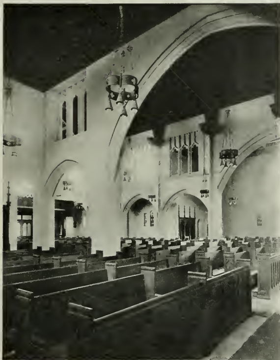
INTERIOR, ALL SOULS' CHURCH, SOUTH SAN FRANCISCO George E. McCrea, Architect
