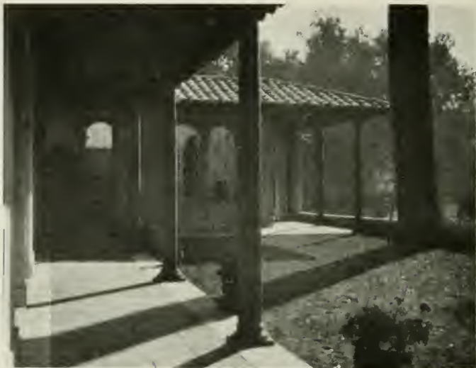
WEST LOGGIA, VILLA OF MR. CHARLES D. BLANEY, SARATOGA, CALIFORNIA Willis Polk & Co., Architects
