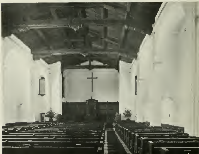
INTERIOR, FIRST CONGREGATIONAL CHURCH, RIVERSIDE Myron Hunt, Architect
