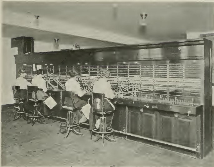
TELEPHONE SWITCHBOARD IN THE SAN FRANCISCO CITY HALL
