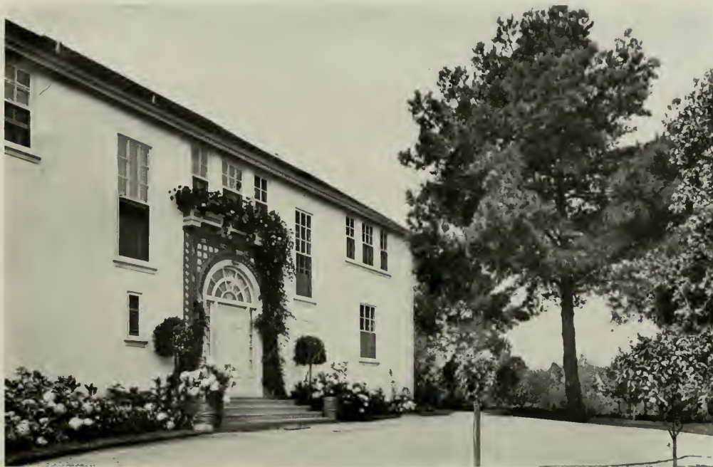
ELEVATION, HOUSE OF DR. W. C. CHIDESTER, SAN MATEO, CALIFORNIA LEWIS P. HOBART, ARCHITECT
