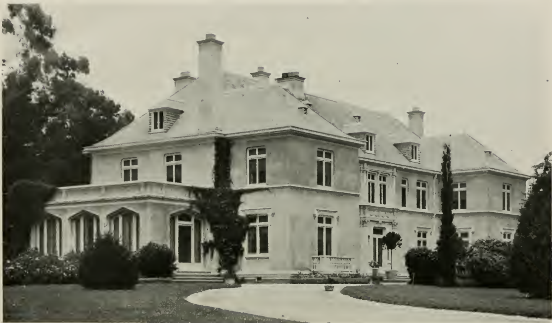
HOUSE OF W. G. HITCHCOCK, ESQ., HILLSBOROUGH, CALIFORNIA LEWIS P. HOBART, ARCHITECT
