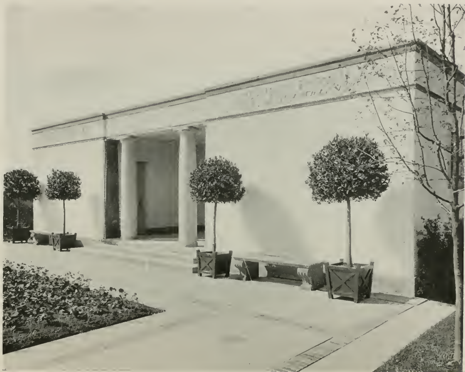
BATH HOUSE, OUTDOOR THEATRE, ESTATE OF GEORGE G. BOOTH, ESQ., CRANBROOK, MICHIGAN. MARCUS R. BURROWES, ARCHITECT
