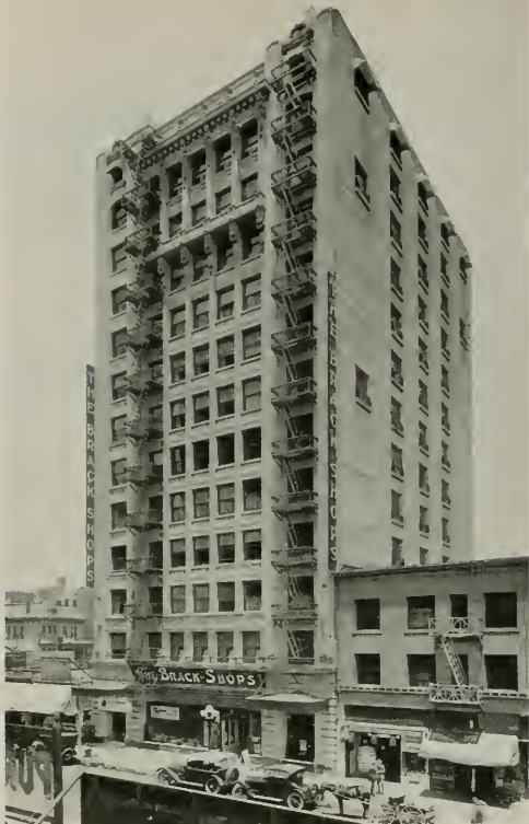
The New "Brack Shops" Building in Los Angeles. Interior partitions throughout are of Buttonlath.
