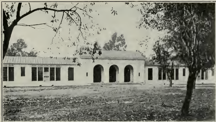
LOCKWOOD SCHOOL, OAKLAND J. J. Donovan and Lewis P. Hobart, Associate Architects
