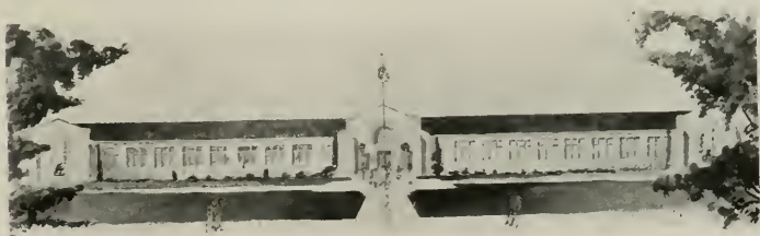
OROQUIETA UNION HIGH SCHOOL. Ernest J. Kump, Architect.
