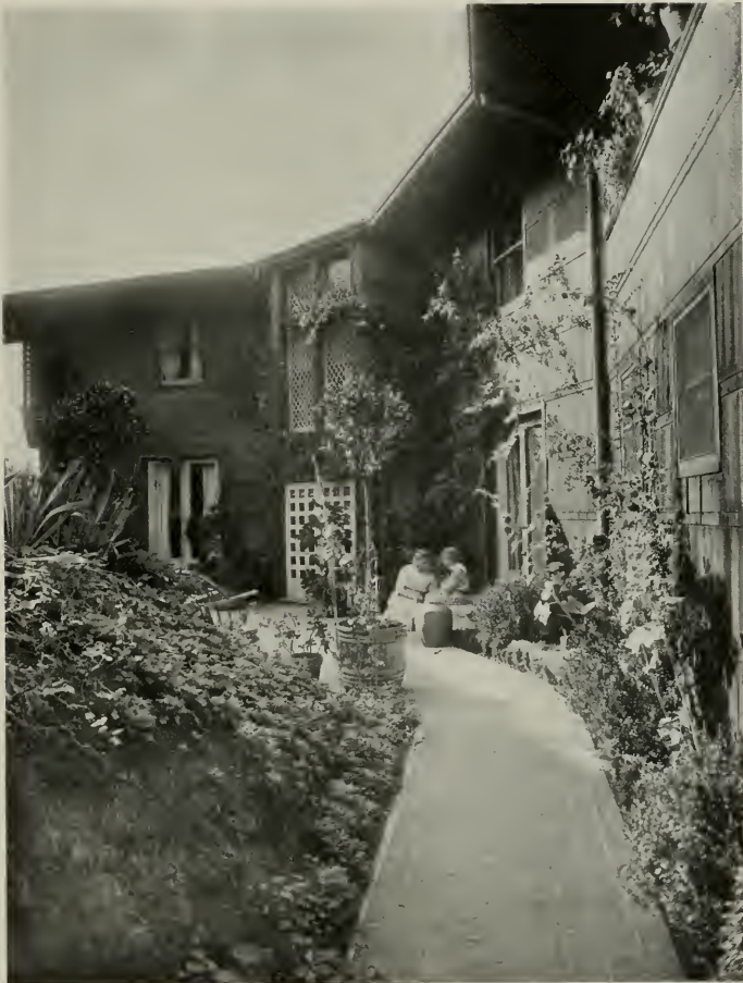
COURT, SHOWING EFFECTIVE LATTICE TREATMENT, HOUSE OF JOHN GALEN HOWARD, BERKELEY
