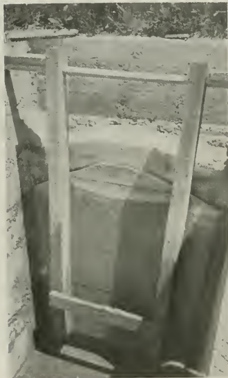
FIG. 1—Automatic Drainage Gate, Ralph Bull ranch, near Arcata, California, on Humboldt Bay. Concrete conduit and wooden cover. Area of conduit approximately 16 square feet. Approximate thickness of concrete 6 inches. The wood gate is not sufficiently sensitive to water level changes.
