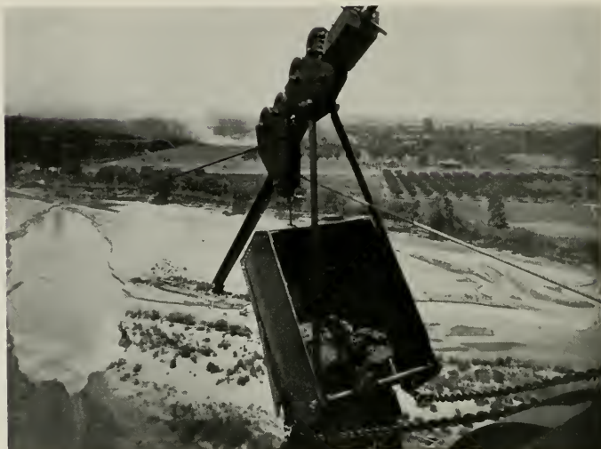
BUCKET CONVEYING RAW MATERIAL FROM GRAVEL PIT TO PLANT
