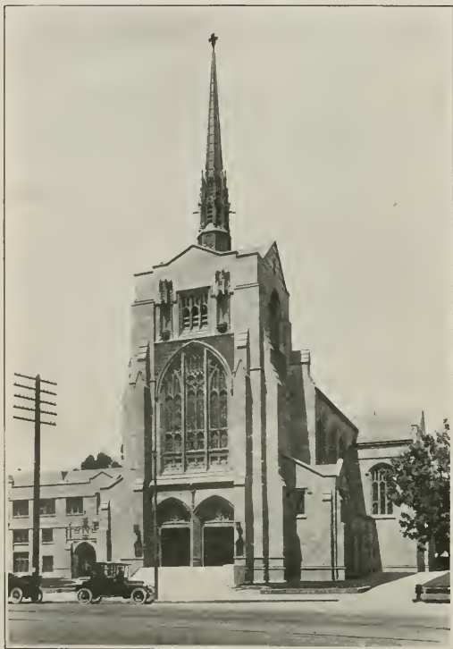
FIRST PRESBYTERIAN CHURCH, OAKLAND William C. Hays, Architect
