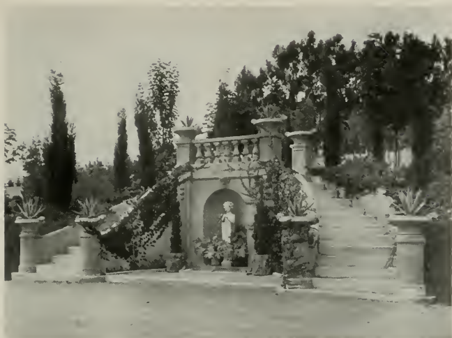
STAIRS AND FOUNTAIN, COUNTRY ESTATE OF MR. THOS. DRISCOLL, HILLSBOROUGH. Louis P. Hobart, Architect.
