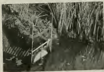
FIG. 5.—Gate partly closed, water rising. 36-inch Automatic Drainage Gate attached to 50 feet of corrugated pipe, installed on Russ Island, five miles west of Vallejo, California. This picture was taken just at the turn of the tide, and shows the gate, slightly open, discharging water. The tall metal extensions which are shown were supplied for the purpose of carrying counter-weights, which were found to be a hindrance rather than an aid and were subsequently removed.
