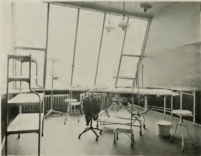
OPERATING ROOM, HANFORD HOSPITAL. Ernest J. Kump, Architect.
