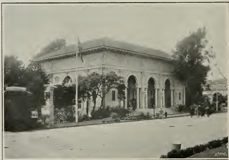
HAWAIIAN BUILDING, P. P. I. E. C. W. Dickey, Architect
