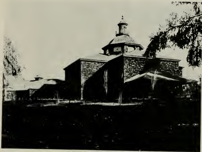
STABLES, MR. J. B. CORYELL, SAN MATEO Willis Polk & Company, Architects
