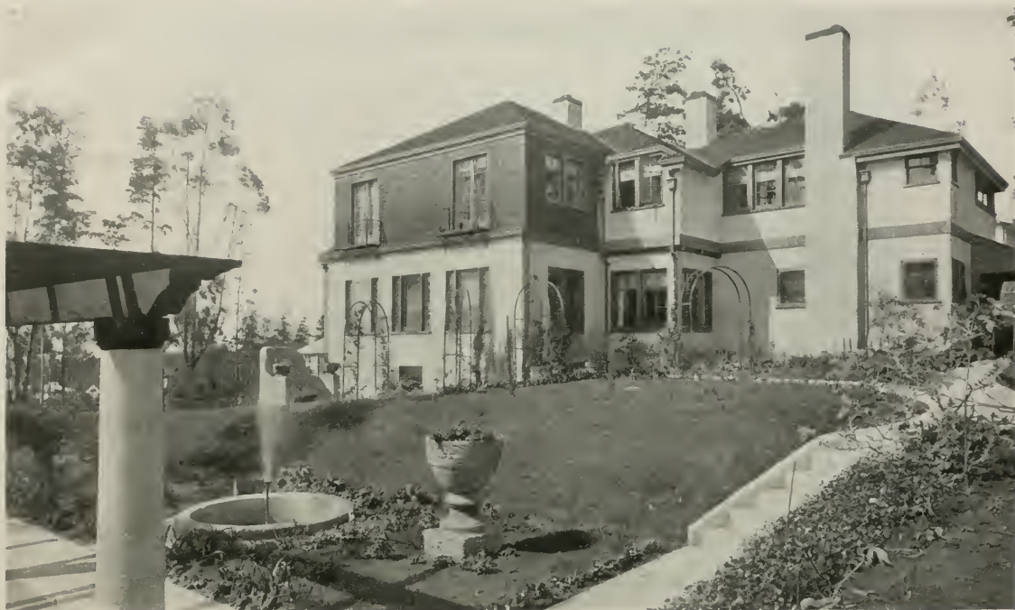
HOME OF MR. FREDERICK M. GIBBS, SIX BENITO WAY, ST. FRANCIS WOOD HENRY H. GUTTERSON, ARCHITECT
