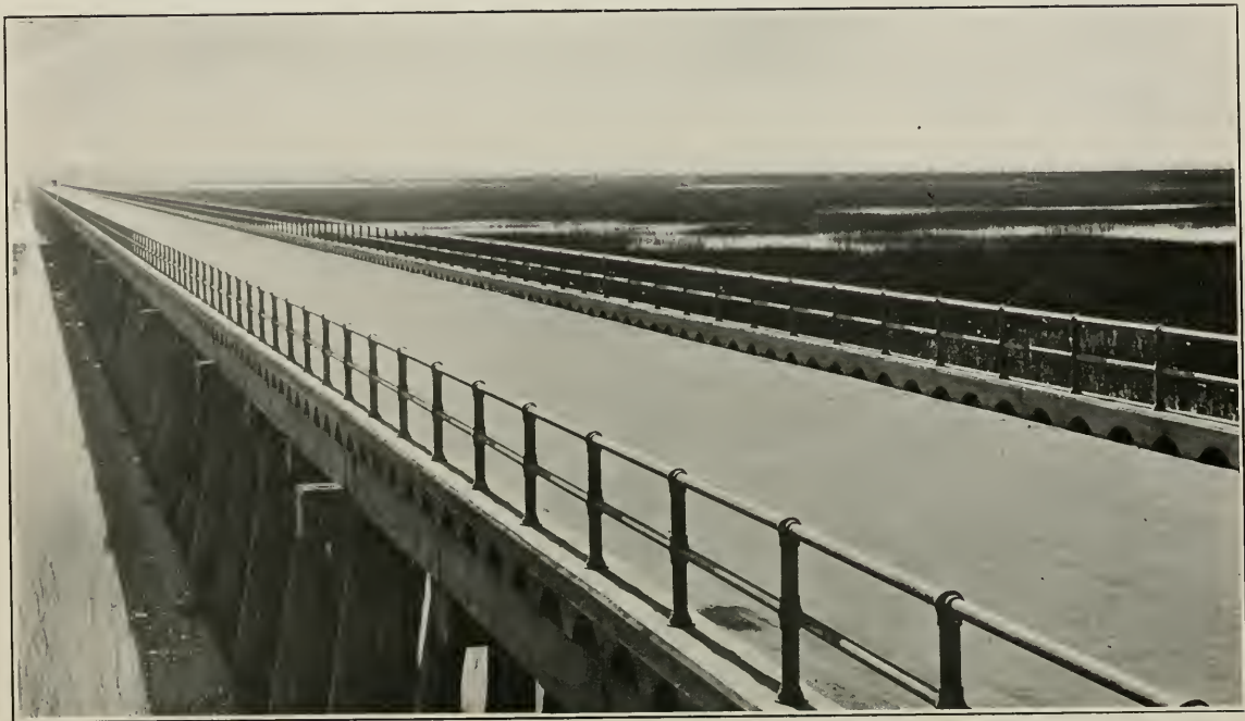
YOLO TRESTLE, CALIFORNIA STATE HIGHWAY AUSTIN B. FLETCHER, CHIEF ENGINEER
