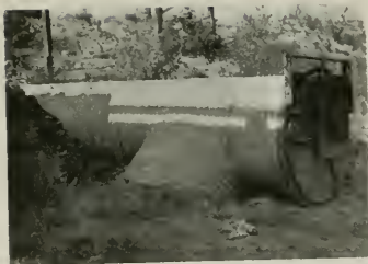
FIG. 4.—48-inch Automatic Drainage Gate, attached to 300 feet of corrugated pipe, installed on Reclamation District No. 1000, about twenty miles north of Sacramento, California.
