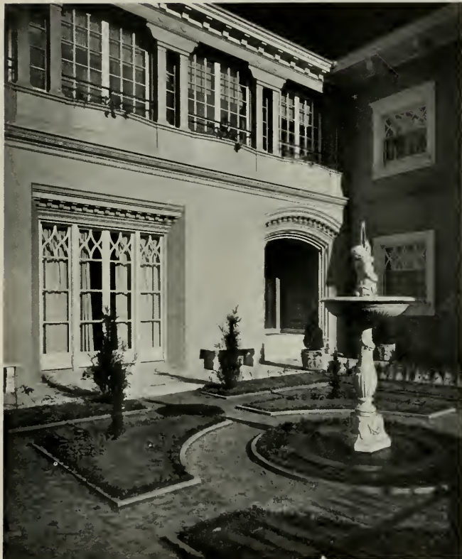
COURT, HOUSE OF MRS. H. C. MOFFITT, PIEDMONT WILLIS POLK & COMPANY, ARCHITECTS
