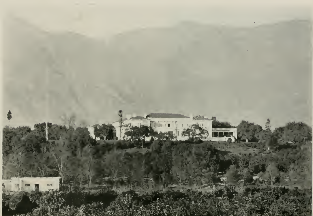
RESIDENCE OF MR. HENRY E. HUNTINGTON, PASADENA, CALIFORNIA MYRON HUNT AND ELMER GREY, ARCHITECTS
