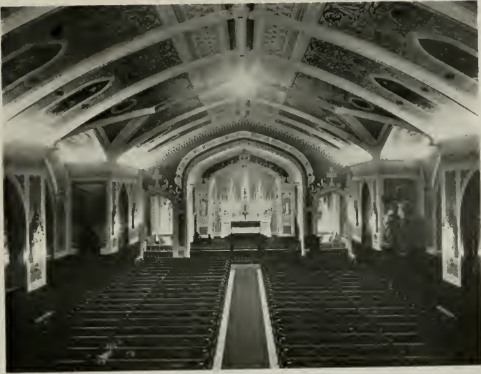
INTERIOR ST. JOHN'S CHURCH, FRESNO. Ernest J. Kump, Architect.
