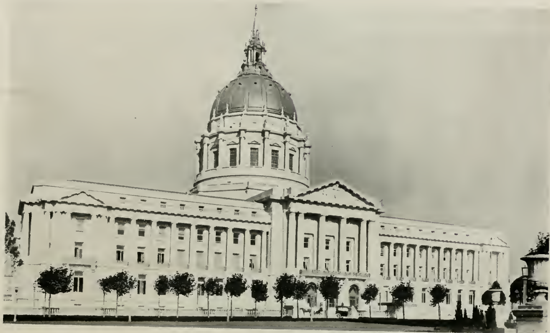
SAN FRANCISCO CITY HALL, VIEW FROM CIVIC CENTER BAKEWELL & BROWN, ARCHITECTS
