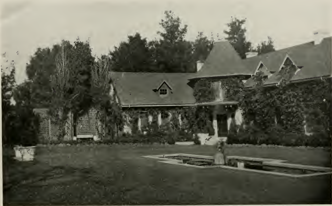
GARDEN ELEVATION, HOUSE OF R. M. TOBIN, ESQ., HILLSBOROUGH, CALIFORNIA LEWIS P. HOBART, ARCHITECT
