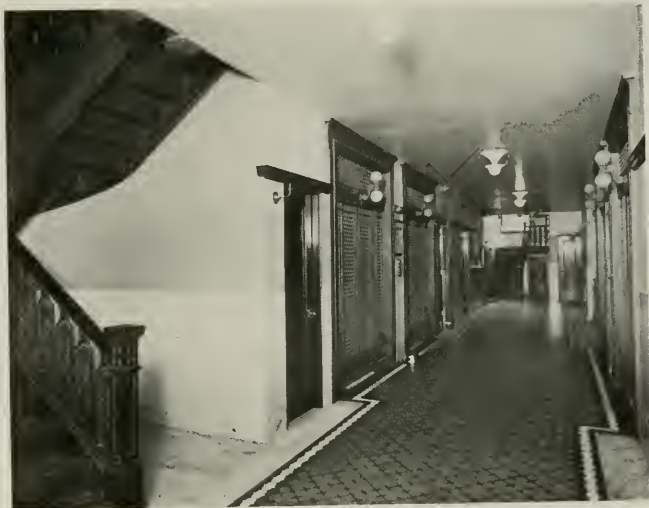
TYPICAL CORRIDOR, STANDARD OIL BUILDING, SAN FRANCISCO BENJ. G. McDOUGALL, Architect
