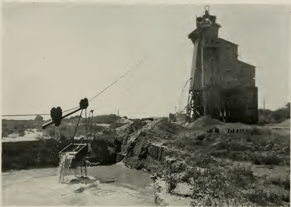
EXCAVATING FROM UNDER WATER, CALIFORNIA BUILDING MATERIAL COMPANY'S PLANT, NILES
