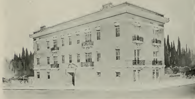
RESIDENCE FLATS FOR MR. M. SPIRO, SAN FRANCISCO Heiman & Schwartz, Architects J. S. Malloch, Builder
