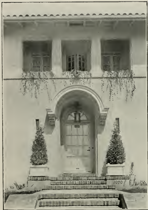
RESIDENCE T. W. FORREST Schirmer, Bugbee & Co., Architects
