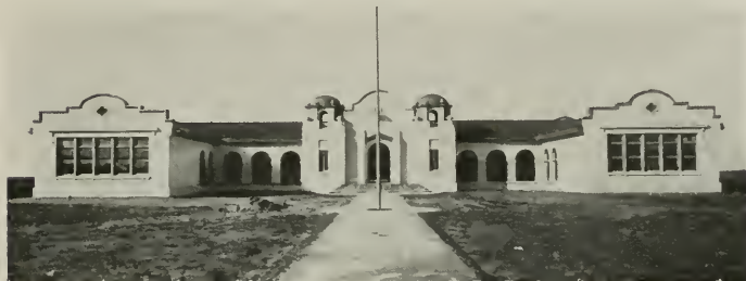
CARRUTHERS UNION HIGH SCHOOL. Ernest J. Kump, Architect.
