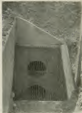
FIG. 8.—Intake end standard drain for water pocket. The lower pipe has Automatic Drainage Gate on opposite end, and runs thro' levee into canal. The upper pipe is an inverted siphon used to carry the run off beneath the canal when flood water in the canal is too high to permit operation of the gate. Water thus entering the District is permitted to drain naturally to the river levees, where it is caught in sumps and pumped into the river.
