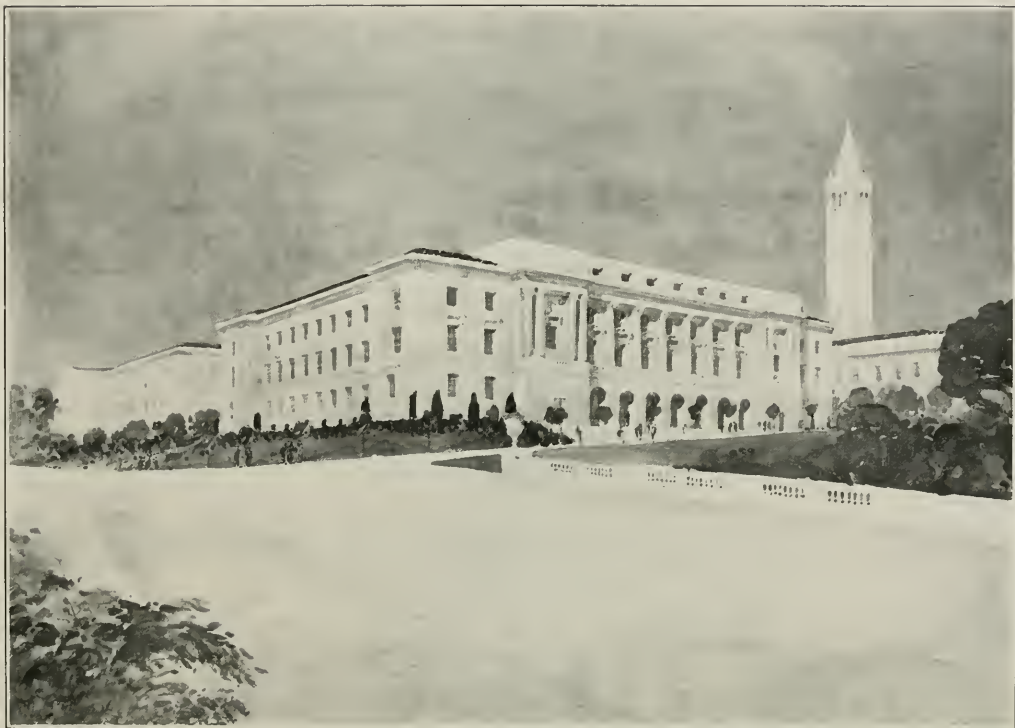
CLASS ROOM BUILDING, UNIVERSITY OF CALIFORNIA, BERKELEY JOHN GALEN HOWARD, ARCHITECT
