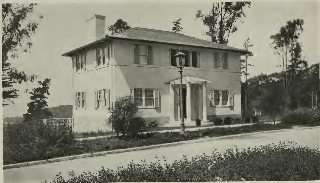
HOUSE OF MR. L. J. DAVIS, ST. FRANCIS WOOD HENRY H. GUTTERSON, ARCHITECT
