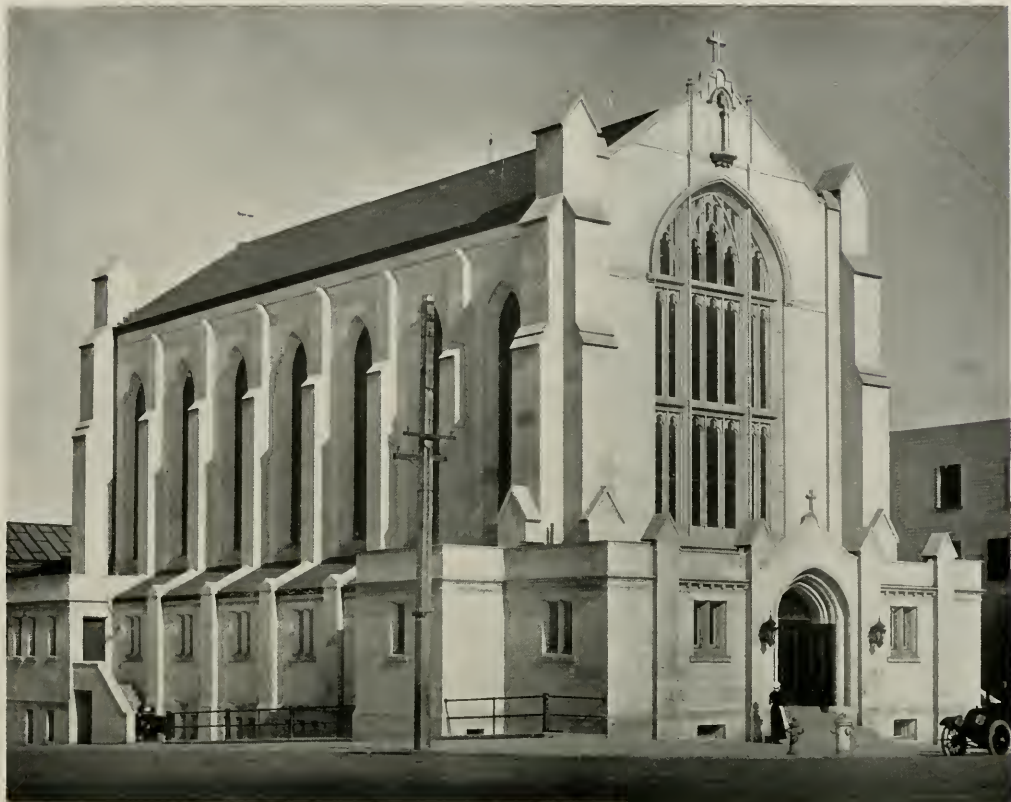
ST. LUKE'S CHURCH, VAN NESS AVENUE, SAN FRANCISCO BENJ. G. McDUGALL, ARCHITECT
