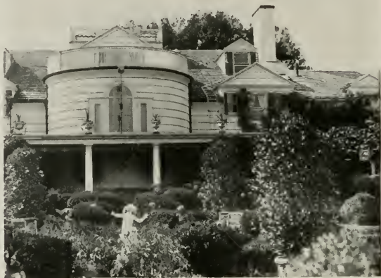
FIG. 1. Day view of the residence of J. L. Breese, showing the arrangement of the projector units on the roof of the porch for lighting this garden, and also in the foreground the two box lights for lighting the fountain.
