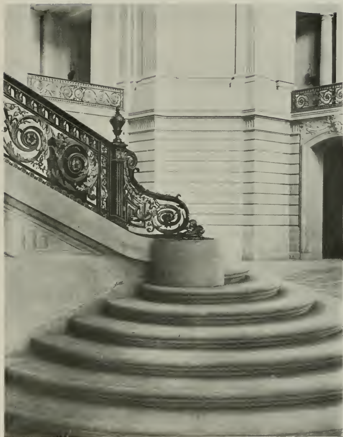
SAN FRANCISCO CITY HALL, DETAIL OF ROTUNDA STAIRS BAKEWELL & BROWN, ARCHITECTS
