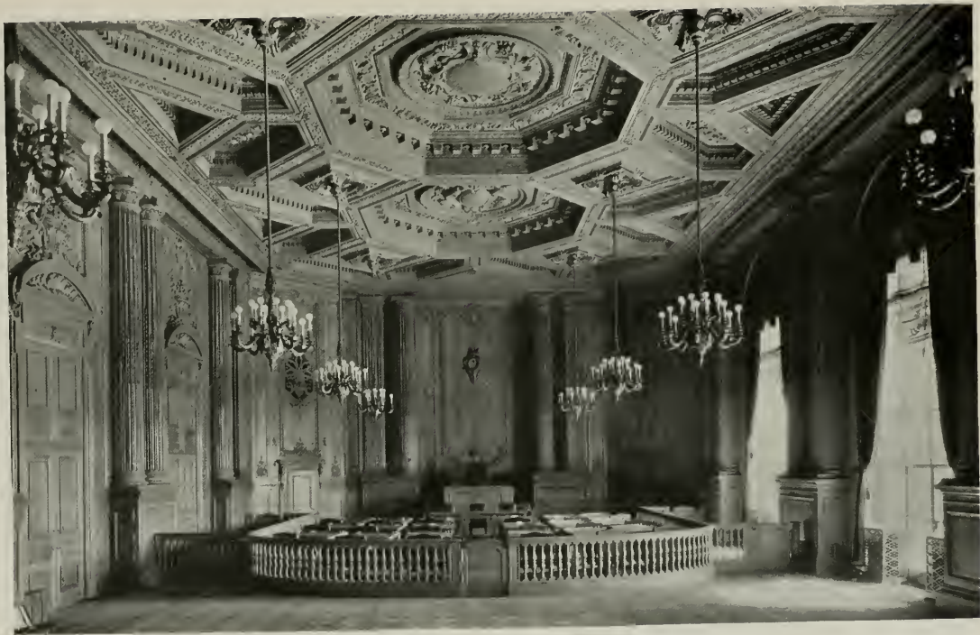
SAN FRANCISCO CITY HALL, COUNCIL CHAMBER BAKEWELL & BROWN, ARCHITECTS
