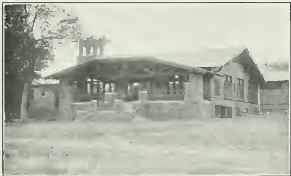
Norfolk Hotel, Norfolk, with Open-Air Section Norman F. Marsch, Los Angeles, Architect
