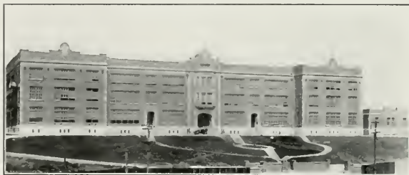
Roman Catholic Orphan Asylum, San Francisco Smith O'Brien, Architect Wiring by National Electric Company
