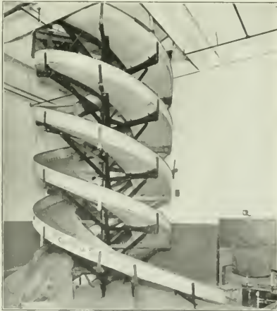
Double and Triple Chutes Are Used to Advantage
