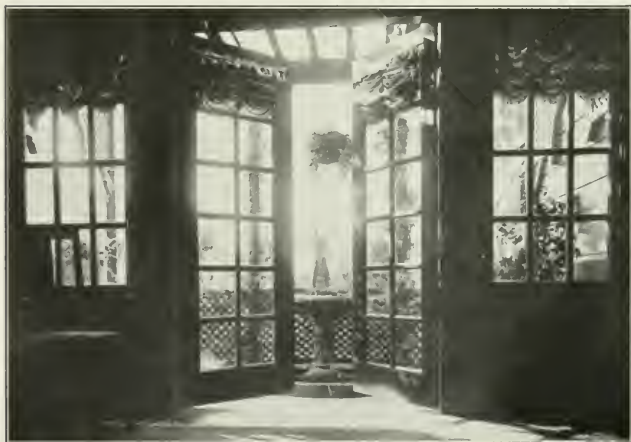
Residence of Irwin Barr, San Francisco Fabre & Bearwald, Architects
