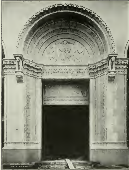
Entrance Masonic Temple, San Francisco Bliss & Fawcett, Architects
