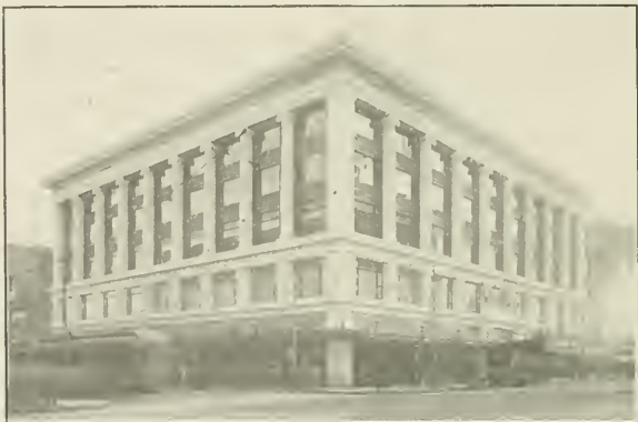
U.S. Post Department Store Building, San Francisco Architects: MacDonald & Bailey, Chicago
