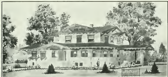
Country Residence of Mr. J. H. Wheeler, near St. Helena, California L. M. Turton, Architect
