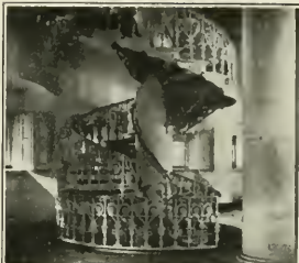
CIRCULAR IRON STAIRS IN HALL OF RECORDS, SAN FRANCISCO. Erected in 1870.
