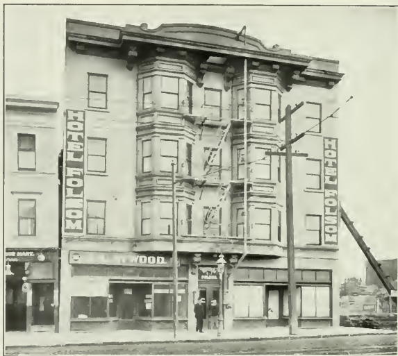
Hotel Folsom, San Francisco, Showing How Building Has Settled
