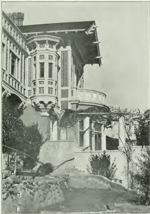
Residence of Eugene H. Christensen, L. S. Architect Thomas L. Primm, Architect
