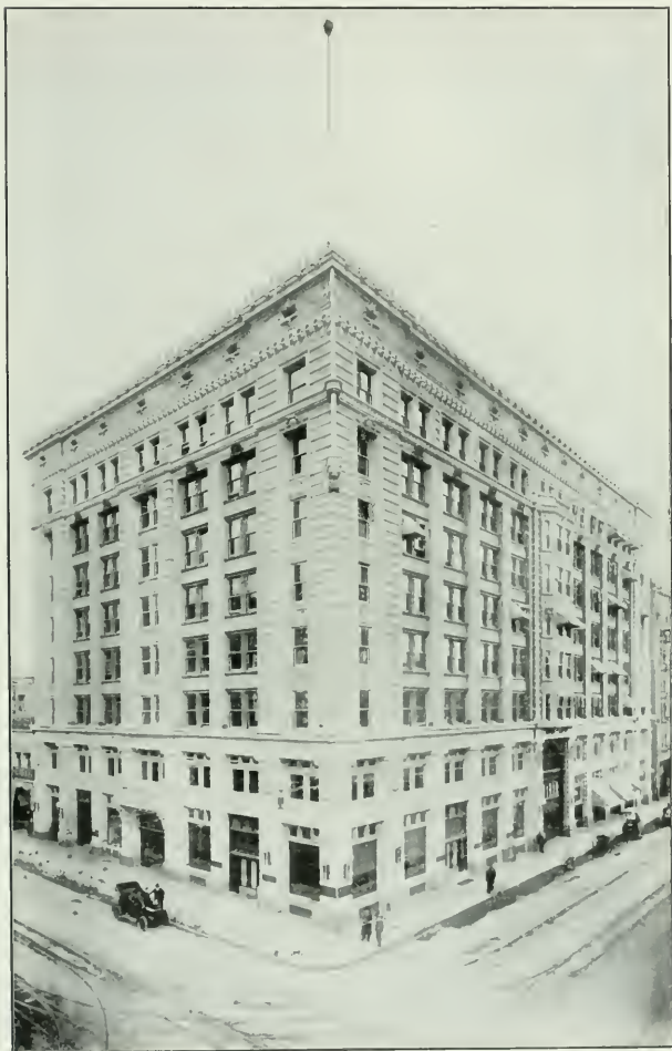
Herman W. Hellman Building, Los Angeles Alfred F. Rosenheim, Architect
