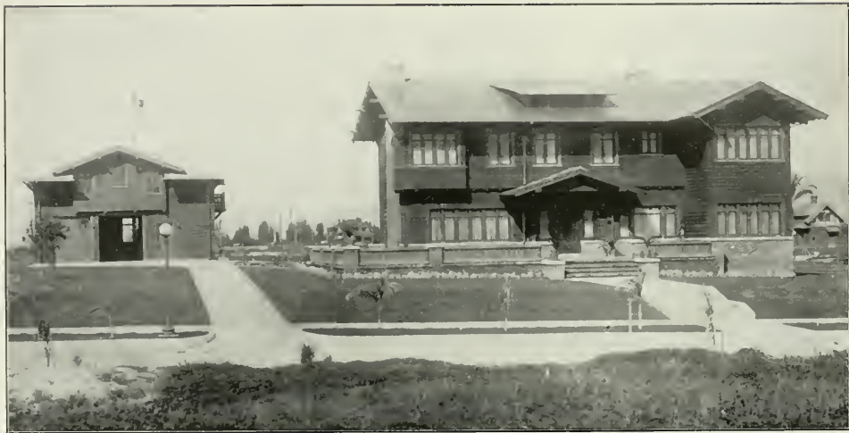
A Los Angeles Residence and Garage Alfred F. Rosenheim, Architect
