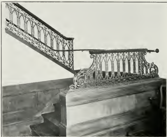
Ornamental Iron Staircase, Knights of Columbus Building Executed by California Artistic Metal & Wire Company
