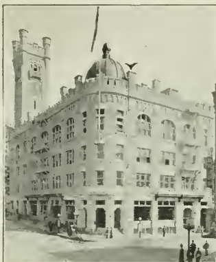
Times Building, Los Angeles, Cal. Foundations Waterproofed with Ceresit.
