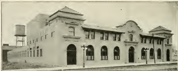
HY-RIB Concrete Sidings (Built Without Forms) Sunset Publishing Co., San Francisco, Cal. Geo. W. Kelham, Architect
