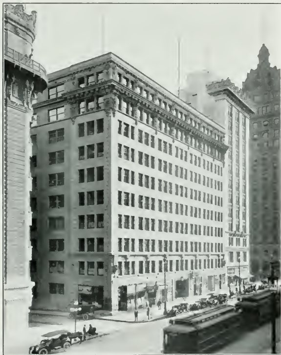
Mack Building, San Francisco*
