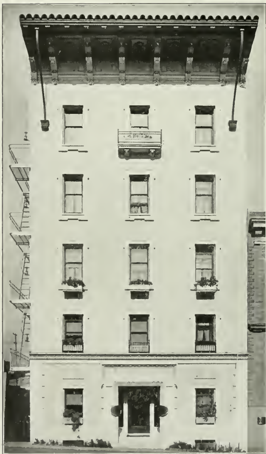
Hotel Hamilton, San Francisco. Charles Peter W. Smith, Architect.
