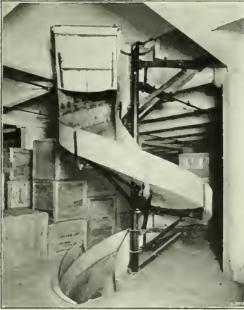
Showing Fire-door and Smoke Baffle under ceiling.
