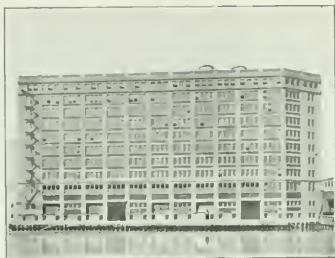
Wenalen Warehouse, Philadelphia, Price, Scott & Co., Architects.
