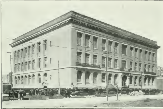
Commercial High School Propped on Rollers Ready to be Moved
