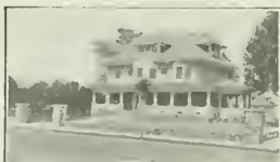
Residence of Mrs. Clara F. Taylor, DeLand, Fla. Roofed with J-M Transite Asbestos Shingles.
