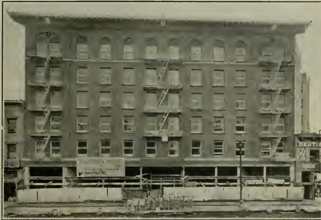
Terminal Hotel, San Francisco, California
