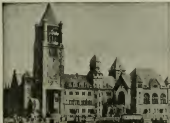
Ceresit waterproofing was used in the construction of the German Emperor's Castle at Posen
