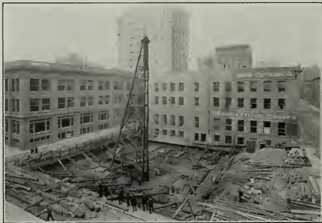
The New Way of Driving Piles With "Dummy" Steam Engine
