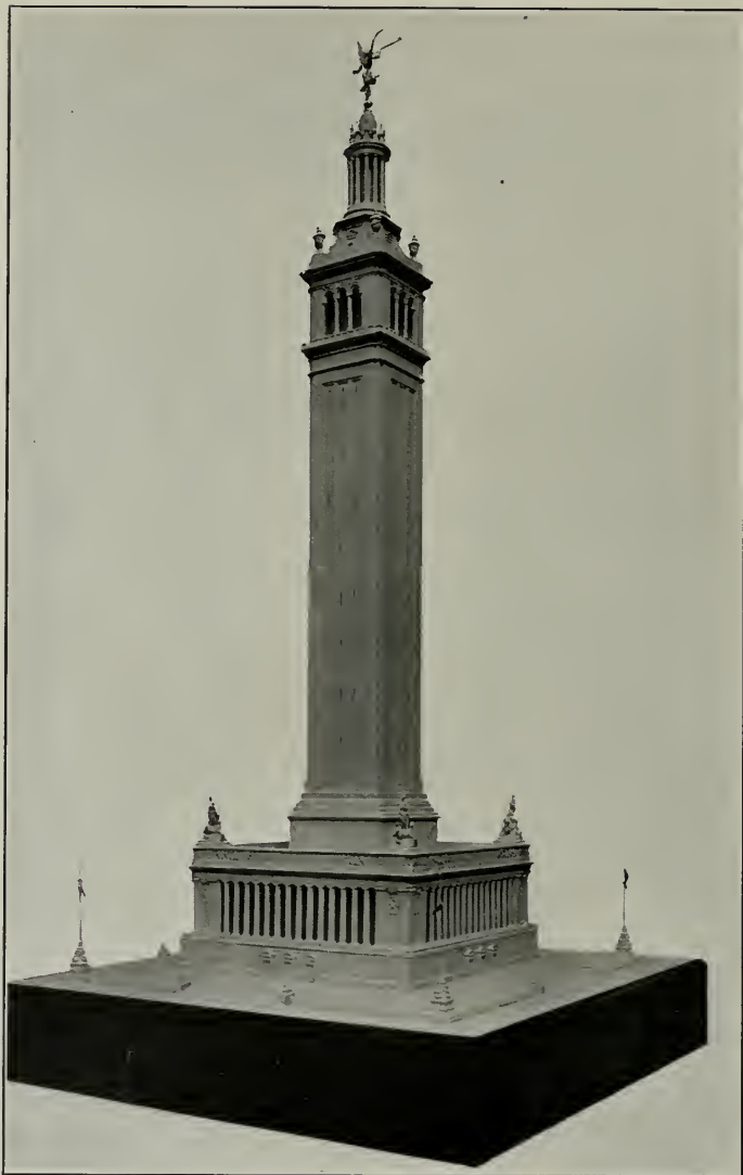
Imposing memorial tower, the first structure formally sanctioned for erection on the proposed site of the Panama-Pacific Exposition, San Francisco. Designed by H. L. Pelton and P. E. Fergusson. The tower, which is to be a permanent structure that will revert to the city, is to be 850 feet in height above the ground level, and, with the single exception of the Eiffel tower in Paris, will be the tallest structure in the world. It will cost $1,500,000.
