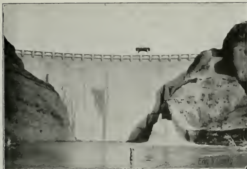
Fig. 4.—Downstream Face of East Park Dam
