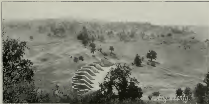
Fig. 6.—General View of Concrete Spillway for East Park Dam
