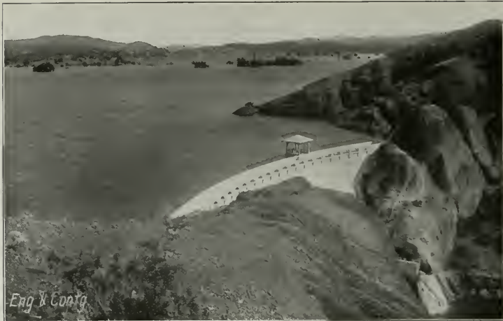
Fig. 5. General View of East Park Dam and Reservoir
