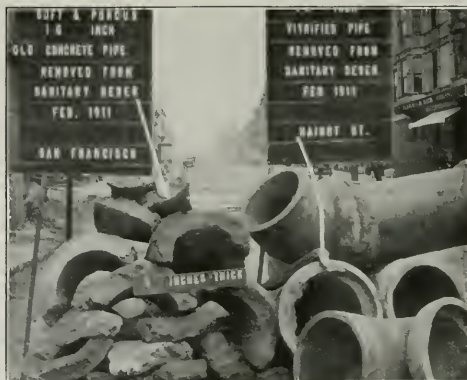
Fig. 3.—Showing comparative condition of concrete and vitrified pipe removed from a sewer in San Francisco, February, 1911.
