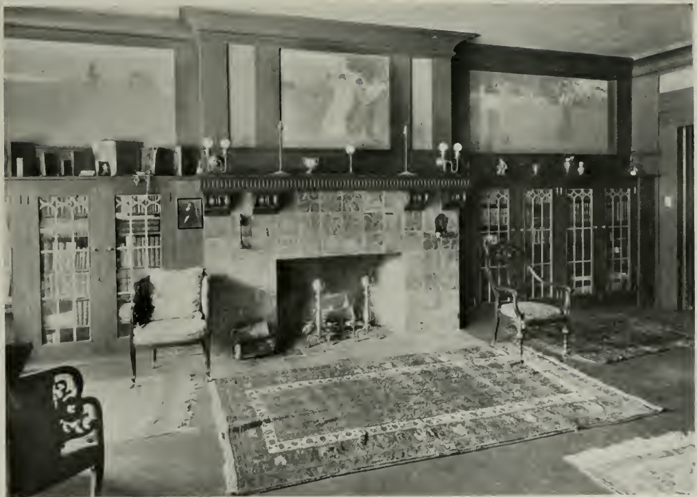
Library in Mr. Rudolph Taussig's Residence, San Francisco
