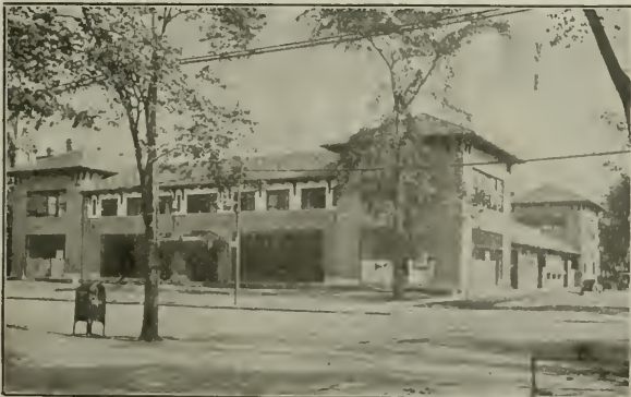
Ferrocimcave was used for Roof of this Garage
