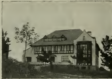
Residence of Mr. Alexander Pantages, Seattle, Wash. Loveless & Wilson, Architects. Neposet Waterproof Building Paper Used.
