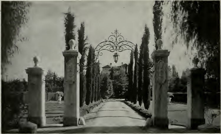
The Italian Villa as Found in California has no Counterpart in Italy
