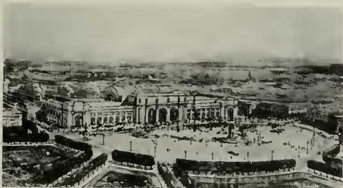
Station at Washington, D. C.—A Convenient and Attractive Entrance to a City
