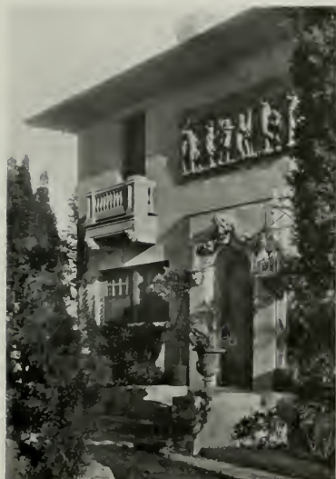
A Detail of the Rowayton Villa Slee & Bryson, Architects, Brooklyn, New York
