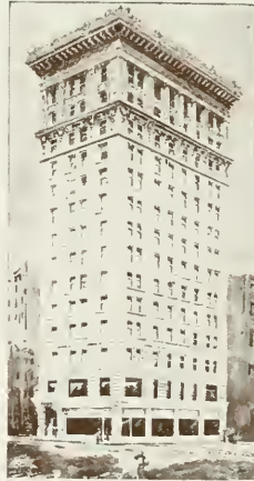
HEWES BUILDING Entirely Equipped with Haas Hydrometers
