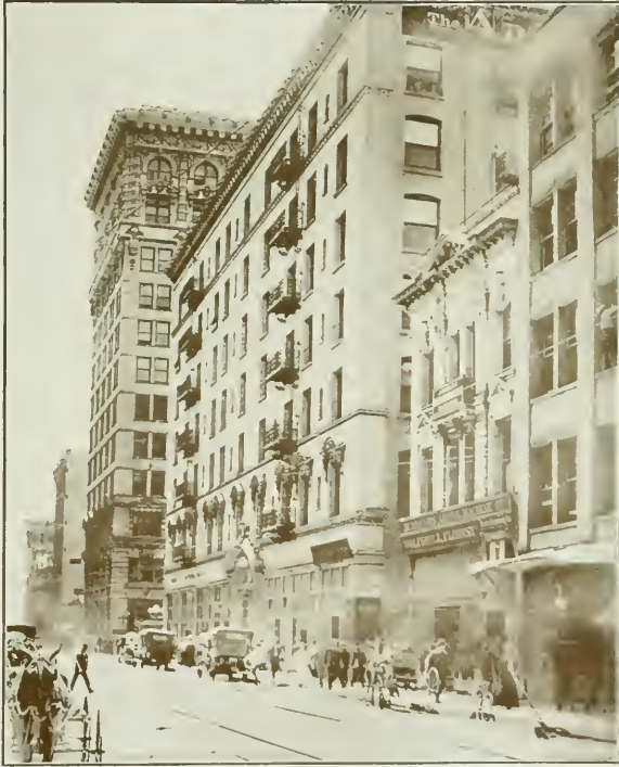
Detail of Union Trust Building, and Street North of ... Ingleby Hotel and Trust Building
