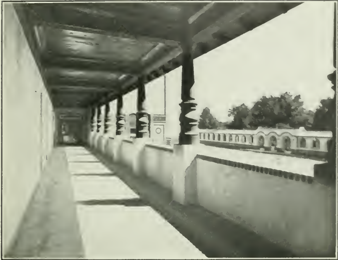
Looking West from Second Story Open Corridor
