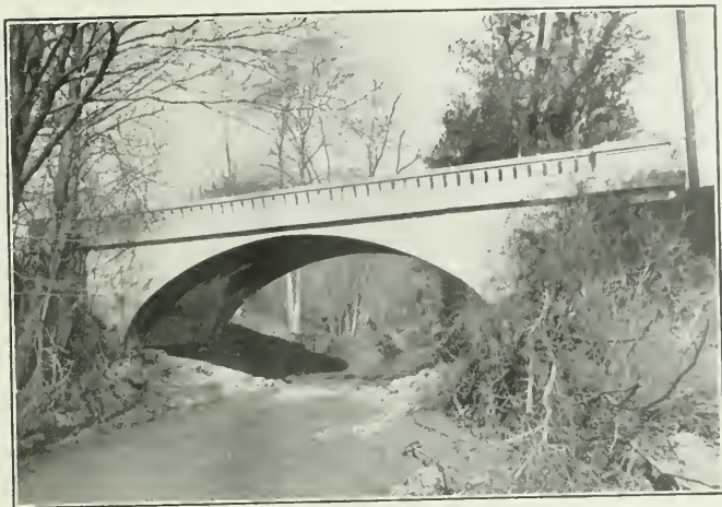
Fig. 6—Reinforced Concrete Arch Bridge, City of Ross, Marin County, California John B. Leonard, Engineer
