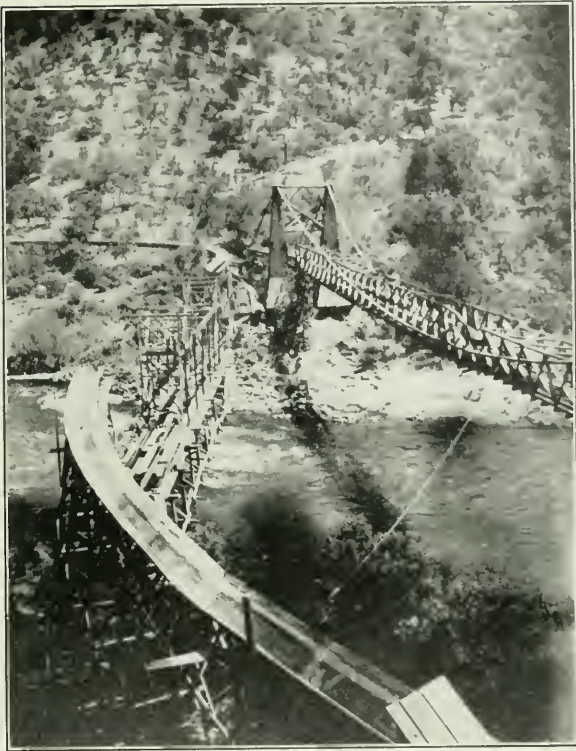
Old Suspension Bridge Across Kings River, California, on the Right; New Steel Bridge Under Construction, on the Left
