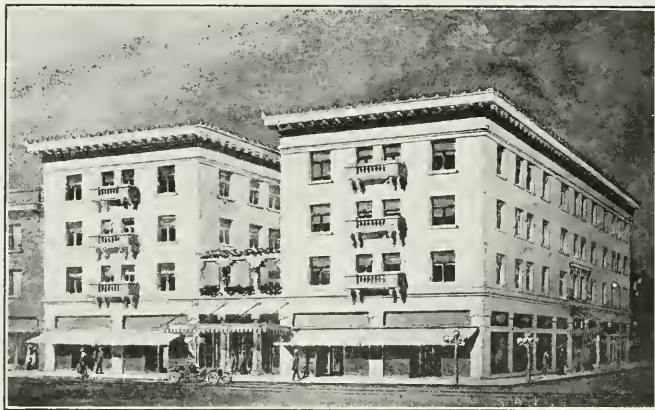
Hotel for the Conservative Realty Company, San Jose William Binder, Architect
