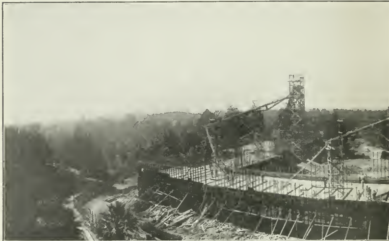
Progress Work, California State Normal School
