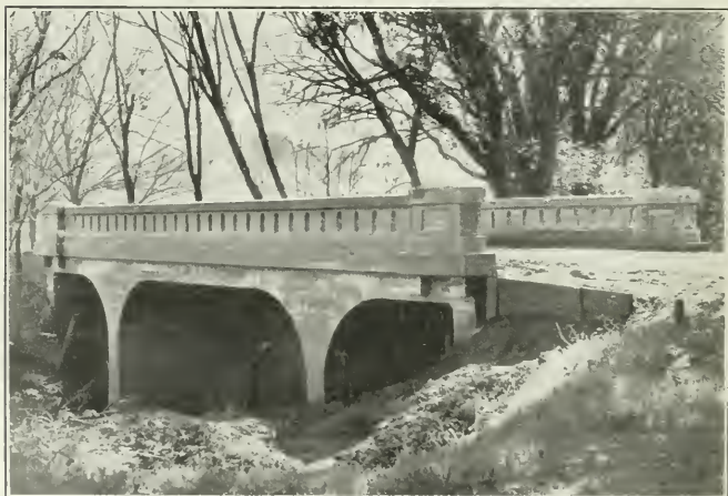
Fig. 5—Reinforced Concrete Flat Slab Bridge, City of Ross, Marin County, California John B. Leonard, Engineer
