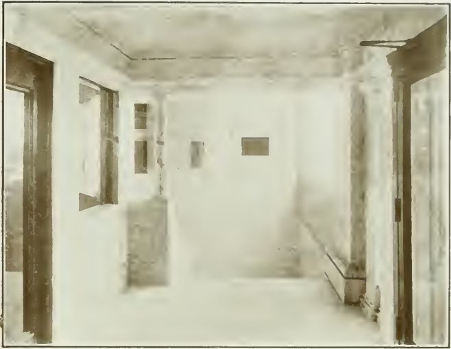
Entrance to Safe Deposit Department, Security Savings Bank Building
