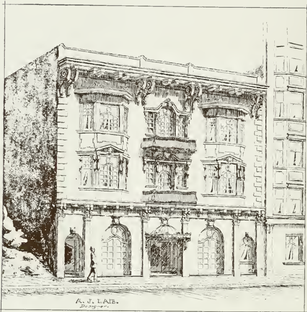
Halstead Building, San Francisco Faced with Stockton White Enamel Brick
