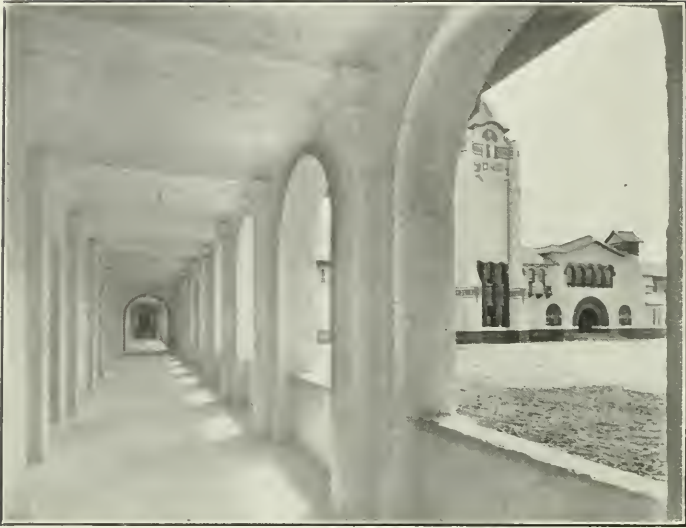
Arcade, Showing Massive Concrete Arches
