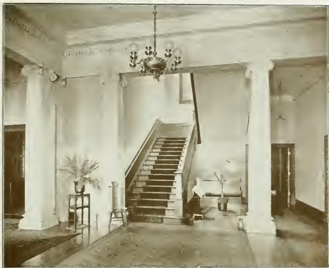
Interior, Bresee Bros. Building
