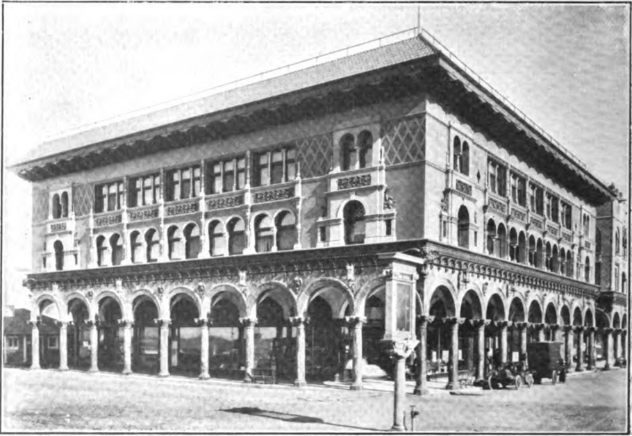
Hotel Saint Marks, Venice. Photos by Graham, Los Angeles.
