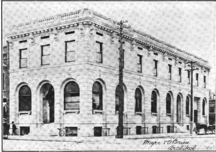
Bank of Bakersfield.
