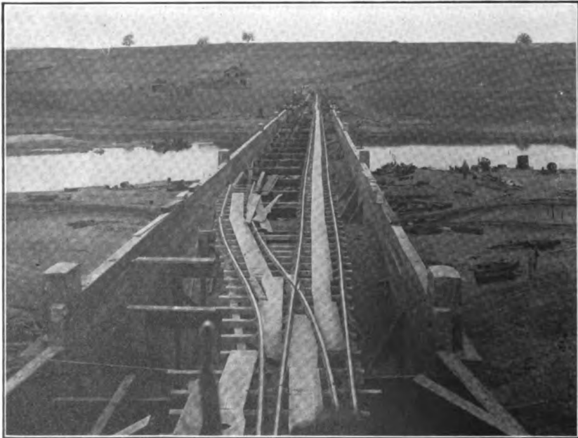
Reinforced Concrete Bridge, Pollasky. View Showing Walls and Buttresses; also Service Track.
