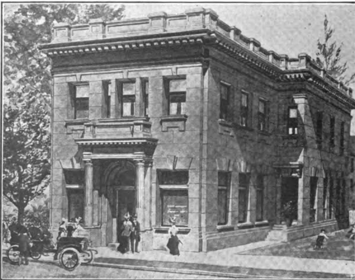
Homestead Loan Association Building, Berkeley C. W. Dickey, Architect. C-222 Stone Furnished by Andrew T. Hunt
