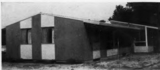
SIDING-SHEATHING method developed by the Douglas Fir Plywood Association is termed Sturd-i-wall construction.
