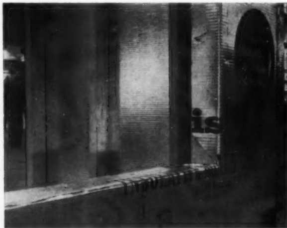
INSULATED SHEATHING is provided by St. Regis Insulative Board. Material is said to have more than 3 times the insulation value of other sheathing. It is perforated for breathing, can be nailed or stapled to studs, is strong and bendable. (M 80, p. 145.)
