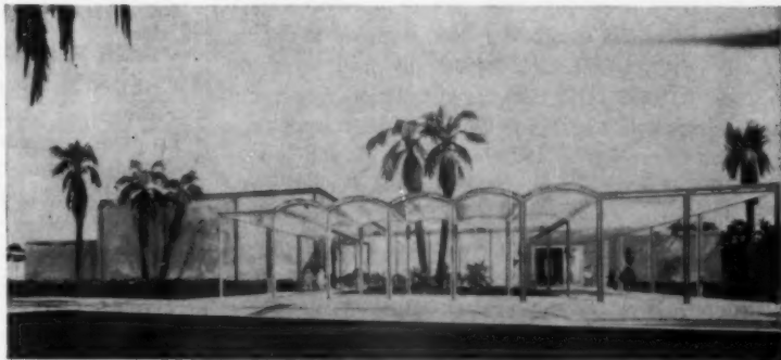
AIR CONDITIONING GOES TO SCHOOL: In Dayton, Southeast Texas, this windowless masonry elementary school is going up at cost of $9.32 per square foot.
