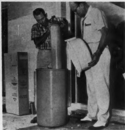
WHAT ↑ AT BUILDING SITE: Water softener unit is assembled. Lindsay man puts Zeolite-filled fiber glass softening unit into its plastic tank. HOW ↓
