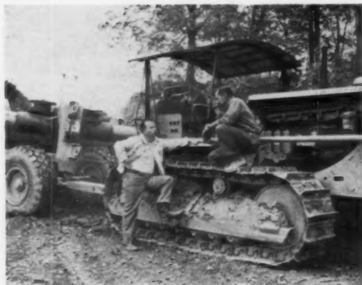
BIG RIG —Builder Ed Mears talks over a haul problem with his operator perched atop Caterpillar D8 tractor drawing a DW21 scraper. Rig takes dirt from high ridge and carries it to dam for balanced earthmoving job.
