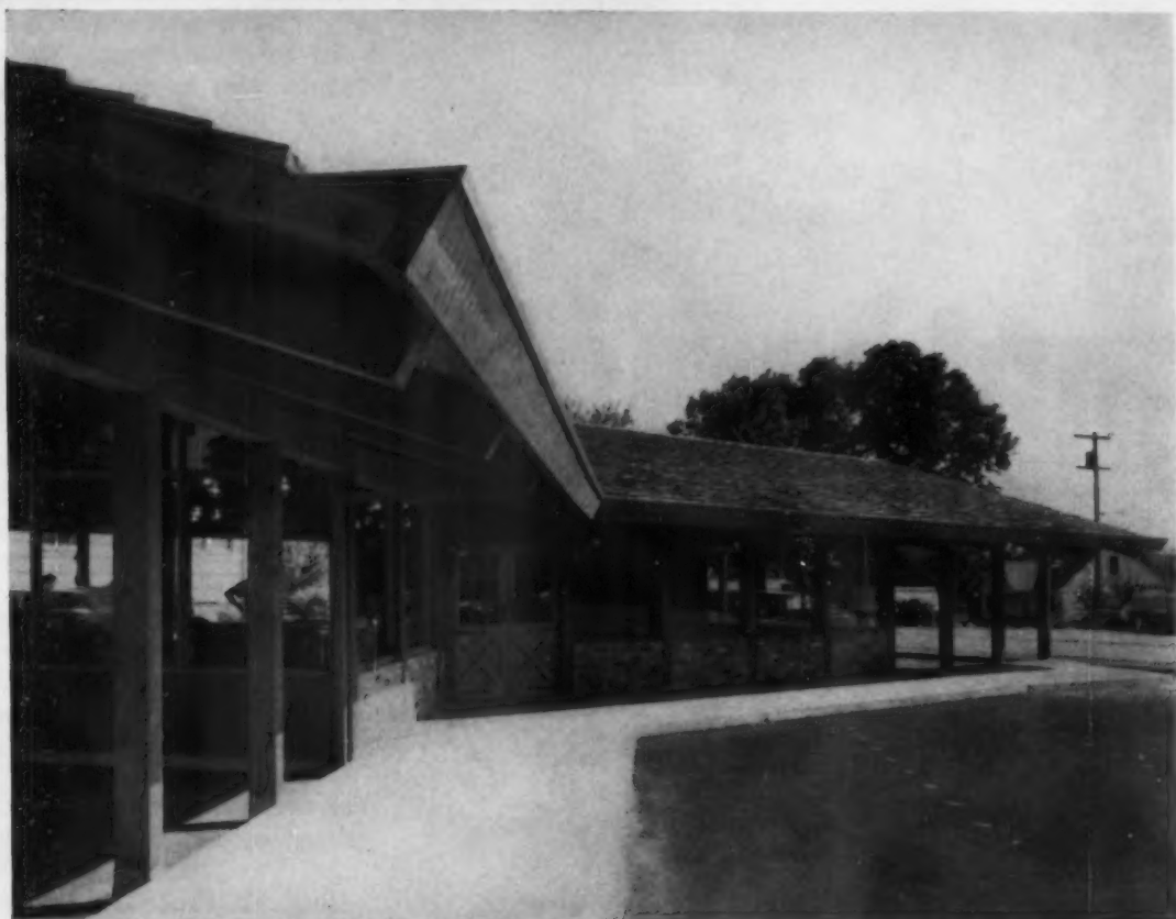
READY TO GROW: Milwaukie, Ore., bank has roof up, wiring in two expandable wings. Enclosed area is 2,475 sq ft, extensions, another 1,170 sq ft. Designed by Logan & Murtaugh, A.I.A., built by Frank Ralph & Son, Portland.
