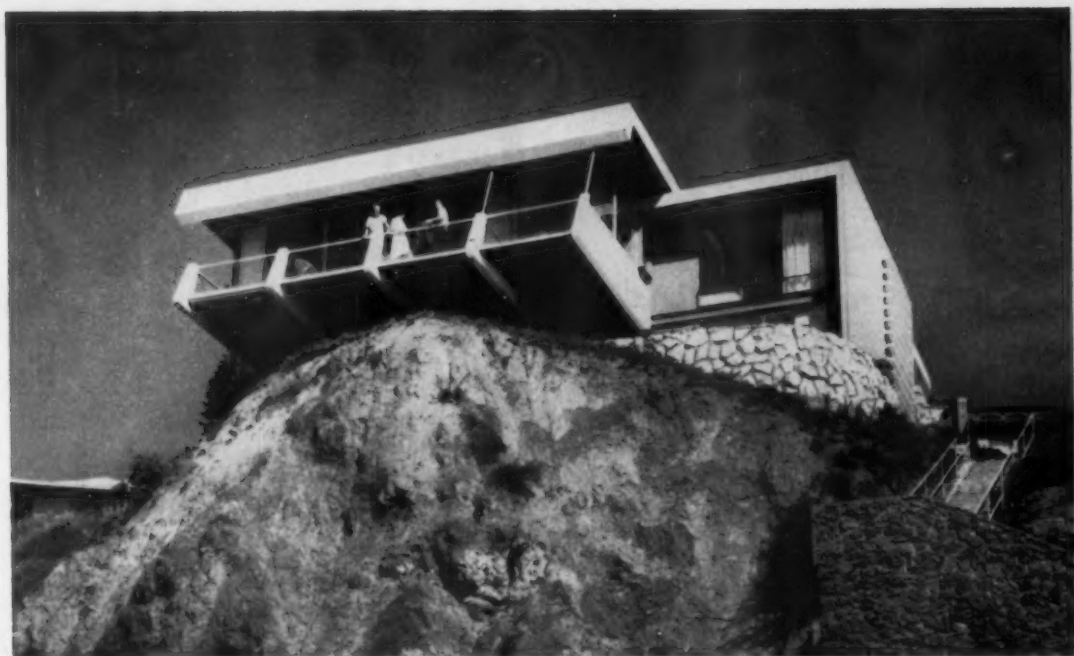
TWO-STORY STEEL house perches on cliff 70' above highway and beach. Sun deck cantilevers 16 feet over the cliff.
