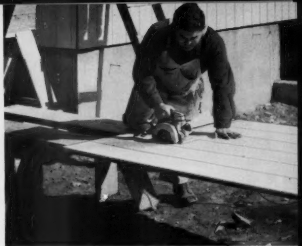
EASY TO SAW AND NAIL. Medema Builders say Insulite Primed Siding "cuts easily with hand or power tools—won't crack, split or splinter." And because its density is close to that of natural wood, no special nails are needed.
