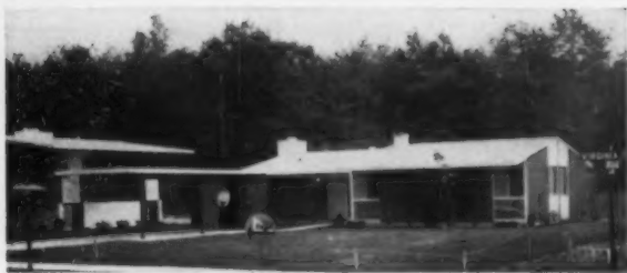
THE VIRGINIAN —This component house features 1,344 sq ft with walls of Texture 1-11 or medium density overlay plywood.
