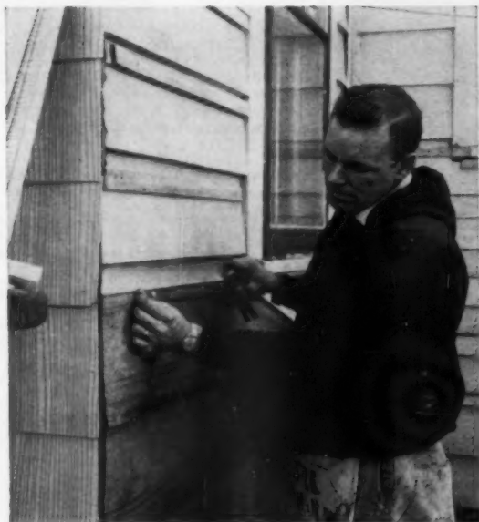
WHEN WOODEN STRIP method is used, strips are nailed over asphalt felt. Then asbestos-cement siding is nailed to hang \frac{1}{8} " or so below the strip. This acts as a drip mold, protects wood from weather, and gives good shadow line.
