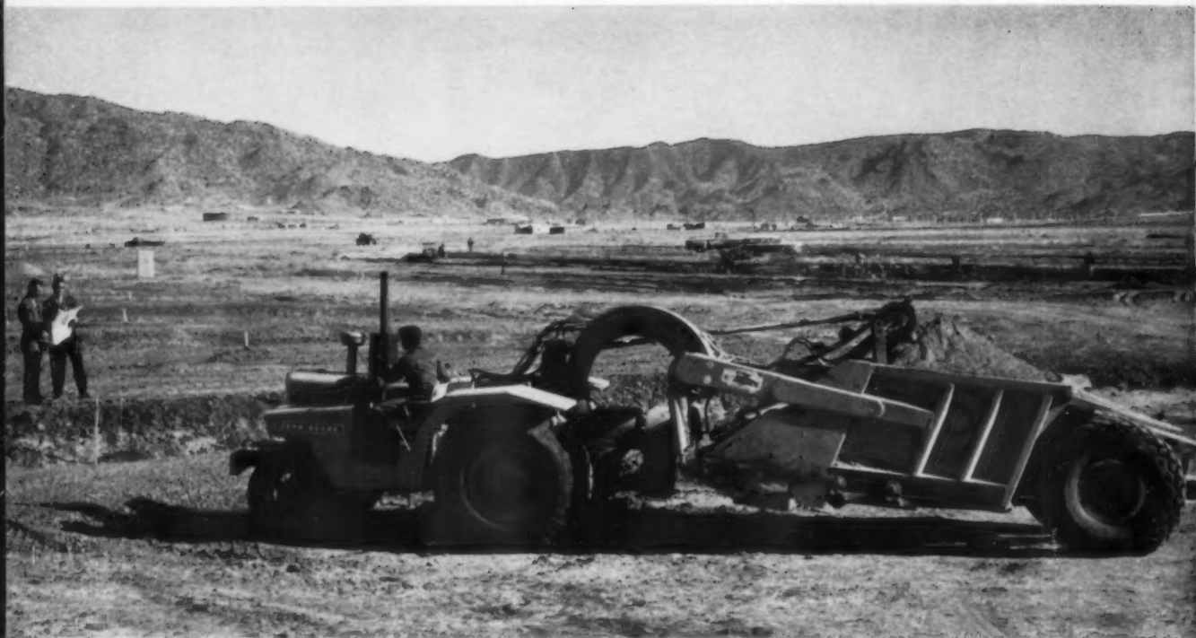
PRODUCTION —Bob Baker, chief engineer for Dale Bellamah homes (left) and Dutch Richardson of Equipment Sales Co., his dealer, view terracing operations on a Bellamah job. Bulldogs of Bellamah fleet are John Deere-drawn Hancock belt loaders.
