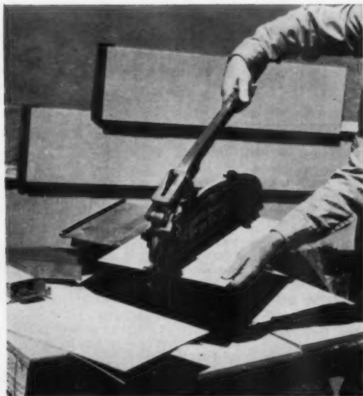
CARPENTER'S BEST FRIEND , working with asbestos-cement materials is a cutter. It not only shears straight cuts, but nibbles curves and cutouts for fitting around chimneys, window and door openings, and other irregularities.
