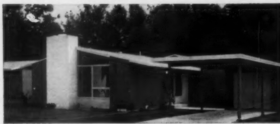
THE WILLIAMSBURG —This model reflects the design range possible with Sturd-i-wall. Carport panels are not insulated.
