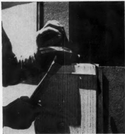
METAL STRIP offered by some manufacturers serves dual purpose. It provides attractive shadow line, and, at same time, seals bottom edge. Normal procedure is to nail along with strip, follow with board. Strip is guide.
