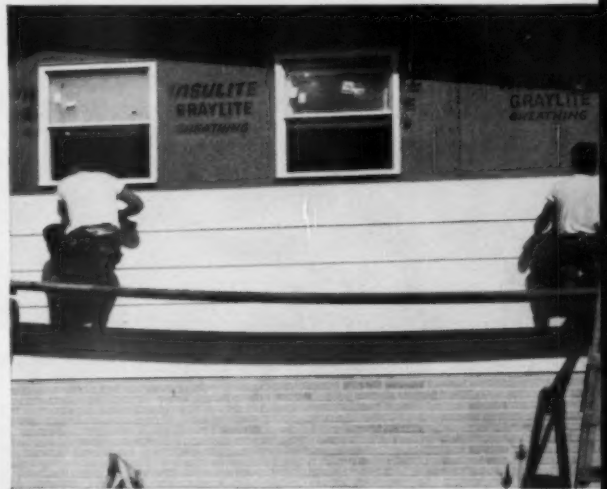
GOES UP FAST. Here's how Medema Bldrs. put it: "Insulite Primed Siding is easy to handle, easy to apply over the rugged Insulite Sheathing we also use. Packages unload from truck quickly—either manually or with fork lift."
