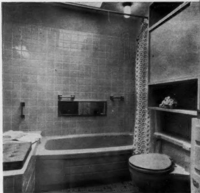
FALL-PROOF bath has extra grab bars, built-in seat close to tub, maximum shelf and storage space within easy reach. "How to" building details below show all four walls.
