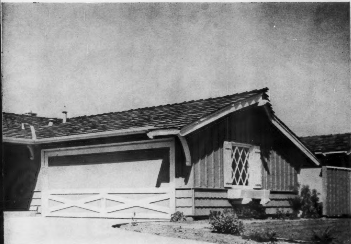
found in every room of its L-shaped plan. Credit is largely due to a careful selection of details, materials and finishes.
