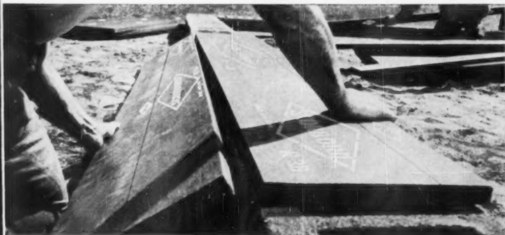
Scorbord snaps off at convenient pre-scored intervals, saves installation time and labor.
