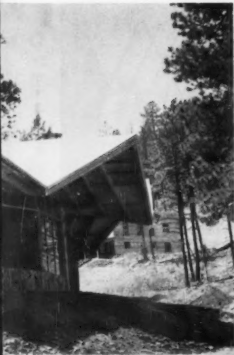
VALLEY CHORDS of plates are 2½x10s; chords at peaks, 3x6s; fascia boards at end of cantilever 4x8s. Pitch: 6-12. WHAT
