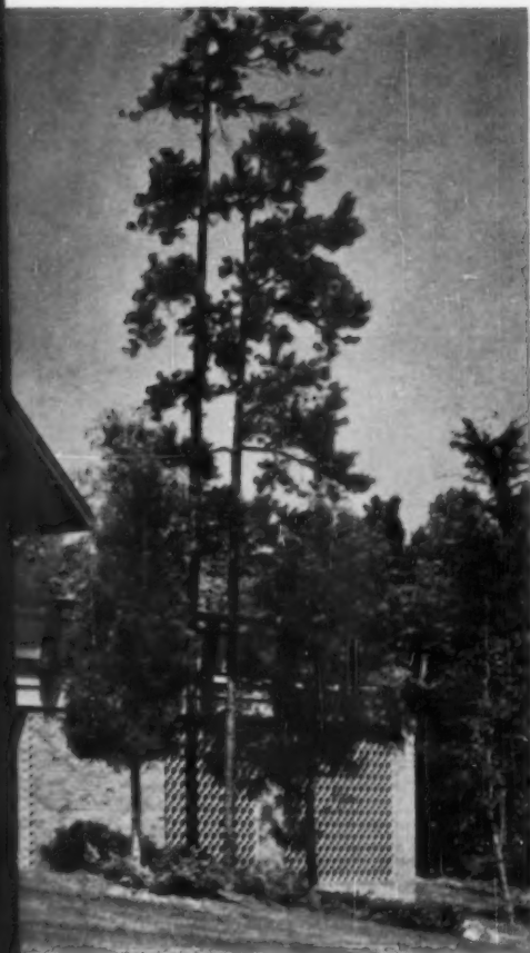
bricks in wall are offset at intervals.
