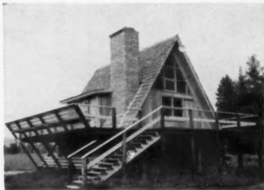
MULTIPLE WINDOW UNITS add style with function. Fireplace (regular model) uses 420 std. brick; 100 conc. blk.; 12-ga. metal flues.
