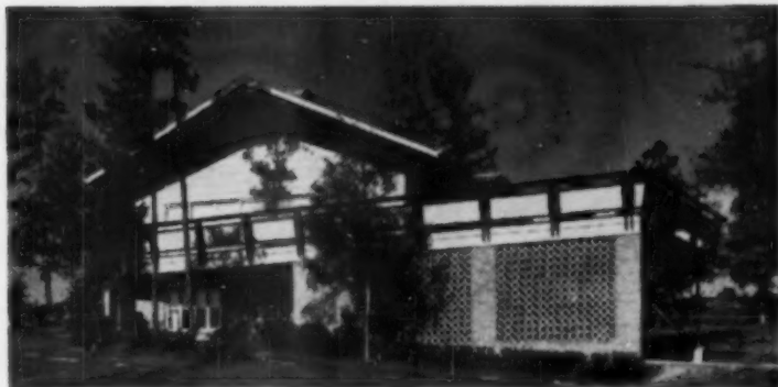
CLAY SOLAR SCREEN hides carport and assures terrace privacy at rear of two-level structure. Yard is equipped with hidden irrigation system. When water is on, pressure raises spray heads about 1½ in. for sprinkling.
