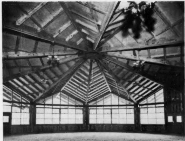
VALLEY CHORDS of plates are 2½x10s; chords at peaks, 3x6s; fascia boards at end of cantilever 4x8s. Pitch: 6-12. WHAT
