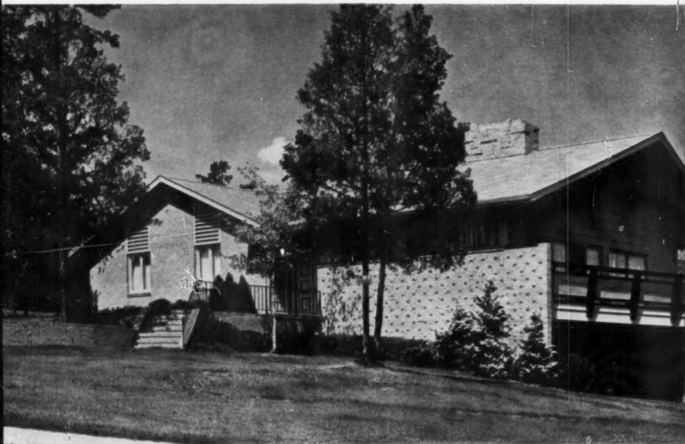
BRICK, CLAY UNITS , skillfully interwoven with wood, put Echo Home in luxury class without custom cost. For texture,
