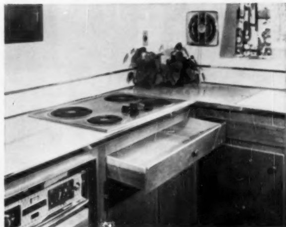
AN ELECTRIC RANGE with top-mounted controls leaves Schroeder enough space underneath to build in this handy utensil drawer. All Schroeder's cabinets are made for him locally.
