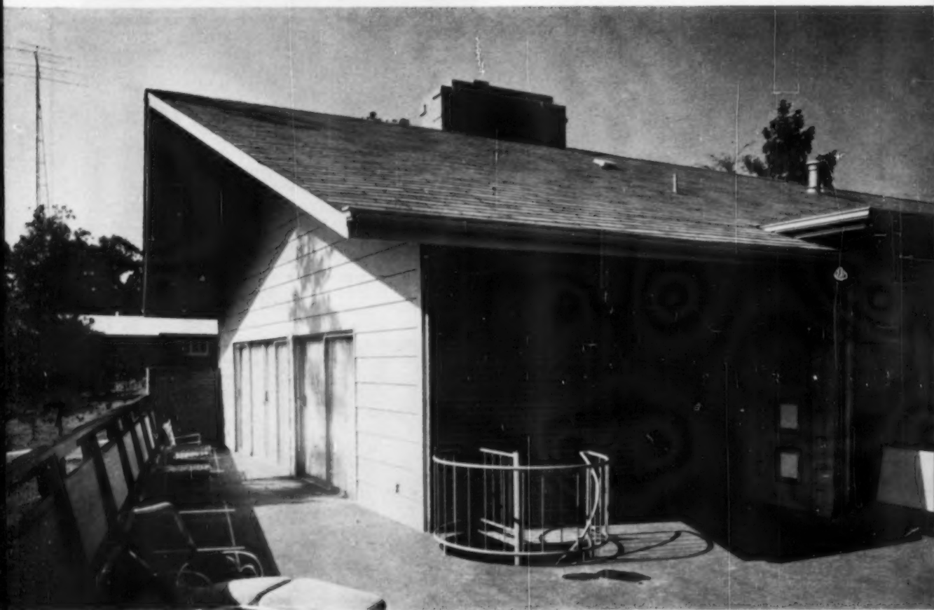
OPEN DECK TERRACE used for entertaining and as sundeck is big design feature. Spiral staircase leads to carport, living area below. Door opens to activity area.
