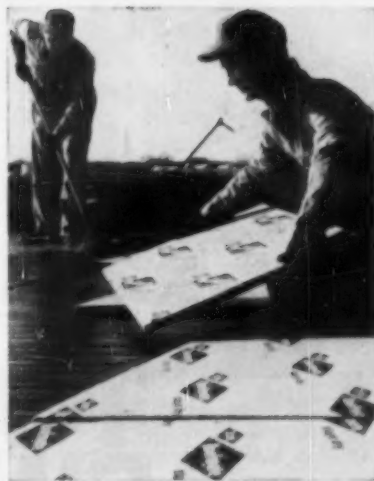
Roofmate provides permanently low "C" factor, high moisture resistance for built-up roofs.
