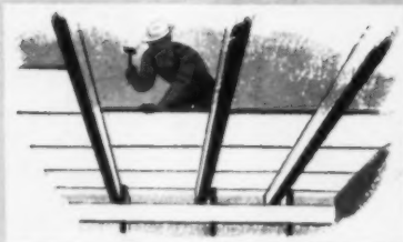
INSULATING ROOF SLABS. Roof deck, insulation, built-in vapor barrier, finished ceiling, plus continuous vapor seal at all joints. (Or without vapor seal and barrier.) Ideal for exposed-beam construction.
