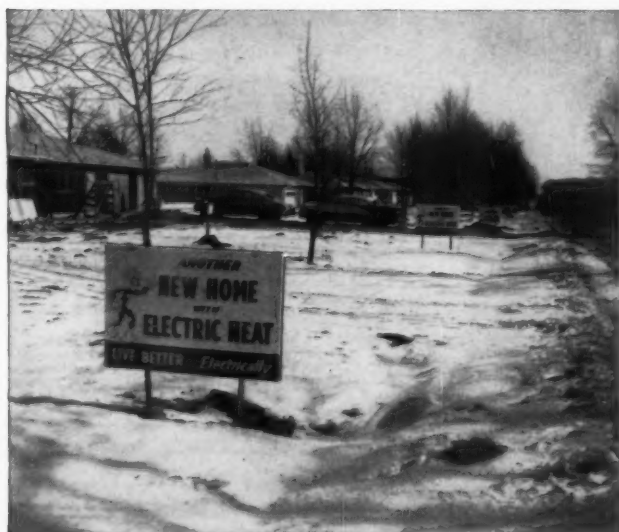
Medallion homes now under construction at the "Swanson Highlands" subdivision. Every home has its own sign featuring electrical living.
