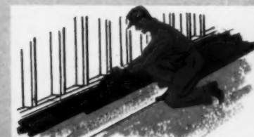
FLEXCELL* PERIMETER INSULATION. Asphalt impregnated throughout entire thickness of the board. For concrete slabs at grade. Like all Celotex Fiber Board products, effectively protected against dry rot and termites by exclusive Ferrox* process.
