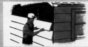
HARDBOARD SIDINGS. Beautiful, durable, easy to paint. Channel-Lap* siding applied with aluminum channels; factory primed; invisibly fastened; self-ventilating. Vert-Groove* panels offer modern vertical plank effect. Textbord* lap panel, or shingle siding; striated surface.
