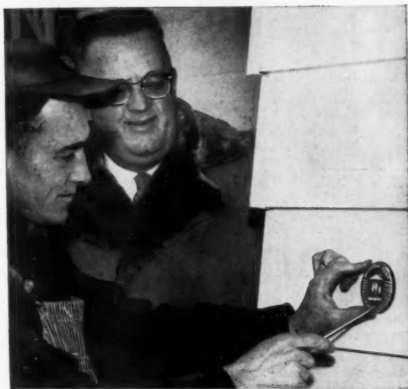
Live Better Electrically Medallion is installed on new home as builder Swanson looks on.
