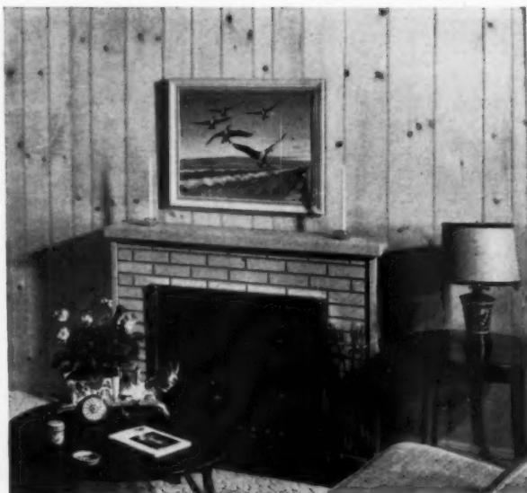
GRUVE-PLY: Idaho White Pine or Knotty Cedar plywood produced with surfaces carefully sliced like the most expensive imported woods. Looks like individual boards side by side. Goes up quickly, economically. Pre-grooved edges give uniform joints, eliminate need for mouldings.
