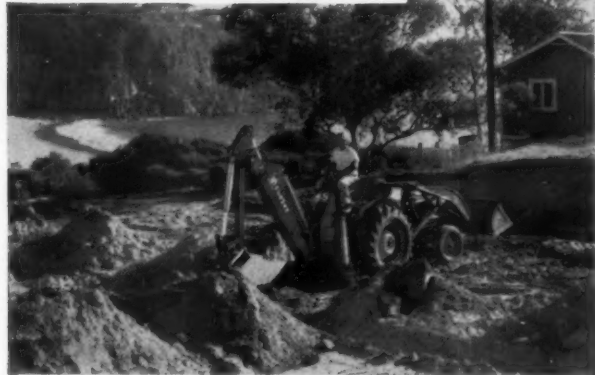
Mr. E. L. Shaner handles an "F" Sherman Power Digger for contractor E. A. Irish at a new subdivision in Laguna Beach, Calif. He says, "I have run them all and I like the Sherman best. It is easier handling. For instance, if I am sitting on a bank, I can swing up-hill—something you can't do with some of the other rigs. They just won't do it. And the Sherman has a full 90 degree swing both ways."
