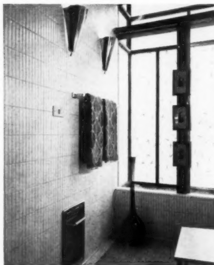
13 PLASTICS are all over the bath. In the Research House, laminated screening over the window (background) provides privacy, but also permits daylight to flood the room.
