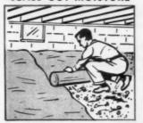
Warp's Polyethelene COVERALL permanently solves moisture vapor problems under houses. Prevents rotting of joists and sills. Also recommended for use between Studdings and Siding, and between Sheeting and Roefing material. COVERALL lasts a lifetime—is inexpensive, comes in various thicknesses and widths to 40 feet, for simple, easy installation.
