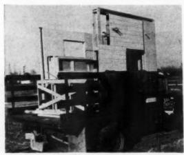
1 ENTIRE two-bathroom package is easily carried in a medium-sized truck. All fixtures are included.
