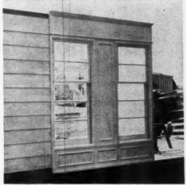
WINDOW PANELS start at 32" width, go up to any size in 16" multiples. "Homestead's" style carries window casing right to deck line, eliminates "lacing up" the horizontal siding at points where panels butt.
