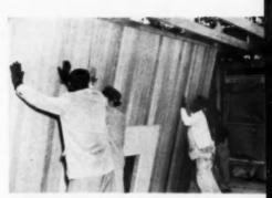
PREBUILT paneled wall with fireplace opening is set up in front of the shell and the furnace unit.
