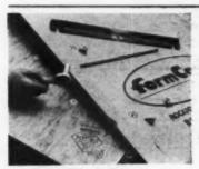
PLYWOOD FORMS are edgerouted for form tie insert.
