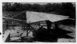
KEY ELEMENT in roof construction, Ledner says, is 1"x6" tongue-and-groove sheathing, which serves as structural skin for roof frame; helps make 42' span.
