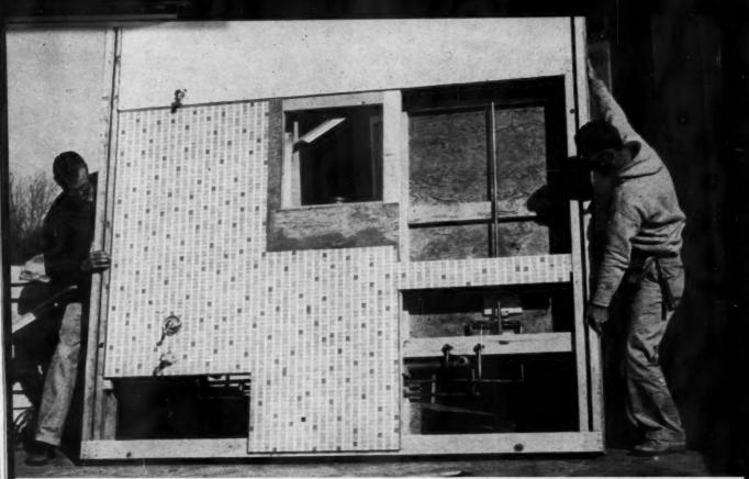
3 CORE of the bathroom package is this wall, which holds all the rough plumbing for two baths. Other
