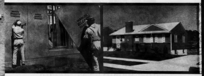
4'x 9' size avoids "piecing out," in vital sill area between foundation and sidewall. One man can easily lift, carry and nail a big, light 4' x 9' Bildrite panel. Applied, it makes a solid, tight, strong insulating shell from eave line to top of foundation.
