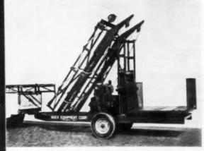
TO ERECT HOIST: turn on motor, throw out clutch. Hoistower is self-erecting and rises as wheels retract to its 45' unloading height.
