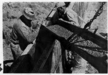
CONCRETE SURFACES stay smooth, rubbing and finishing time is cut because FormCo panels have no projections inside the forms. Clamps and ties are placed so concrete's pressure makes forms self-aligning and rigid.
