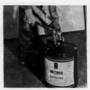
CAULKING-TYPE gun is loaded from 5-gal. can with an Alemite pump. Nozzle of gun is cut at 45 degrees. Angle determines position of gun while workman applies adhesive.
