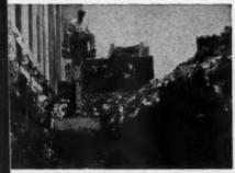
Digs flush when you need to — only the Model 210 Davis Backhoe has the ability to dig flush alongside walls, buildings, fences. Has 200° continuous operating arc.
