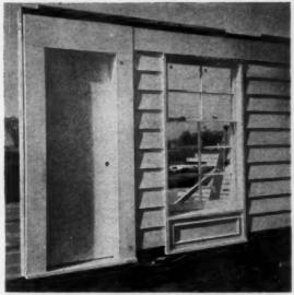
**DOOR PANELS** start at 48" width in the new Thyer system, get as big as 84" with double doors and big side lights. This rear door panel is 48"; front door panel on the "Homestead" is 64".
