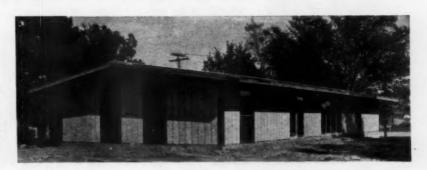
EXTRA THIN load-bearing walls of the test house make extra space available inside. Wallboard is nailed to 2x2 furring strips. Finished wall is only 5" thick, less than veneered wall.
