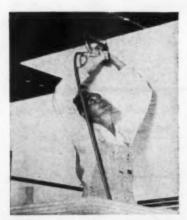
a hundred other materials are secured quickly, firmly with a power tacker. Here, a compressed air tacker, from Fastener Corp. (No. F54, p. 124).
