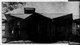
SUGGESTION of the Oriental is achieved by roof. Glass doors in center lead to dining room. Lapped 2"x10" siding, right, gives board and batten effect.
