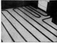
Install radiant panel or grid of steel pipe and connect with existing hot water heating system.
