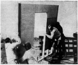
FRONT WALL is unloaded. Open area under tiling is where tub will fit; rest of panel is dry walled.
