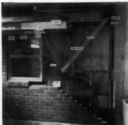
FROM OUTSIDE IN "Hidden Values" like insulation sheathing, trusses, window calking, extra paint are shown.
