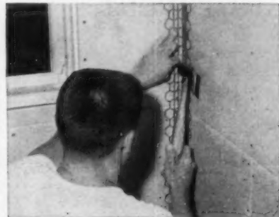
Keycorner is precision shaped to assure proper embedment in the plaster for maximum reinforcing value. It is easy to lap without interfering with plastering.
