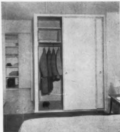
Here GLIDE-ALL Sliding Doors provide decorative panels for the generous storage areas in the bedrooms and halls of this apartment—one of hundreds in the Lake Meadows Multi-apartment project in Chicago. Architects: Skidmore Owings & Merrill. Contractors: Turner Construction Co.
