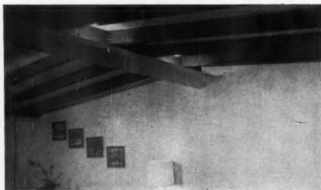
ATTRACTIVE incandescent lighting at ridge, lights living, dining area. 2x3's are used for non-bearing walls.
