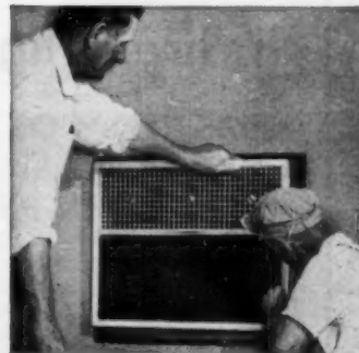
Slide the Thinline in later. Six screws make a strong and weather-tight seal.
