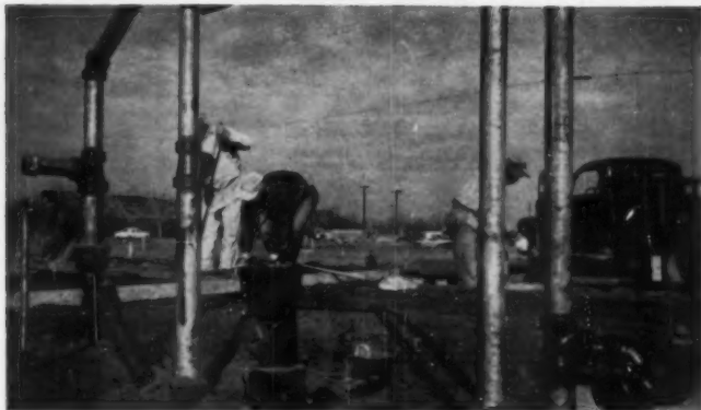
ROUGH-IN PLUMBING is completed before the slab is poured (left). Masons find light block easy to handle; King likes its low cost.
