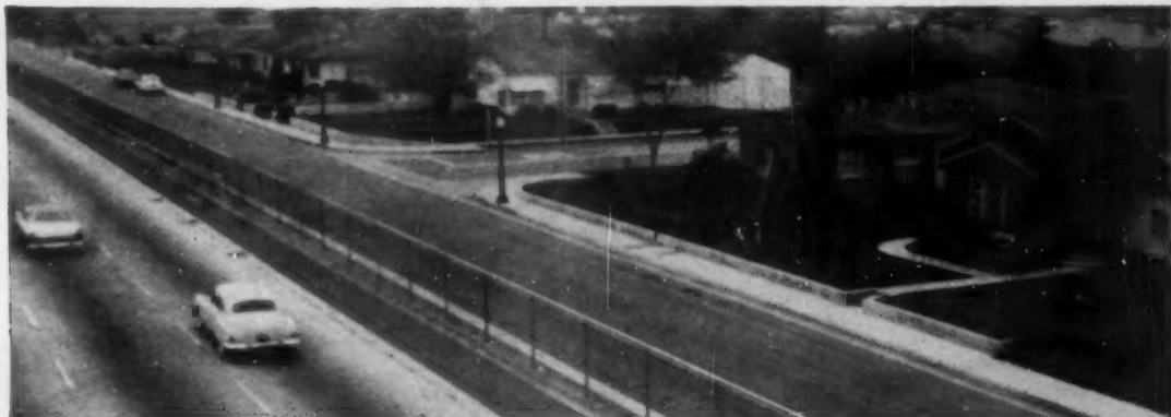
HOMES on frontage road alongside San Bernardino Freeway are separated from traffic by a chain-link fence.
