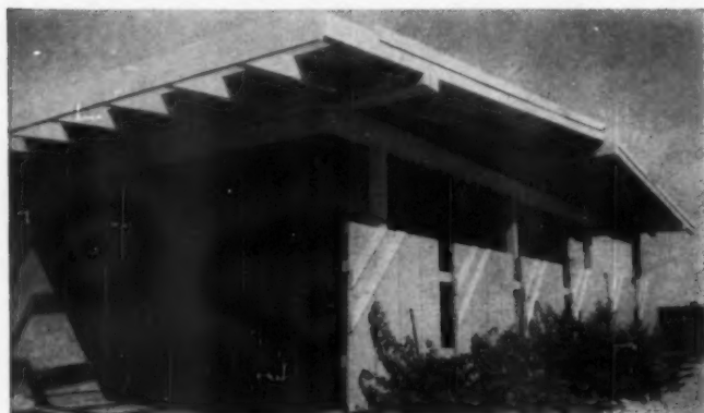
BEVELED 4x8" acts as bond beam, top plate and header for doors and sash. No heel cut in 3x6's is needed.
