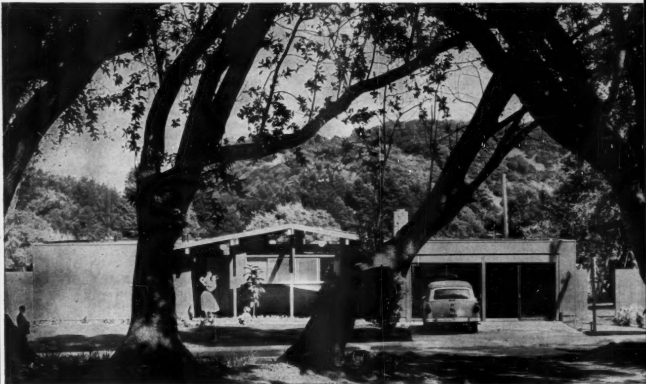
1 UNIQUE USE of sliding-glass doors on garage makes that space do double duty—as car-storage, or as an auxiliary playroom. House is also made to seem larger by extension of roof to form terraced entrance.
