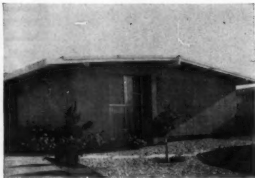
PROJECTION of sidewall, four-foot eave provides shade for the full-view floor-to-ceiling aluminum windows. Stacked bond is contrasted with typical-bond laid blocks.
