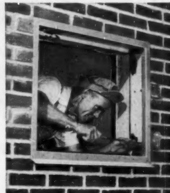
Leave an opening about 27 inches wide, 23 inches high to install General Electric Thinline through wall. Adapter kit makes it easy.
