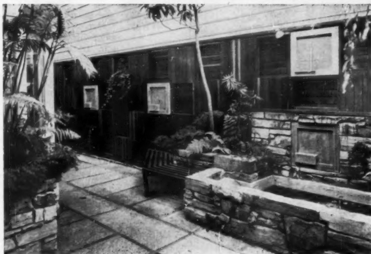
CHECKER PATTERN. Frame with short 2x4" girls toe-nailed to 2x4" posts. Cover squares alternately with short 1x4" V-edge siding (shiplap or T&G). Bruce Heiser, Architect.
