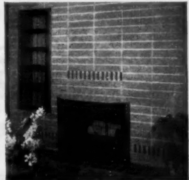
Stacked split units of any height make an eye-appealing fireplace. Shown are 4"x16" split block in stacked bond.
