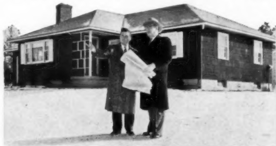
Here are Mr. Keddy and Mr. Vadnais at the site of a newly finished K-V Home. All K-V Homes are equipped with Crane plumbing and heating.
