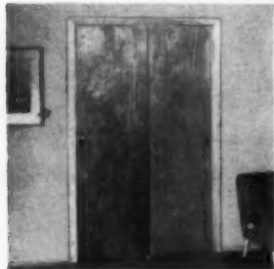
Adjustable Kenna-pak is nailed flush with side jambs
