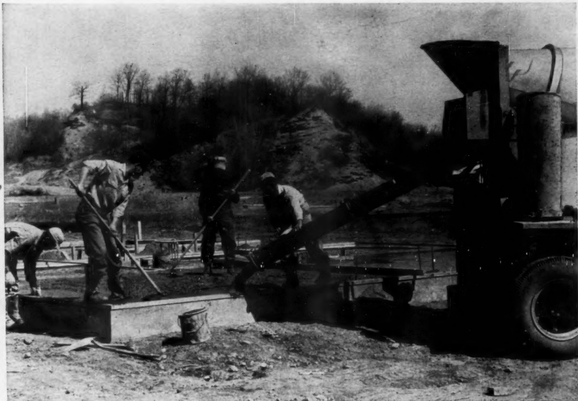
3. Next the slab is poured—and that's it! From experience National Homes finds it has protection from cold and damp for the lifetime of the house.
