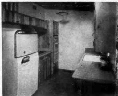
Only the finest of materials was used in these homes, including beautifully appointed kitchens and cast iron soil pipe from street to roof.
