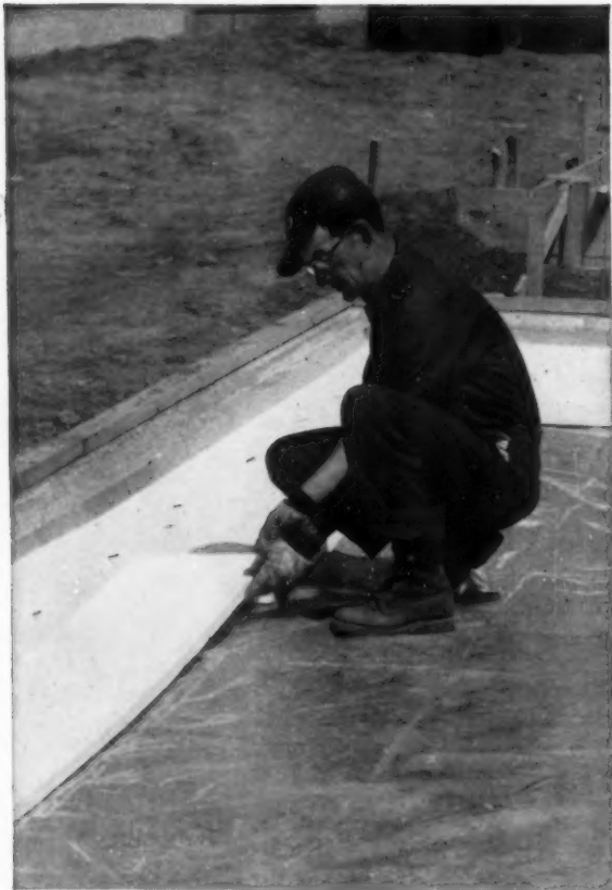
1. National Homes, Lafayette, Indiana, specifies Styrofoam 1" thick placed horizontally around the perimeter 12" from the foundation wall of the house.
