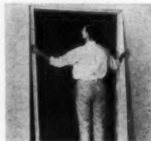
One man raises Kenna-pak and jambs into place
