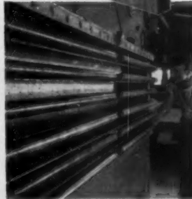
5 Accurate assembly is assured by controlled heat and pressure.
