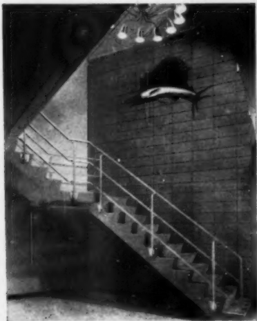
Horizontally stacked 8" x 8" x 16" units enhance the natural beauty of this "all block" office building.
