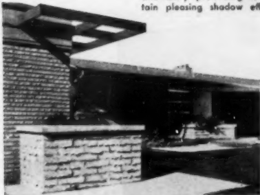
Concrete brick with extruded mortar joints and long low split units combined in this ranch type home.
