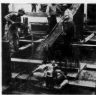
One-Man Electric Vibrator . . . It takes only one man to place concrete with powerful, Homelite high-cycle or universal electric concrete vibrators. Carryable Homelite generator provides power for high-cycle vi-brators and 110 volt DC for all universal vibrators, tools and floodlights.
