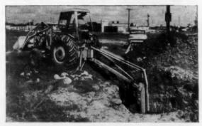
SHERMAN MAJOR DIGGER-LOADER COMBINATION performs a great many different jobs for the city of Dearborn, Michigan. The unit is used to dig water main taps and sewer sections, to install fire hydrants, to load and backfill and to do many miscellaneous jobs.
