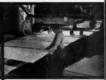
3 AT VENEER GRADING BELT, checks are made of both inner and outer plys for compliance with rigid industry and U.S. Commercial Standards.
