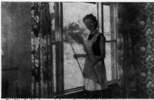
Double, double hung windows offer a full double sash plus screening in a slender aluminum frame. Factory assembled and glazed. All sash are self-storing and removable from inside for cleaning. Low cost . . . minimum maintenance . . . completely weather-stripped.
