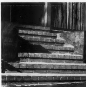
CONCRETE STEPS , shown above, were patterned, show versatility of tools.
