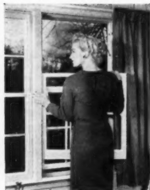
LIFT OUT —removable wood sash speed up installation—improve liveability.
