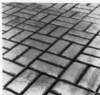
BRICK PATTERN after stamping. Tools penetrate to a depth of about 1 inch.
