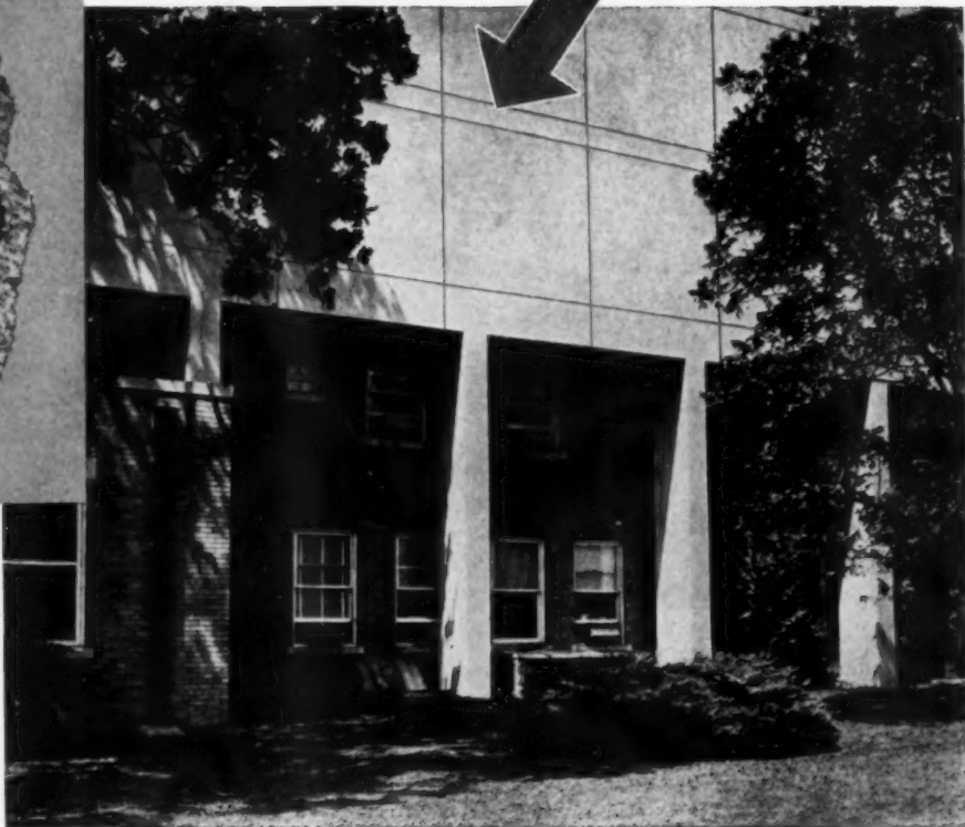
Photographs show how Dallas Medical and Surgical Hospital used Penmetal expansion joint to take care of cracking from expansion, and also to give a pleasing pattern to the stucco.
