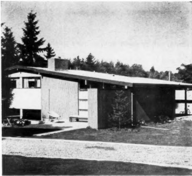
ALTERNATE REAR VIEW , with concrete terrace, can also serve as front of Vaughters' house. Here vertical siding and asbestos board are used. Fascia board extends 3" above roof, has cant strip to form gutter.
