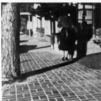
FINISHED brick pattern, shown above, has joints mortared for realism.
