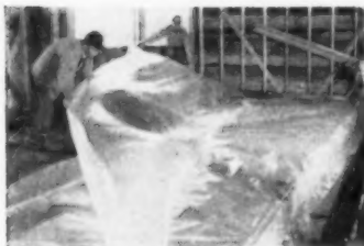
VISQUEEN film is best permanent moisture barrier under concrete slabs or floors. Wide widths and light weight mean low laying costs.
