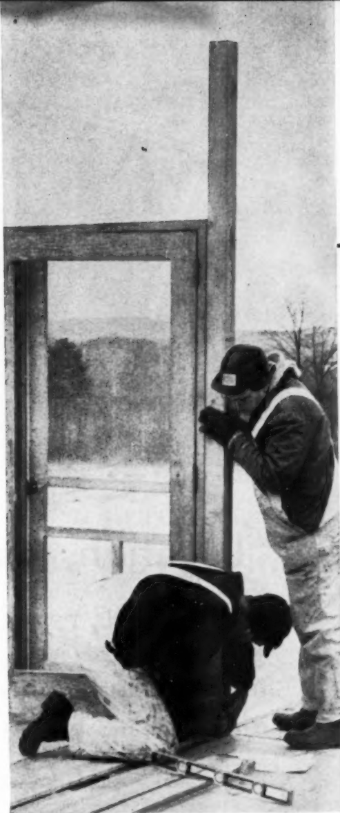
Techbuilt vacation house going up—see pages 98-99.
