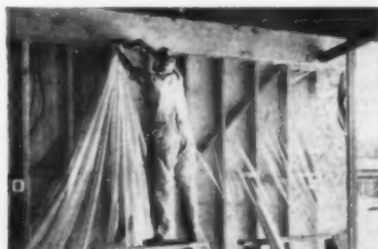
Use VISQUEEN film as a moisture vapor barrier to keep water out of stud walls. Eliminates paint peeling and prevents rot.
