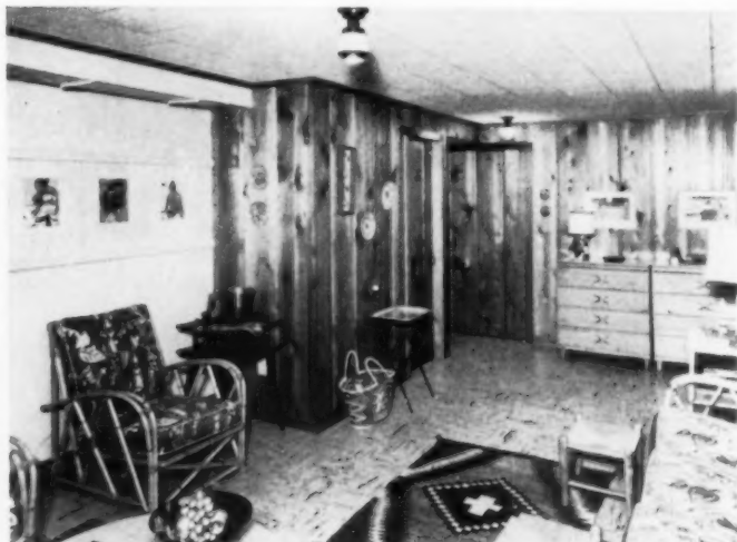
BASEMENT IS PANELED , was put in after house was built at added cost of $600. Area actually serves as a downstairs family room. Underwood believes in the best: #1 Douglas fir joists and rafters and #1 white fir studs in walls.
