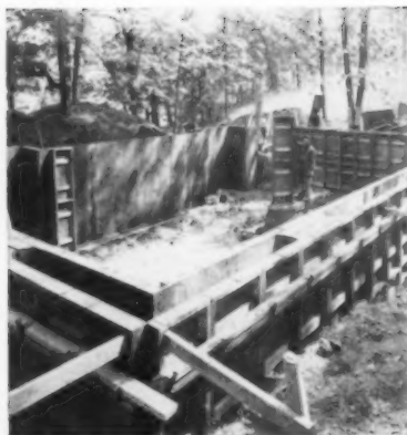
"CHAMP" Forms with cross members on 24" centers, being erected for house foundation in Skokie, Illinois. Contractor, Harding Bros., Northbrook, Illinois.
