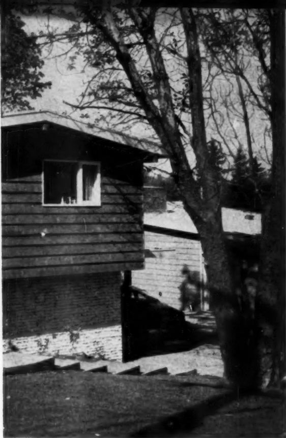
▲ TWO-LEVEL design has 1\frac{3}{4} " : 12 roof pitch, 3-ply Pabeo built-up roof with marble chip surfacing. Upper level of house stands 5 ft. above brick-walled lower level.
