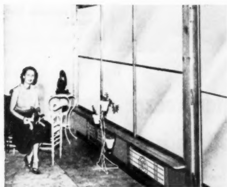
UNDER WINDOW WALL —Here a porch has been transformed into a glass-walled extra room. Twin heating units are placed under the glass window wall, occupying little usable space. Each radiant panel is complete unit in itself, eliminates need for running ducts or pipes
