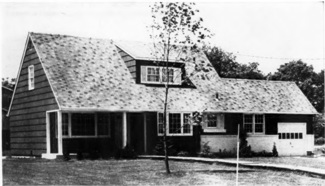
Space normally used as breezeway is utilized as dinette in front, covered porch in rear
