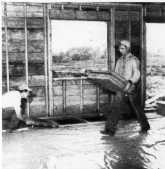
Perimeter insulation is individually wrapped in VISQUEEN film.
