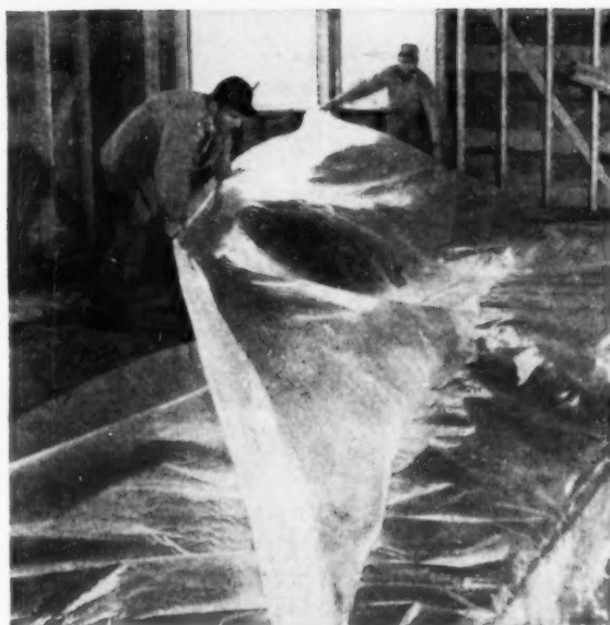
16 foot wide VISQUEEN drops into place with minimum of labor.
