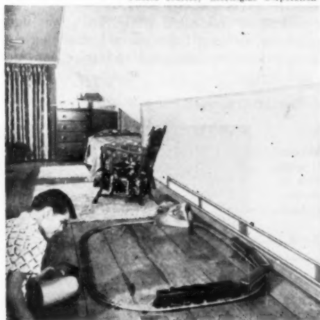
INSTALL IN BASEBOARD —Long, narrow unit is placed under low slope attic ceiling, provides radiant heat in areas otherwise hard to reach. Eliminates need for placing additional load on present heating plant. Units are controlled by wall mounted automatic thermostat
