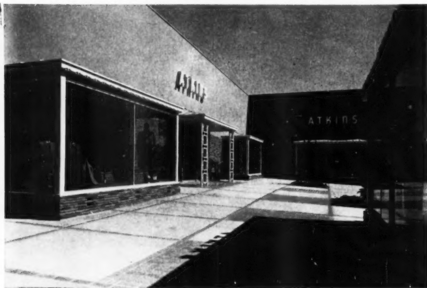
Exterior show windows create a dramatic effect—important for the display of merchandise. Island show window is seen at right, allows viewing on four sides
