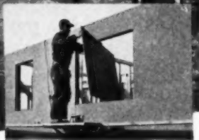
● King sizes mean one or two panels cover an entire wall area. Application time cut 50%. Window cut out after applying, pieces used elsewhere.
