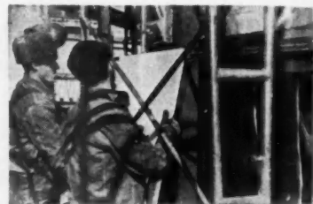
PORCELAIN ENAMEL PANELS were hung on "J" type 16 gauge galvanized furring
