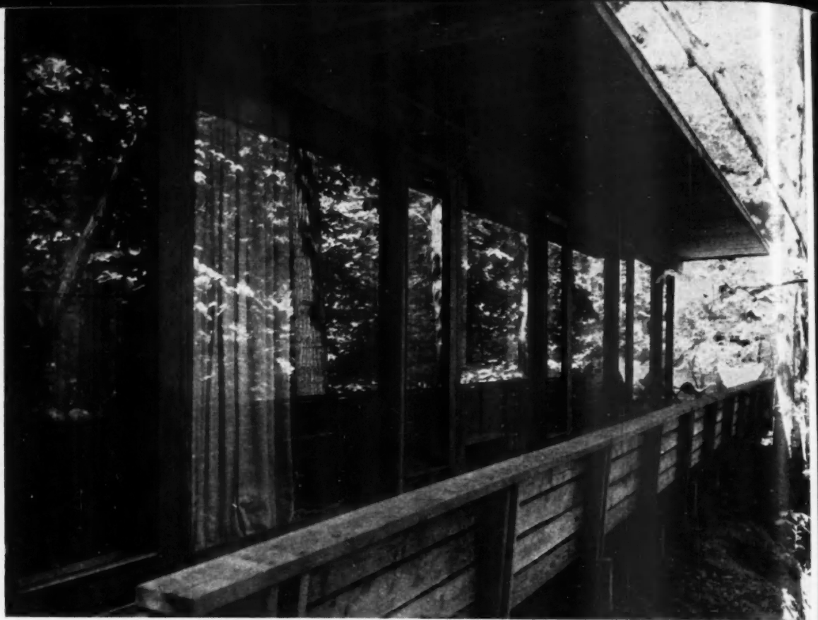
REAR WALL of house has a continuous assembly of glass panels and sliding doors placed between supports
