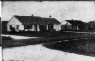
Robert Bartlett Bldg. Corp.
