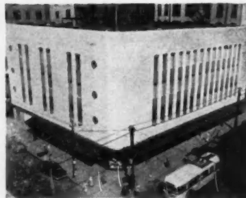
PORCELAIN PANELS give "1951 Look" to Denver apparel store, built in 1880
