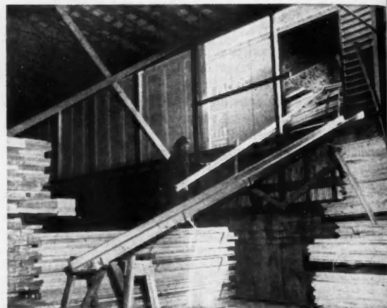
END LOADING from railroad car to pile lowers handling cost
