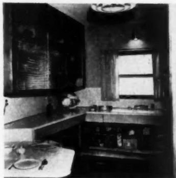
SLIDING ORNAMENTAL GLASS DOORS make it possible to see outlines of packages in cabinets
