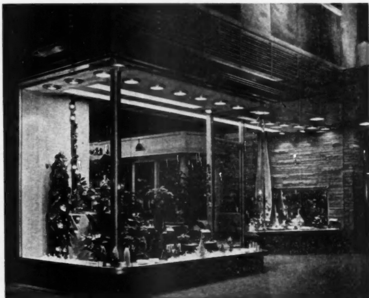
CANDY STORE —Notice how the "1-3-5-10 store lighting formula" is used in this 18 x 22-foot store with an 11-foot 6-inch ceiling. Four individual and one double 2-lamp 40-watt fluorescent recessed troffer units provide the "1" step of the formula in the circulation area. These units combined with another troffer of four units located next to the wall behind the counter provide the "3" step of the formula, providing 35 footcandles of general appraisal lighting. Nine 100-watt incandescent downlights contribute an additional 20 footcandles on the counter top. This local counter lighting, plus the fluorescent lamps inside the showcase provides the "5" step. Fluorescent-lighted wall displays are "10" step of formula
