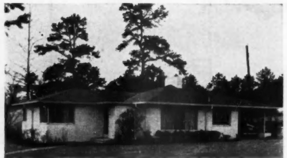
EXTERIOR SURFACE is concrete blocks, painted
