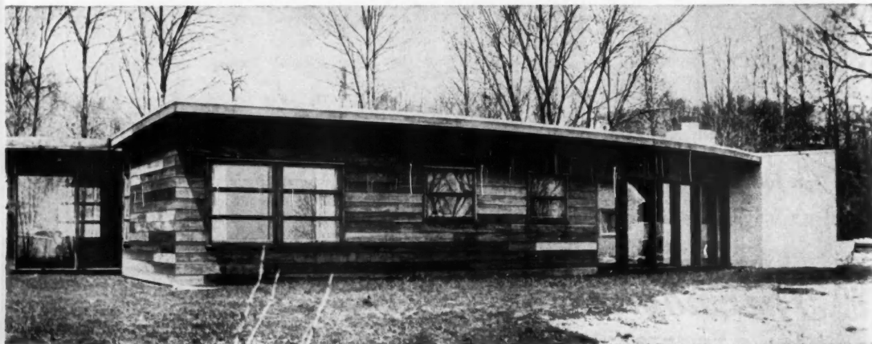
LONG CURVED OVERHANG in front ends at concrete block wall projection
