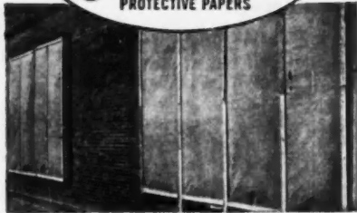
SISALKRAFT used for closing-in.
