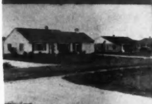
Robert Bartlett Bldg. Corp.
