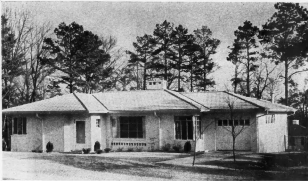
WALLS are white stucco over concrete block; roof surface is light colored asbestos shingles
