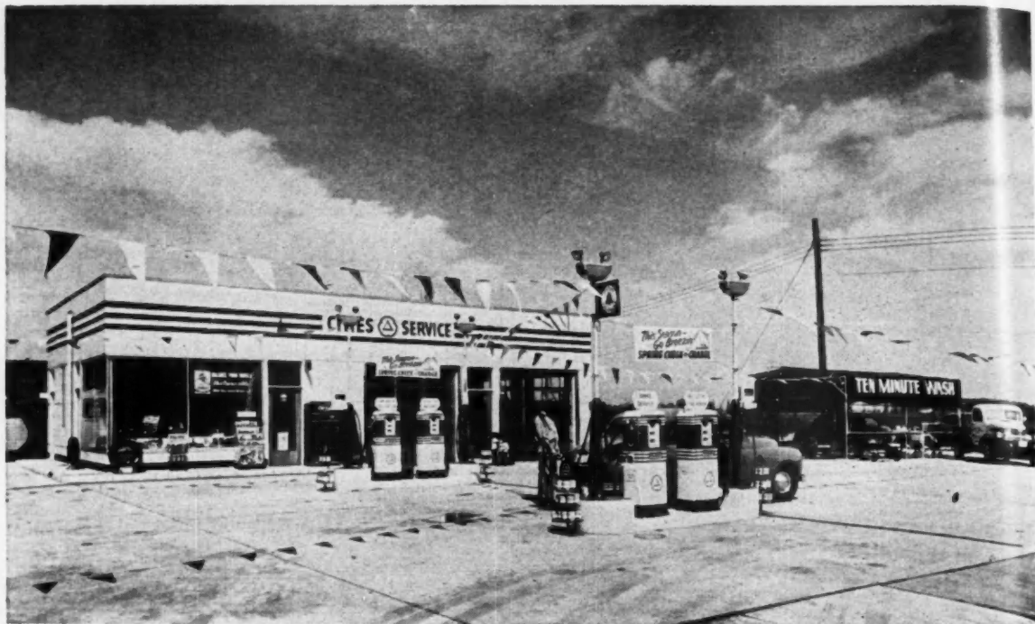
ASBESTOS-CEMENT wall panels and roof tile simplified construction of this Marion, Indiana service station
