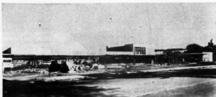
CONSTRUCTION view of two story unit at south end of project
