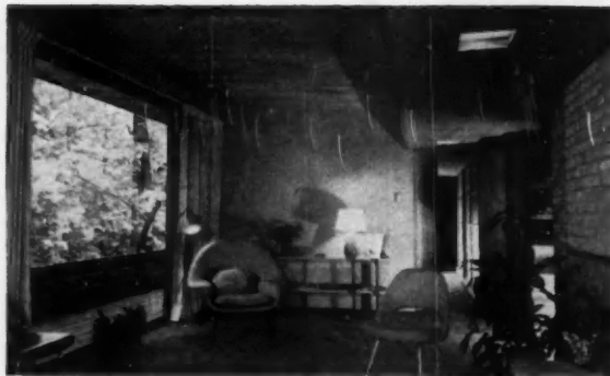
3-INCH MILLED roof boards form ceiling in living room
