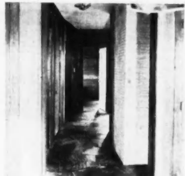
CURVED HALLWAY has walls of scored concrete block and redwood boards. The floor is Tennessee stone
