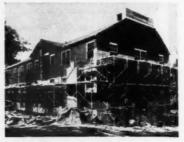
SECTIONAL steel scaffolding is used for apartment masonry work. Scaffolds illustrated in this article were made by Patent Scaffolding Co., Inc., Long Island City
