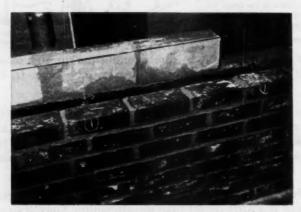
IN BUILDING this test wall the mason has taken the necessary precautions to smooth out the mortar squeezed out of the joints in the cavity
