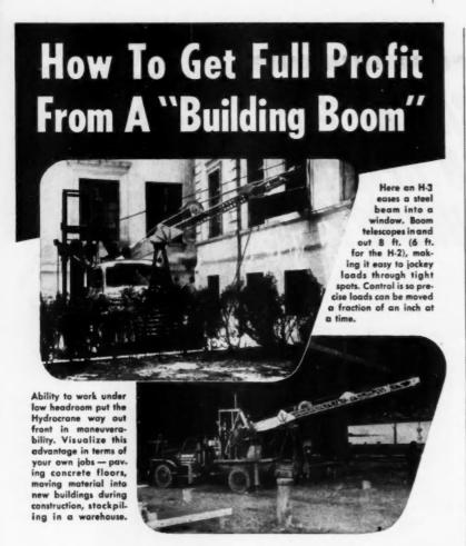
GET a boom that telescopes — hydraulically. That's the kind of boom the Bucyrus-Erie Hydrocrane gives you — and it's one of the biggest advantages ever built into a crane. This boom can nose in and out of windows and doors, between framework and overhead wires — without the crane moving an inch! And to make this an even greater advantage the Hydrocrane's boom is mounted high on the "A" frame for effective operation in horizontal position.
