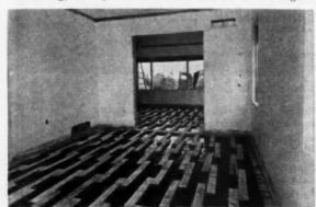
SIMPLIFIED METHOD: T & G strip hardwood flooring is applied to these staggered sleepers imbedded in mastic on slab
