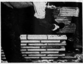
APPLYING asphalt paint to cavity face of interior wythe
