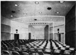
SEATING CAPACITY of auditorium is 300. Ceiling is lightweight acoustical plaster. ½-inch thick, for sound control
