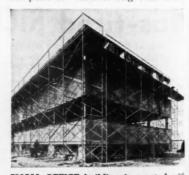
SMALL OFFICE building is erected with aid of prefabricated sectional scaffolding
