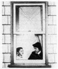
MADE of plastic laminate in three layers. the window opens automatically by folding about its edges when explosive pressure builds up. This action prevents the window from being blown into room
