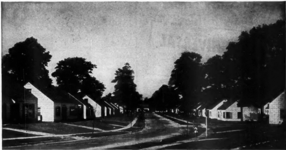
Street of new homes in Searhurst Subdivision, Cuyahoga Falls, Ohio. "Century" Siding Shingles used on all 166 homes in this project.
