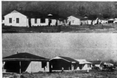
COMPLETED and unfinished homes of the 51-unit housing project
