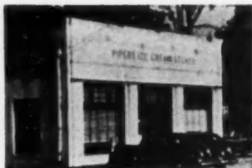
OLD BUILDING before remodeling
