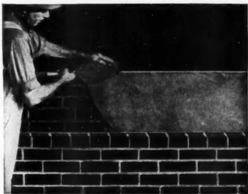
The face brick should be backplastered.
