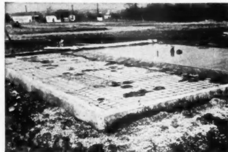
FOUNDATION has 12-inch walls and concrete slabs over slag
