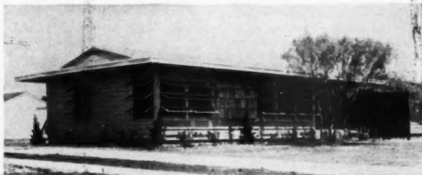
WIDE OVERHANG keeps sun from striking windows in summer. Price of house, $11,200
