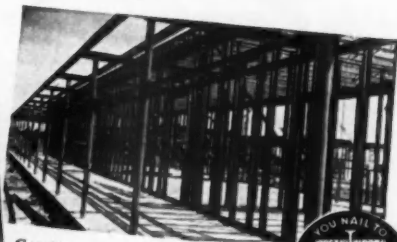
Corridor detail of school showing Stran-Steel framing.
