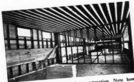
Interior view of school under construction. Note how wood collateral is nailed directly to metal framing.
