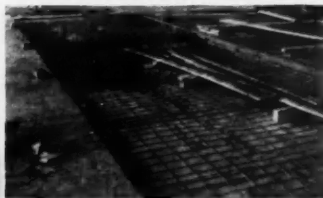
Big building, above, small home, below; SISALKRAFT covering subfill of both
