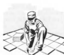
Nail over wood sub-floor or old wood floor
