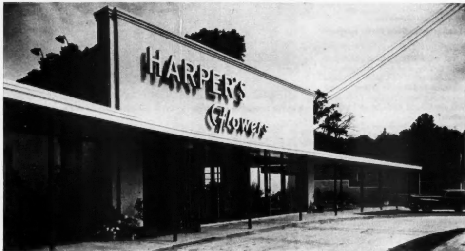
THE ADDITION of a curved canopy and remodeling of front wall completely changes the character of old building
