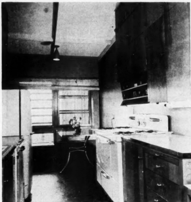
VENT HOOD over stove is built into cupboard. Condiment shelves are above. Construction details at right
