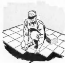
Install in mastic over concrete slab
