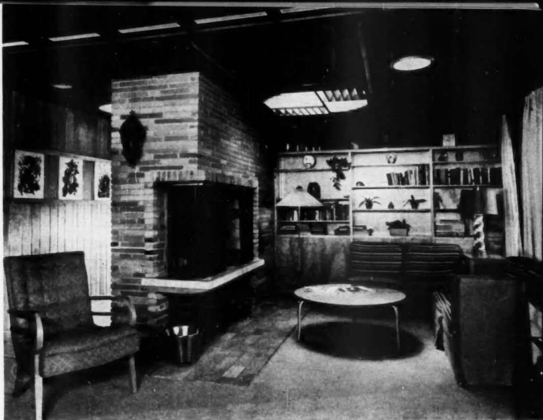
LIVING ROOM nook. Plexiglas blister in ceiling over front of fireplace provides a concentration of natural light
