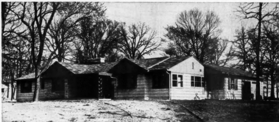
GABLES break low horizontal lines on front elevation. Without gables large expanse of roof would be monotonous
