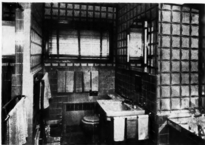
CLAY tile and washable wall paper simulating glass block make up the interior design of the bathroom. Window with venetian blinds is aluminum type with awning. Tub is at left in glass enclosure. The handle of built-in scale is near floor opposite lavatory
