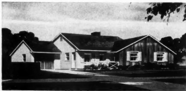
EXTERIOR SURFACE of stucco and wood presents a pleasing and varied appearance
