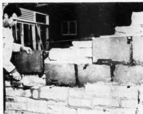
TYPICAL core wall construction with FOAMGLAS laid between outer and inner walls of cut stone
