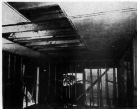
USKON panels are nailed, screwed on ceiling joists as are conventional wallboards
