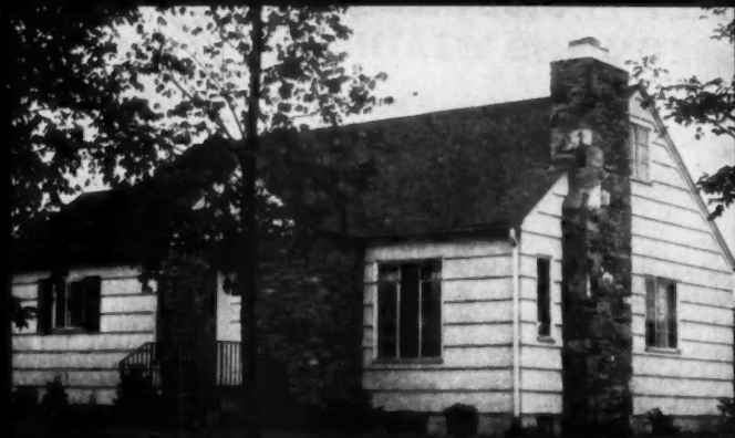
Residence of Paul B. Sullivan, Jamestown, N. Y. Axel H. Johnson, Contractor
