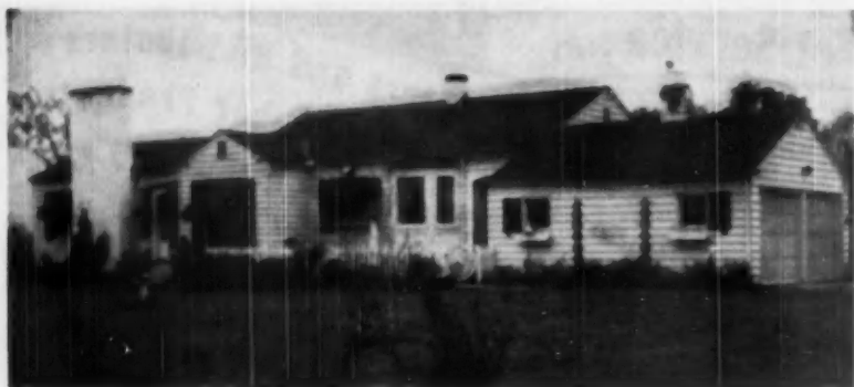
EARLY American charm of this home is represented both outside and in, and the builder-owner says it has served as a valuable advertisement of his work. Siding is Red Cedar.
