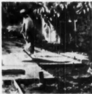
CONCRETE with vermiculite aggregate is used under regular concrete floor at ground levels to provide insulation. Wood sill prevents irregular temperature gradients. Felt checks moisture penetration.
