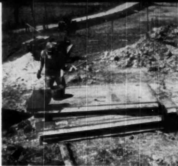
LEFT and above, workmen coat forms with oil to reduce water absorption
