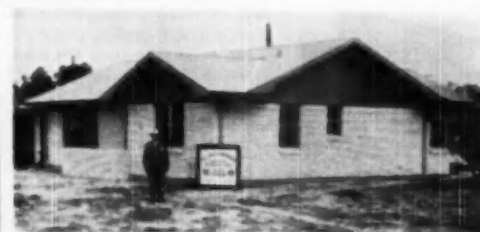
COMPLETED McClanahan home emerges from tent
