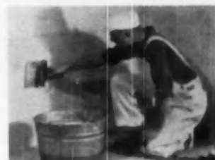
6. SECOND coat is painted on wall with whitewash brush while first coat is damp
