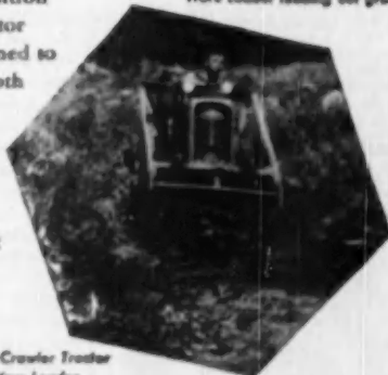
OLIVER Model "88" Wheel Tractor and Ware Loader loading out gravel.
