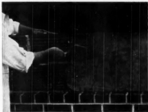
If the back-up units are laid first, the front of the back-up units should be plastered.
