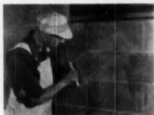
2. WALLS must be cleaned, scrubbed with a stiff brush, before they are painted
