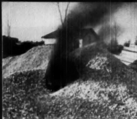
WORKING with concrete in cold weather demands special precautions, such as heating materials and covering fresh concrete in place as these two photographs illustrate
