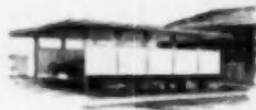
Idea for dressing up a porch. Exterior plywood applied horizontally to framing members of the porch to create weather and sight screen. Plan No. ES-20.
