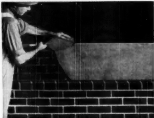
The face brick should be backplastered.
