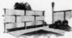
Woven plywood fence. Two-foot wide panels secured to alternating sides of posts with a "floating" spreader to give the woven effect. Plan No. ES-40.
