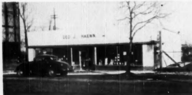
FRONT of the office and display room of the Haenn yard in Philadelphia. Because the bulk of business here is with builder-contractor customers, there are no elaborate displays in the showroom nor in the windows. There are fully adequate facilities here, however, in the form of office space and conference rooms for conferring with customers, servicing accounts
