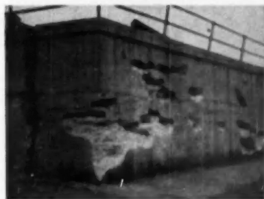
HOUSES in right column were constructed of pneumatically applied concrete. In lower right photo, workman are preparing walls for pneumatic application. Above are shown wall sections that are readily repaired by shooting concrete against the damaged surface
