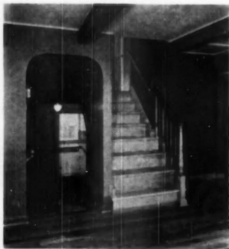
WALLS of stairwell and halls are covered with Sanitas
