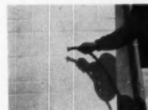
7. LIKE all cement products, cement paint must be cured, sprayed after application
