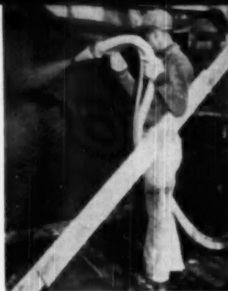
GUN for applying concrete is held at right angles to surface, as shown in top photos. Rebound collected at base is uncoated sand
