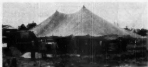
CONCRETE is placed with tent slope up in warm weather
