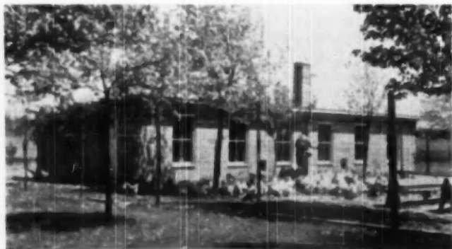
HEAT absorbing qualities of concrete recommend it for radiant-heated poultry houses
