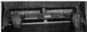
Measuring tread or riser
