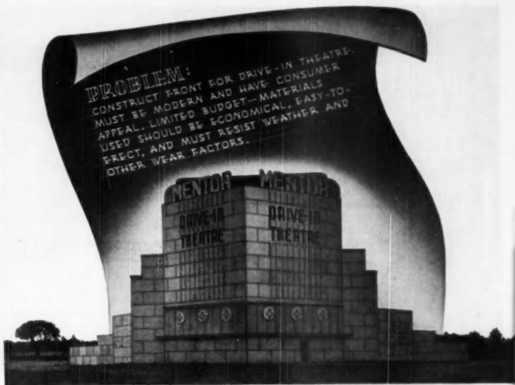
Decorative strip is K&M "Century" Asbestos-Cement Corrugated
