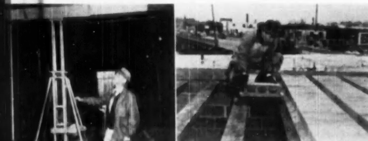
TELESCOPIC forms with jacks to facilitate installation and removal simplify the construction of floors with masonry floor filler block and eliminate need for form lumber. Blocks are aligned on spaced forms, preferably with staggered joints, after which reinforcing rods and radiant heating coils are placed before covering with concrete
