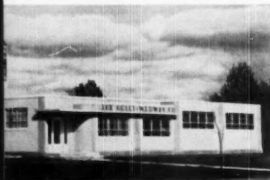
THIS small industrial building was constructed of tilt-up panels. Cast-in-place columns and beams bind the wall sections. A stiff cement mortar seals the base joint at floor level.
