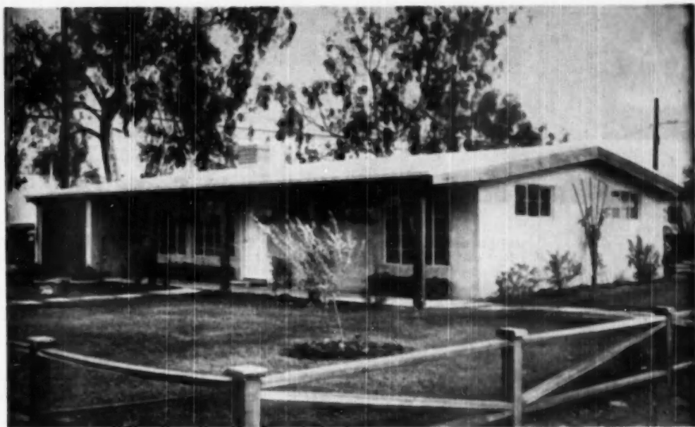
MODEL Gunite home built by Martin has a 5x38-foot porch, was completed in 15 days. Floor area is 1,002 square feet.
