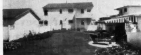
GROUP of three typical two-story duplexes in Westchester Plaza development. Outdoor living area, has good sales appeal.
