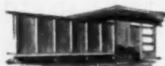
A "stepped" design with plywood. Vertical 2"x6" sections, cut from Exterior plywood panels, with 2"x6" dividers set at an angle. Plan No. ES-10.
