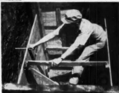
BELOW, earth can only infrequently be used as part of form. It must be solid
