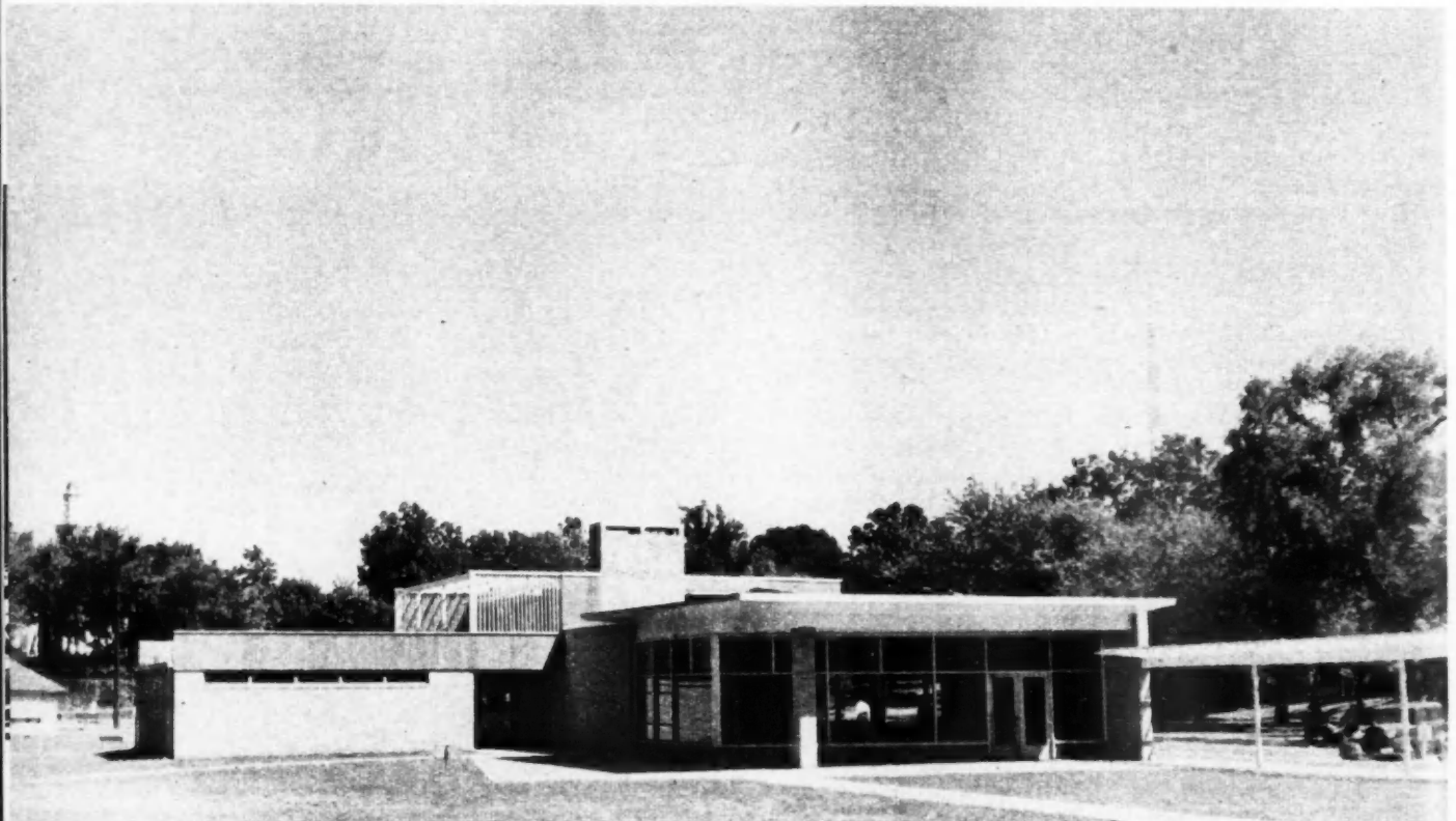
VIEW of building from park. Large lounge and terrace overlook the playing area. Feature is extended trellis at right of building.
