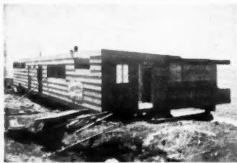
3rd Day 4 men—3 days—Ready for Plates and Roof
