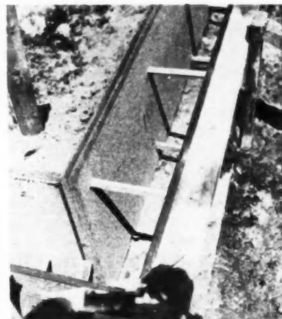
FORMS for the footings are gypsum board on the outside edge and 25/32 inch Insulite Bildrite sheathing on the inside as shown at right. Concrete is poured to ground level. Insulating wall sheathing on house below offers both structural strength and insulation in one package
