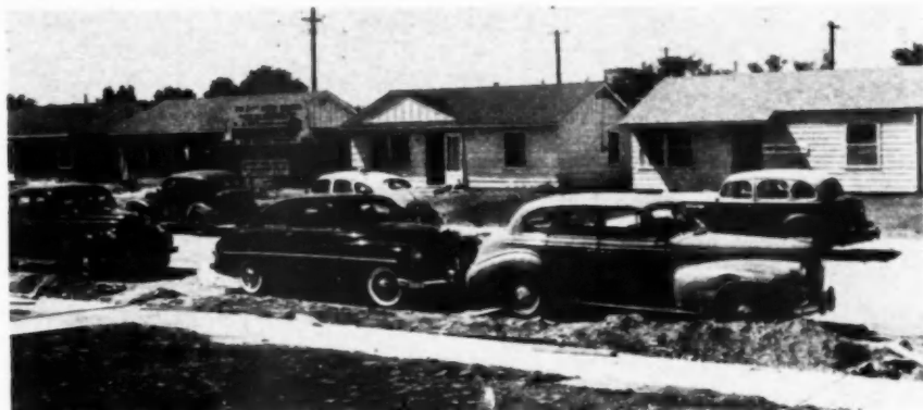
WHEN the project began the interiors of three houses were left unfinished. These are used as cutting shed, for assembly of prefabricated parts and for storing paint
