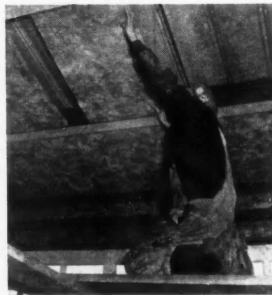
ROOF insulation was fitted between wood strips fastened to the roof beams
