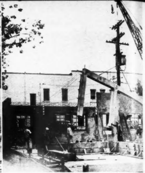
LIFTING precast rigid bent into place in wall.
