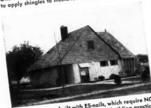
One of the houses in the development, using ES-nails to apply shingles to insulation sheathing.
