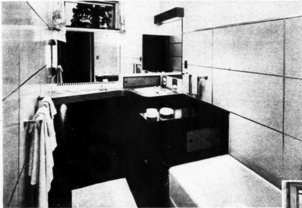
BATHROOM before and after remodeling. Formica has been used for walls, lavatory and dressing table, bulkhead cabinet, light fixtures, door and window trim. Plan below shows details of the remodeling job
