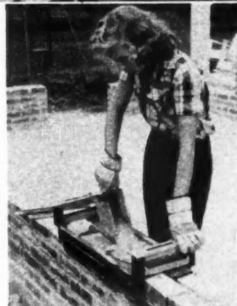
NEW bricklayer is placed at a starting corner on foundation base. A large scoop supplies enough mortar with one operation to bed eight to 12 bricks. Guides and the side walls assure plumb lining, and spirit levels, sides and ends, keep constant check. Arrangements have been made to mass-produce the machine
