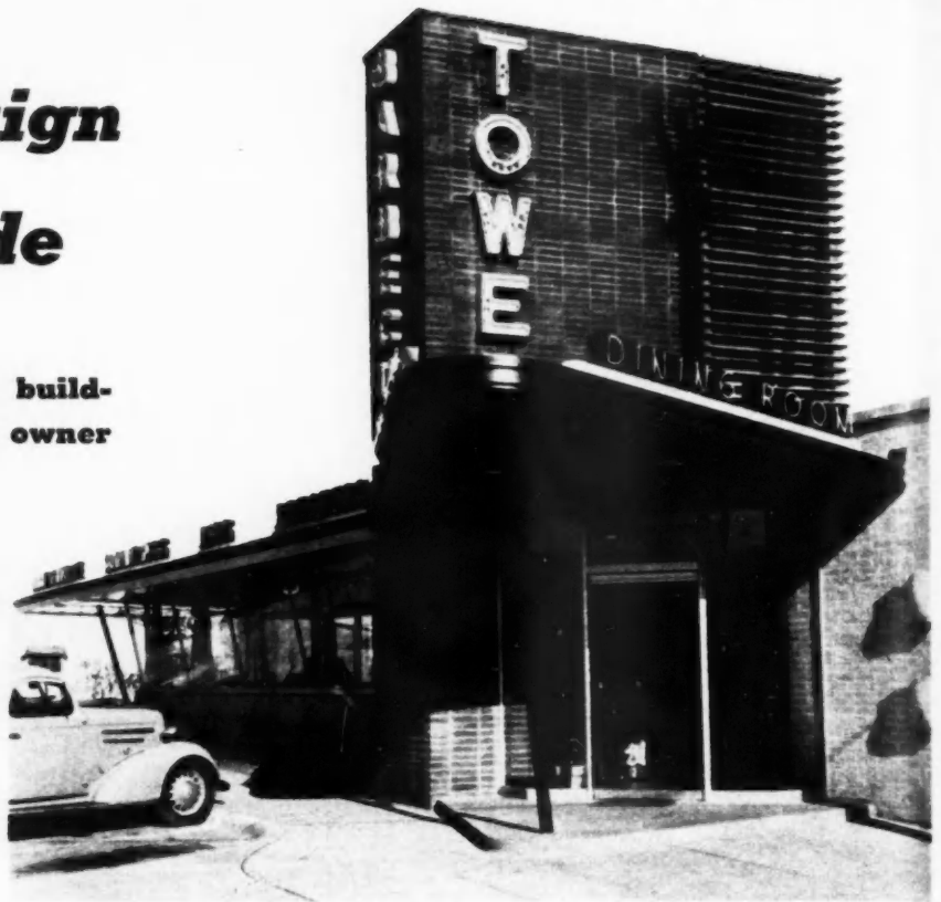
TOWER originally planned for forced draft unit serves only for display purposes
