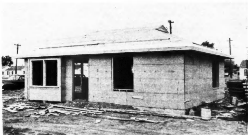
FORMS for the footings are gypsum board on the outside edge and 25/32 inch Insulite Bildrite sheathing on the inside as shown at right. Concrete is poured to ground level. Insulating wall sheathing on house below offers both structural strength and insulation in one package
