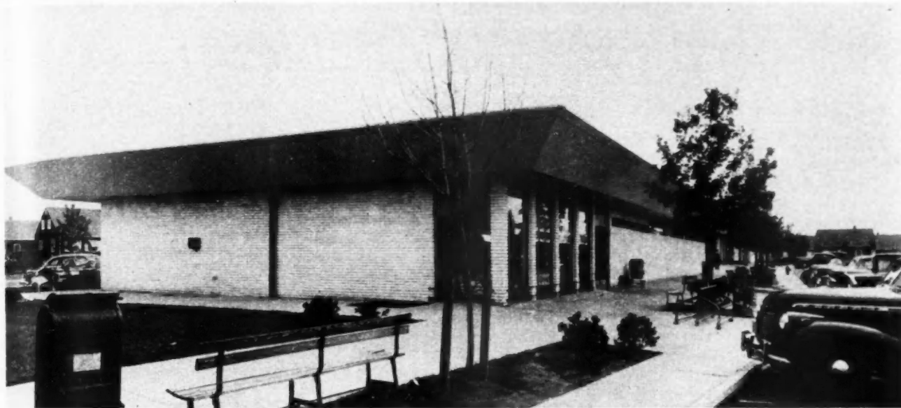
THE seven-foot overhang on these store building units eliminates the need for awnings and protects customers from weather
