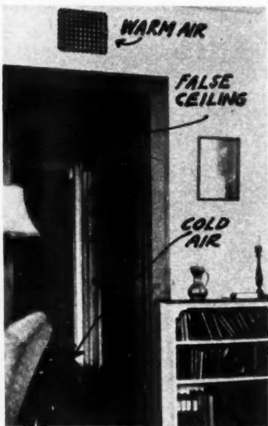
THE basementless house shown on this page was built 23 years ago by V. L. Sherman. Utility room floor is 20 inches below house floor. With warm air furnace placed next to chimney, cold air returns from three cold air faces are brought along under hall and connected to furnace. Except for warm air register to living room, all registers are fed from plenum chamber over false ceiling in hall, permitting warm air to come out above doorways—a hall-plenum system used in some construction today
