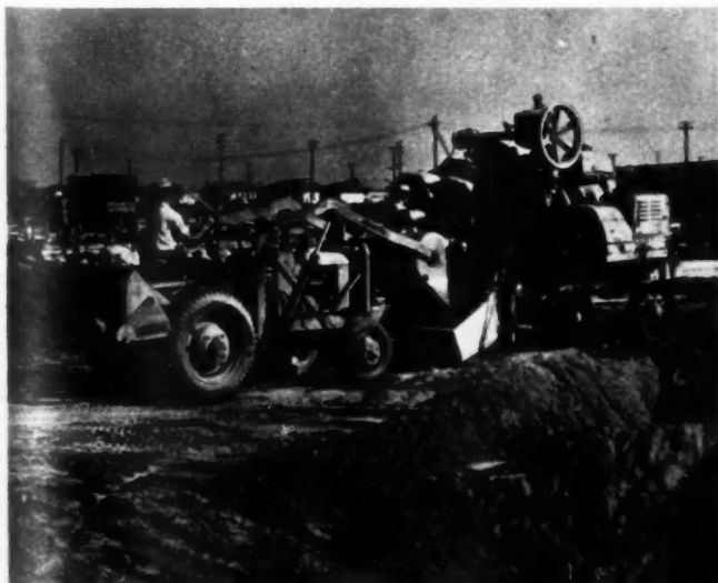
CONCRETE mixer is fed by skip-loader, left; enough rough lumber for a complete house arrives at building site on one truck
