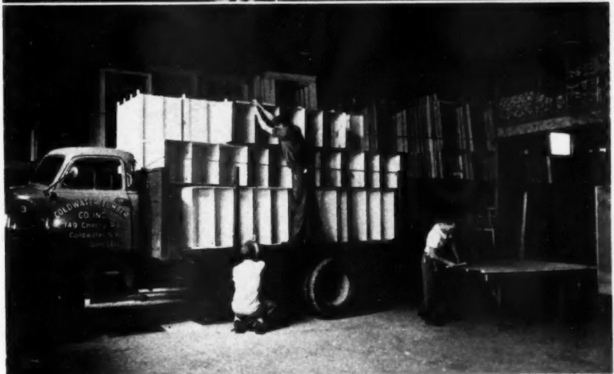
TRUCKLOAD of stairs, linen closets and wardrobe closets is prepared for delivery to project. These materials are partly assembled, and will be completely assembled and stored until needed at the project
