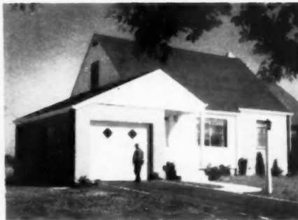
Approximately 20% of the 600 homes are completed with owners moving in as quickly as units are ready for occupancy.
