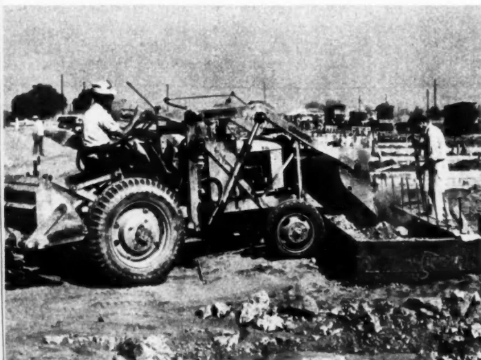
SKIP-LOADER is used for putting fill into area for porches. Sled facilitates fast loading and delivery of form lumber
