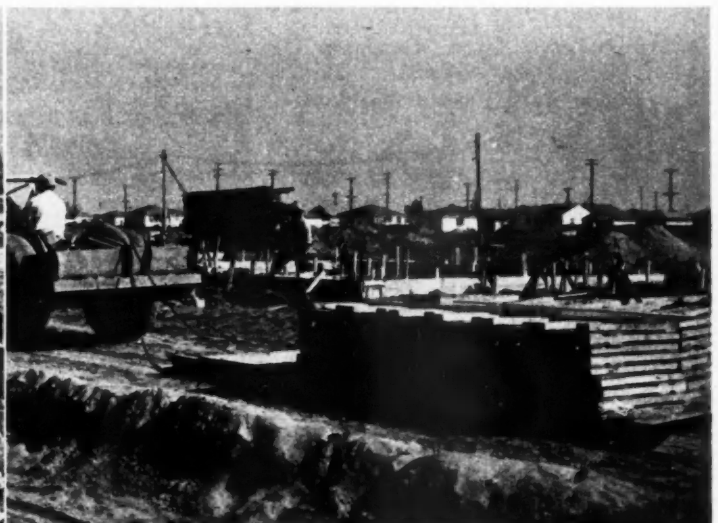
SKIP-LOADER is used for putting fill into area for porches. Sled facilitates fast loading and delivery of form lumber
