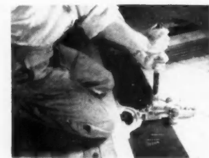
Flooring is held in place by ratchet catch. Both hands free for nailing.
