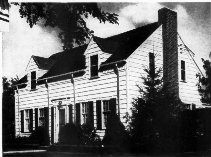
DOWNSPOUTS: Roof drains that will last forever—that's the dream stainless steel makes come true. The downspouts pictured here have been up 10 years.
