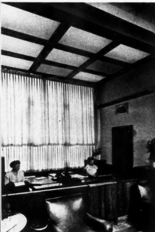
OVERHEAD panels add to daylighting
