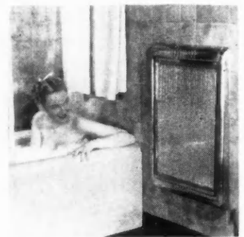
APPLICATION of Radiant Glass panels is illustrated in this bathroom
