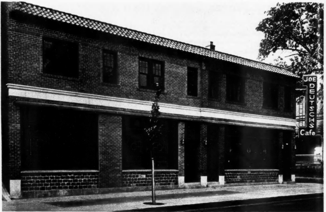
THE UNITY of design belies the fact that two decades elapsed between erection of original building and its annex
