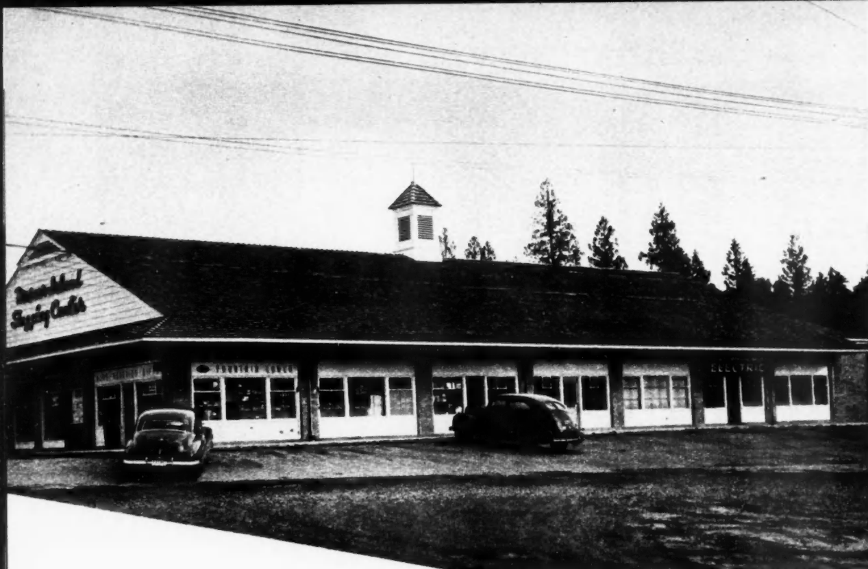
ONE side of Shopping Center, with only one window, may later be easily expanded
