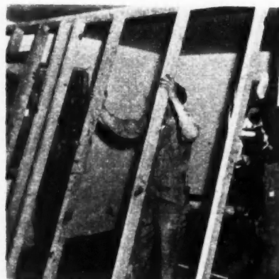
TIPPING a partition into place
