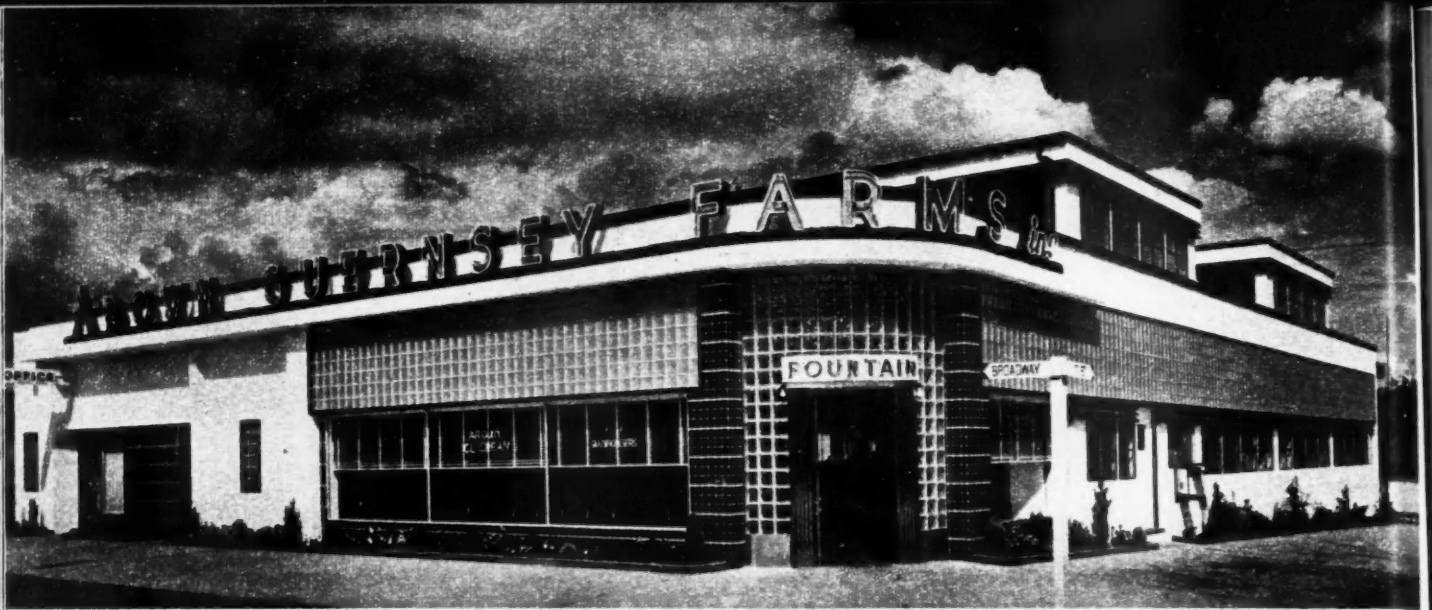
APPLICATION of various types of glass, glazed tiles, and white stucco causes the exterior to sparkle with cleanliness
