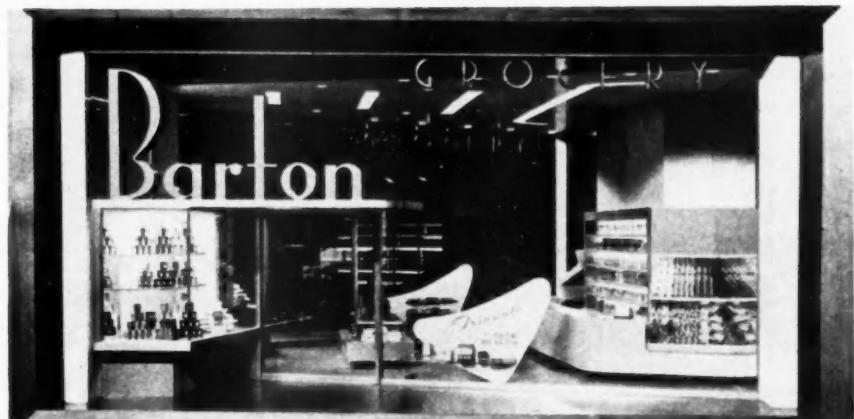
A SMALL FEATURE display window to the left of the entrance has been incorporated in the grocery store front shown here. A large visual area behind which a display unit can be placed is also one of the features. Name is in free-standing letters
