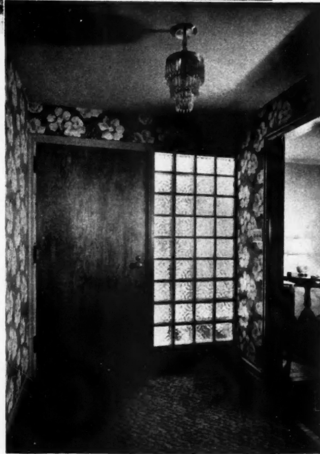
ROOF OVERHANG permits freedom in fenestration, such as application of large glass block area at front door
