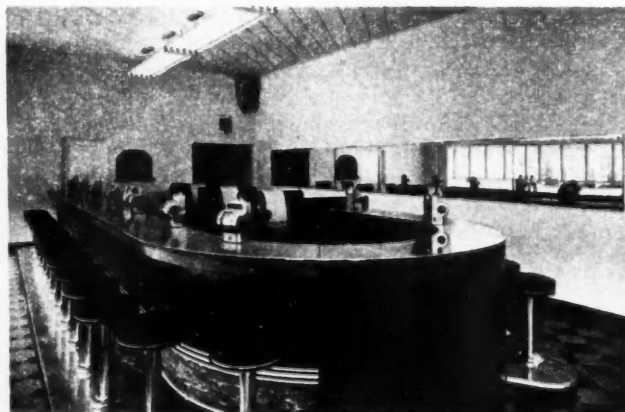
INTERIOR of fountain lunch room with large counter for service
