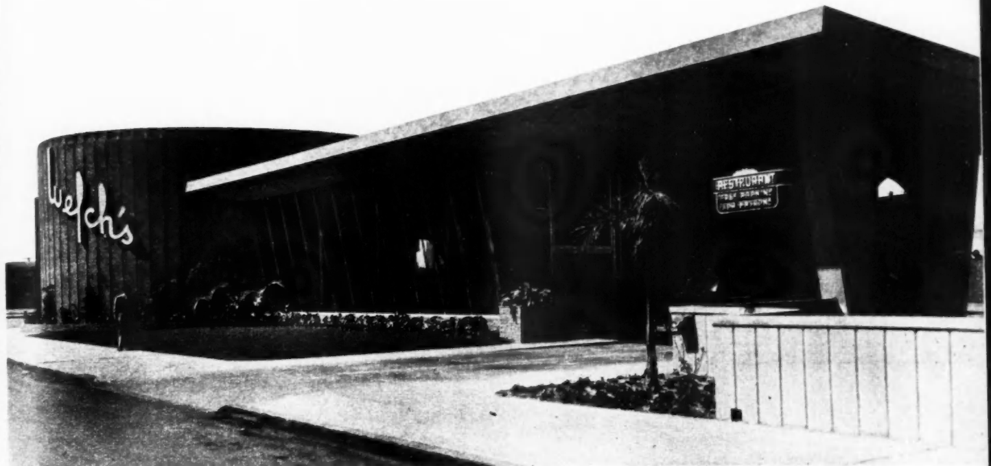
THIS restaurant, designed by the owner, is a good example of what can be done by careful planning and application of materials
