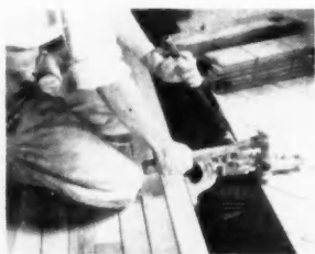
Armstrong Lumber Jack in position on subflooring. Simple attachments make it readily used on joists.
