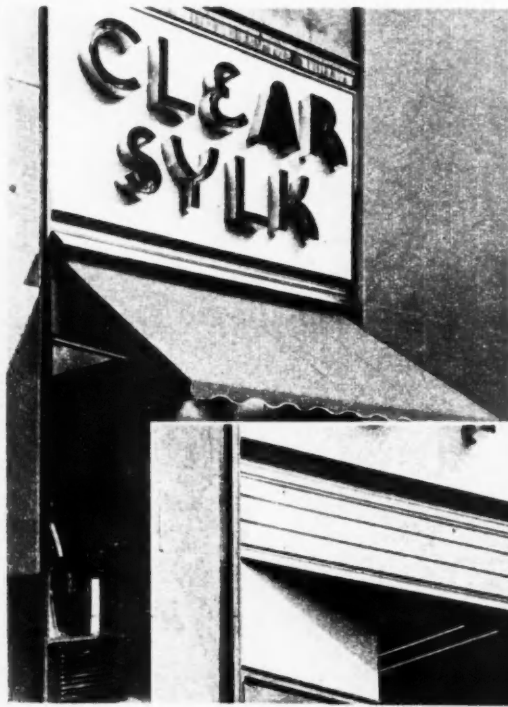
EXTENDED tension arms, maintain tautness of fabric and neat appearance in awning of store above. Arms fold back into recess box as they retract canvas awning
