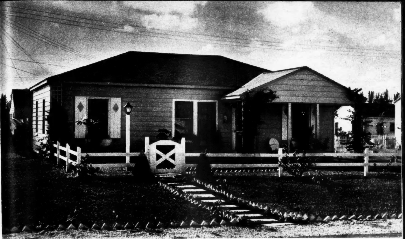
A COMPLETED Essex Village home, one of the 600 being constructed in Hialeah, a suburb of Miami, Fla.
