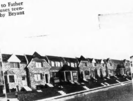
GREENWOOD GARDENS is a Philadelphia row house development, one of several similar projects in the West Oak Lane section of the city that uses a total of over 2,000 Bryant Model GF-56 Gravity Warm Air Furnaces.
