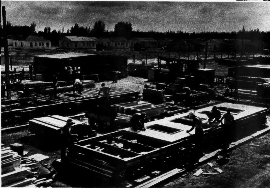
CARPENTERS in Essex Village assembly yard complete a wall or "panel," using pre-cut timber which is quickly fitted into place. Other assembly work is also being carried on in the yard. Completed homes are in background. Typical plan of two- and three-bedroom houses shown below. Variations in layout are made on basic plans
