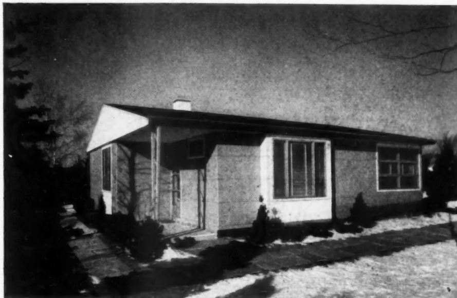
Permanent, easy to maintain, extremely little depreciation—these advantages are basic in the low-cost Lustron Home. Porcelain enameled steel panels can never decay, fade, weather or stain.
