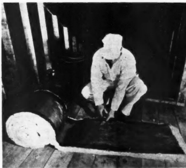
9. TO INSTALL cotton insulation, the workman needs a stapler, a heavy pair of shears, and a step-ladder
