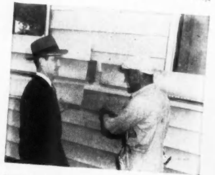
BUTT JOINTS held with back-up plates
