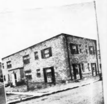
PERSONALIZED HEATING means radiation heating, too! Above is ARNA Valley, Arlington, Va., where more than 600 suites in 8-family buildings are individually heated by Bryant Model 26 boilers.
