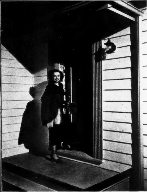
FLUTED architrave member frames the door, enhances attractiveness of entrance, adds Cape Cod touch. Knocker embellishes door
