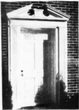
Here is a splendid example of the type of doorway often seen on Pennsylvania Colonial homes. It is suitable for houses of any structural material. Design C-1733.
