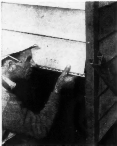
CORNER flashing gives water tight joint
