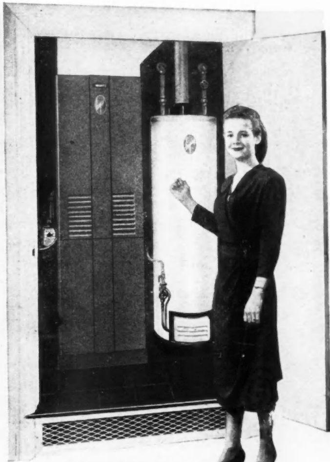
Photograph of an actual Bryant Personalized Heating installation, showing winter air conditioner and water heater installed in a small closet.
