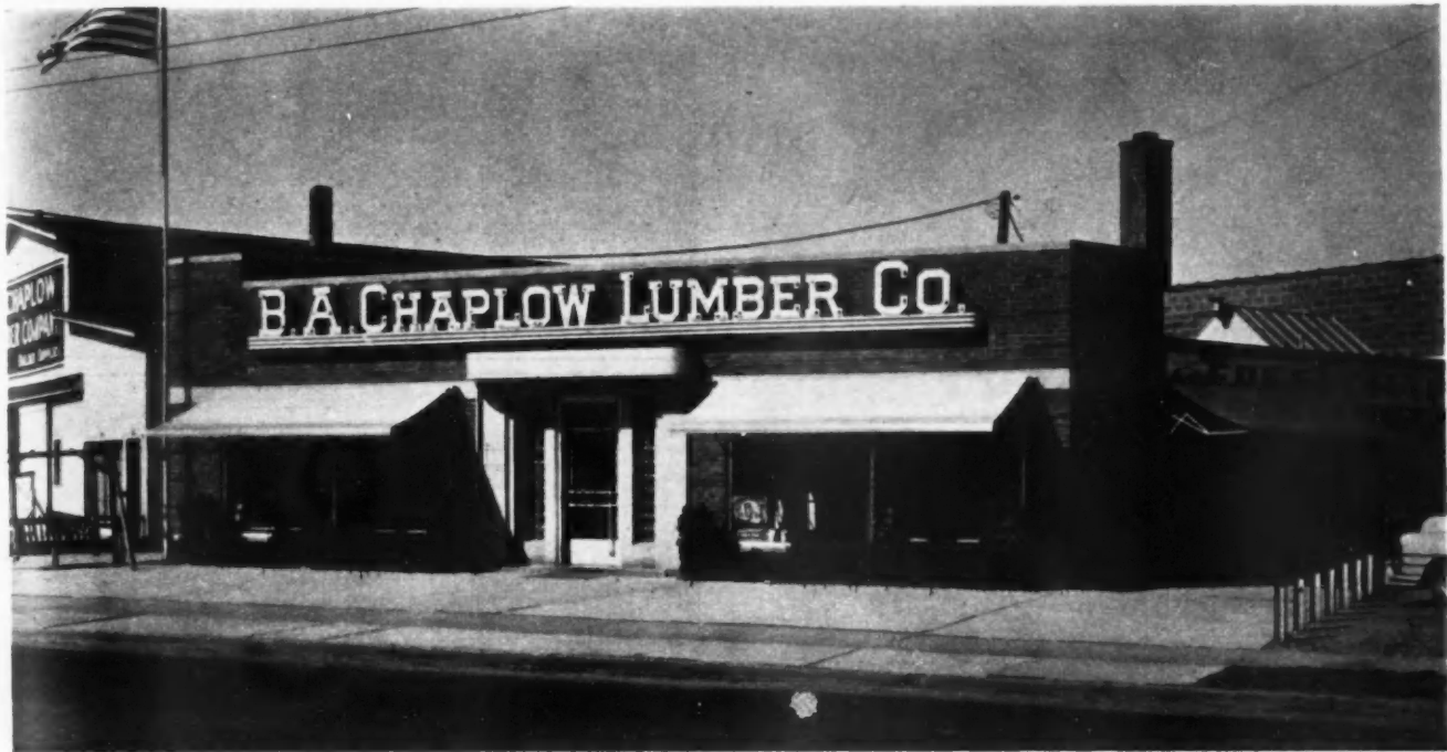
This building, 50x150 feet, houses sales room and offices. There is space for 65 cars in parking lot at right of store
