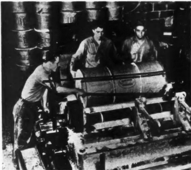
3. ROTARY knives cut the cotton insulation into specified widths before it is attached to the waterproof backing
