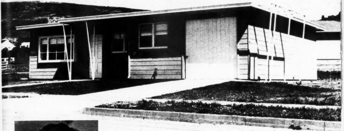
COST savings are obtained with flat roof construction
