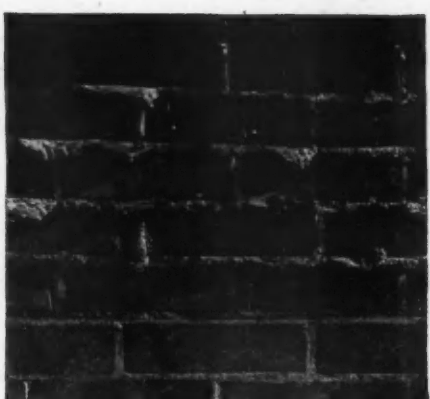
Before backplastering, however, all mortar joints should be cut flush. Parging should not be attempted over protruding mortar joints.
