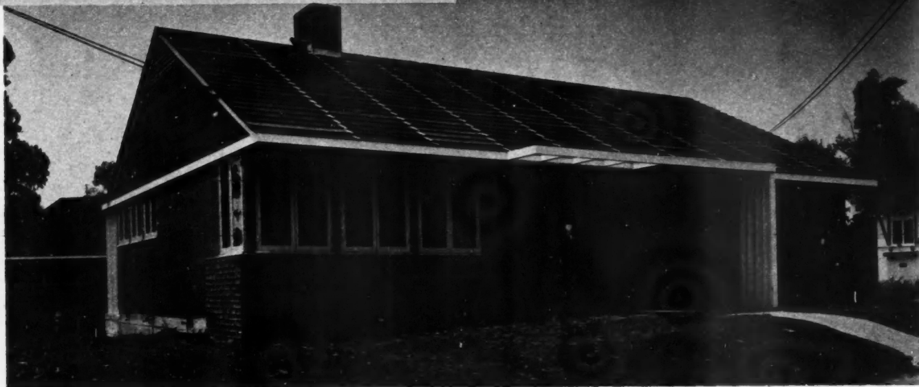
ROOF is covered with 1x12 rough redwood boards in 4-foot lengths fitted to rafters with 2-inch lap joints.
