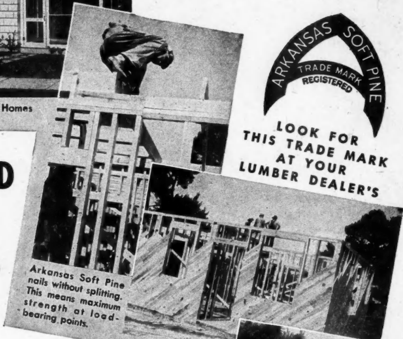
End-matched sheathing and sub-flooring work fast, disregarding stud and joist centers.
