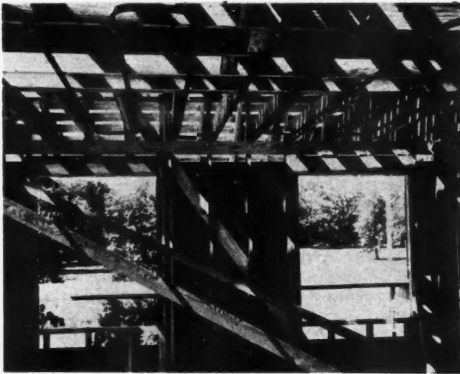
INSTALLATION of iron piping for ceiling panels is shown above.
