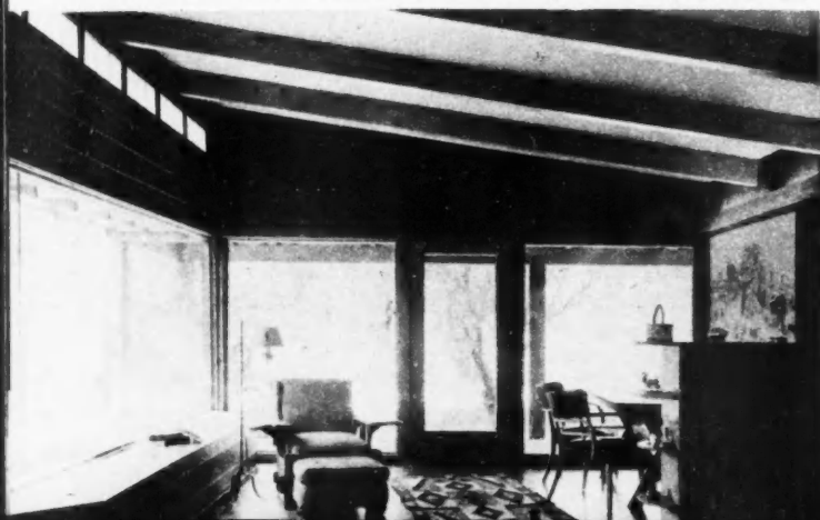
EXPOSED wooden beams support the living and dining room ceilings.
