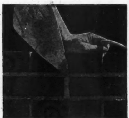
Therefore before the tooling can be completed, it is necessary for the bricklayer to point up the open joints.
