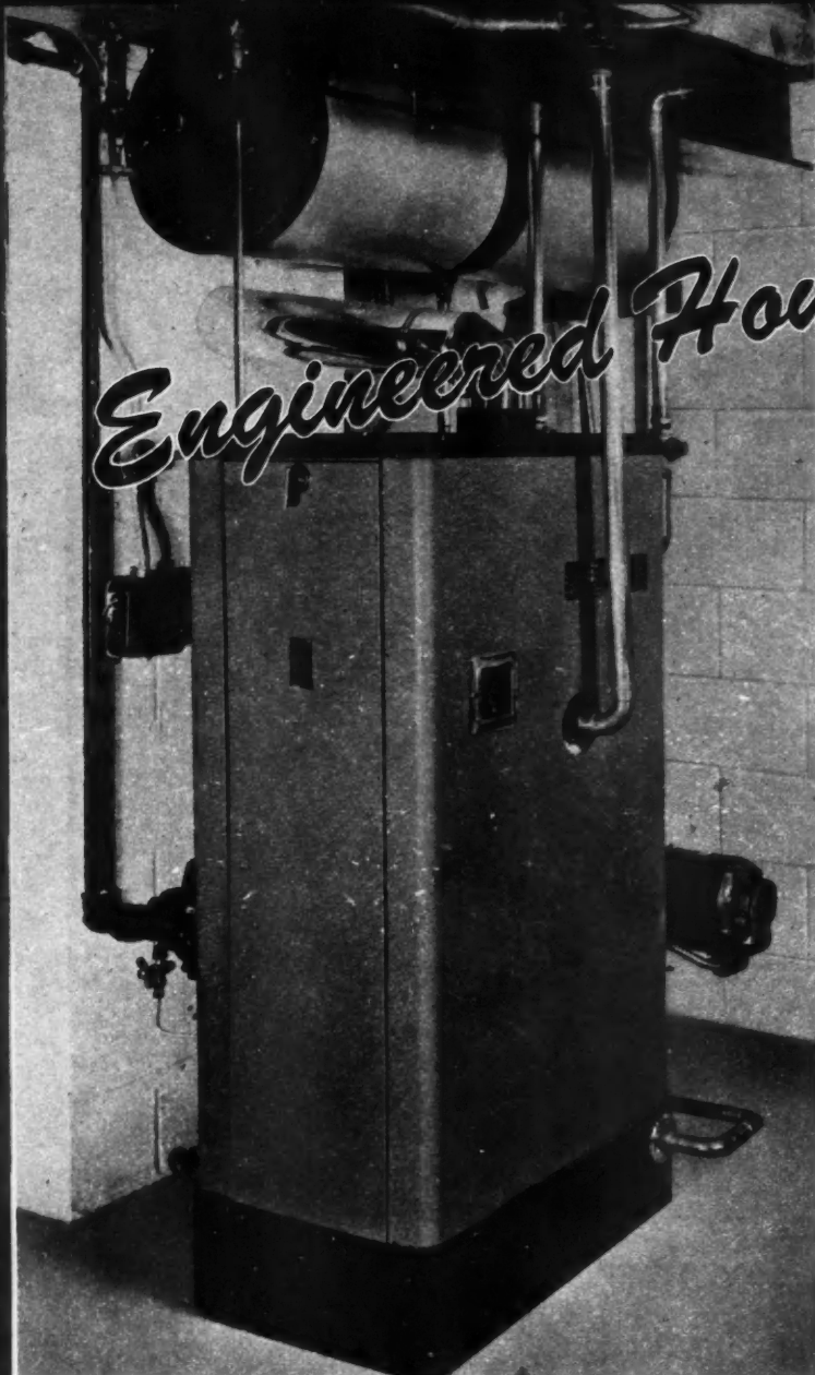
BOILER may be same type as for conventional automatic system.
