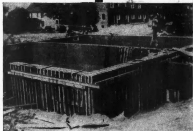
Stripping the forms. Note clean, smooth surface.
