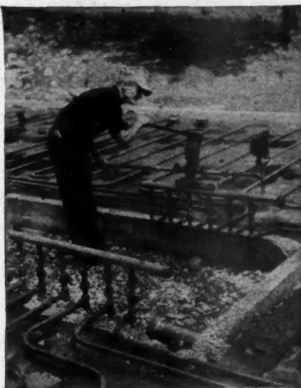
TEST run on piping to guard against leaks.
