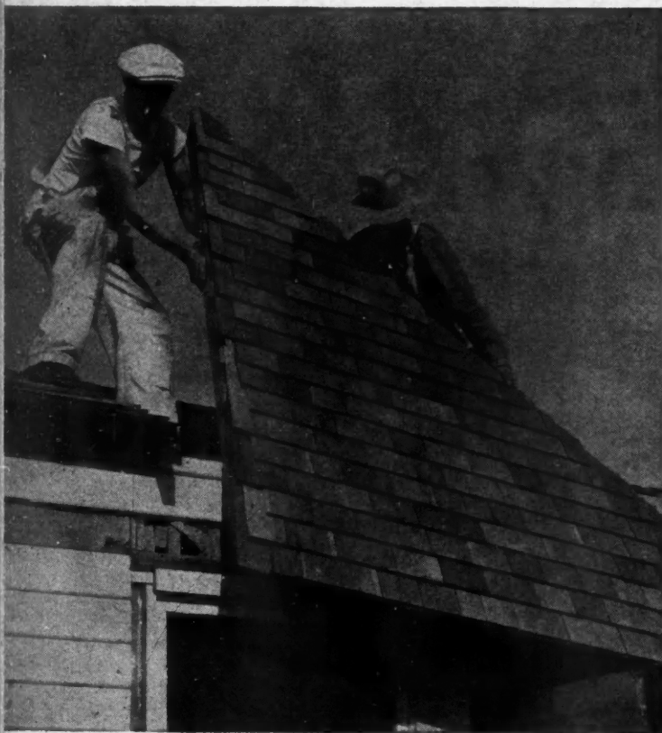
ROOF sections arrive ready for erection complete with shingles.
