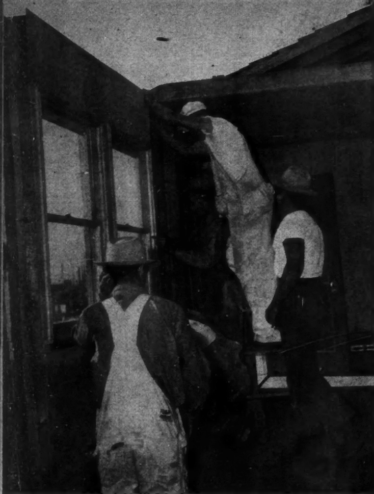
ALL sections interlock and are bolted together at the joints.
