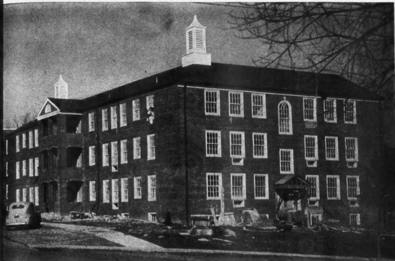
design on each individual building to avoid a repetitious similarity, yet maintaining a unity of expression.
