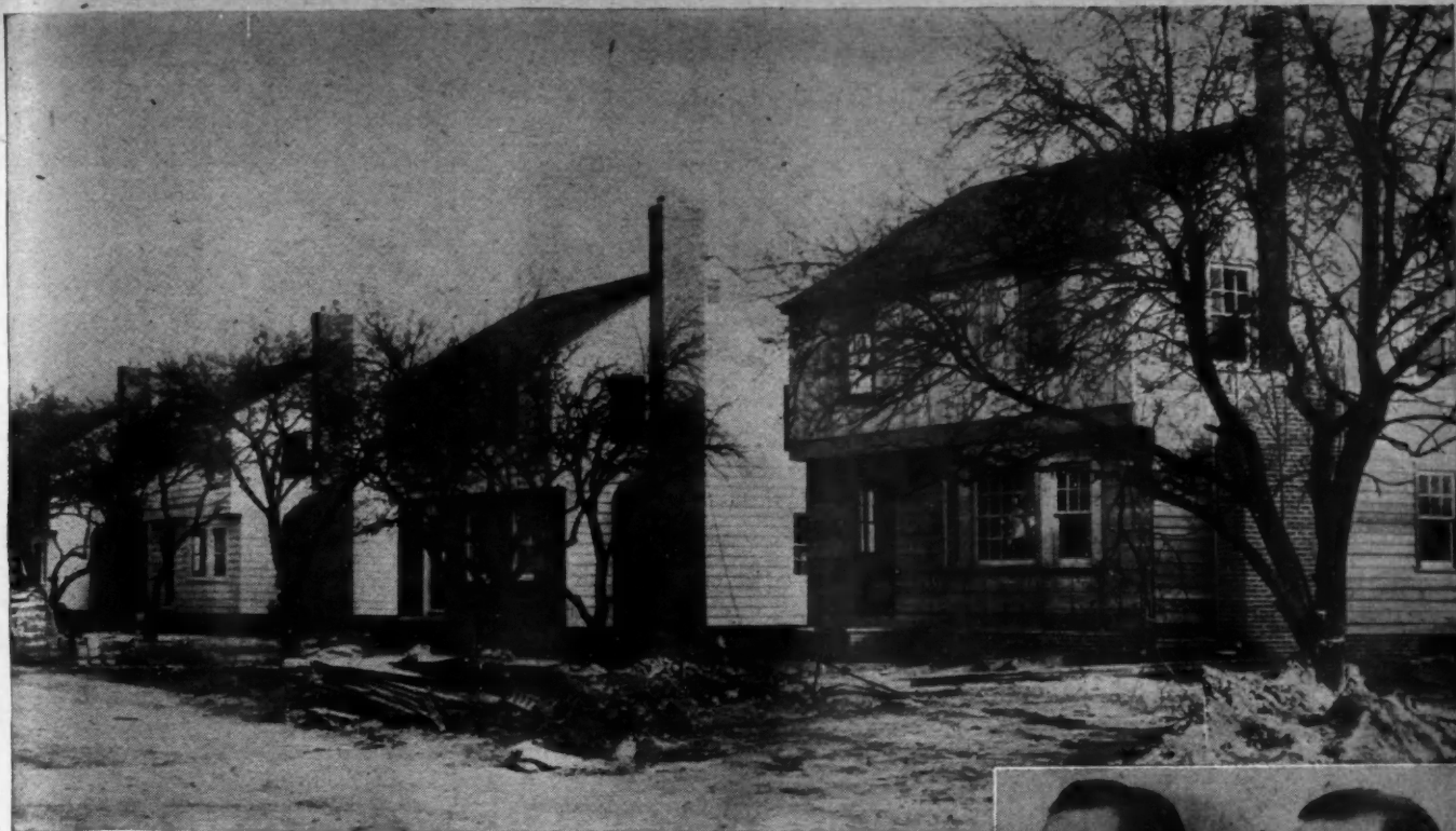
OTHER Inwood Place homes under construction, indicating victory over shortages.
