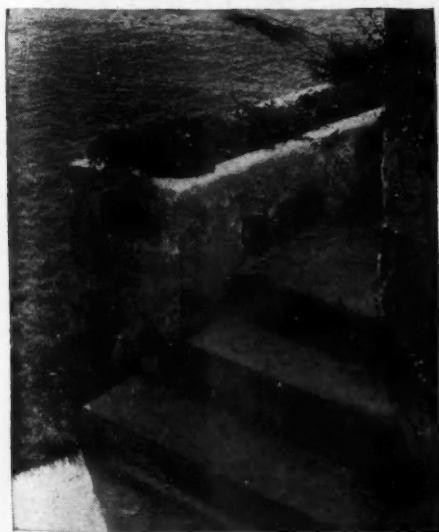
RECESSED light at steps for safety.
