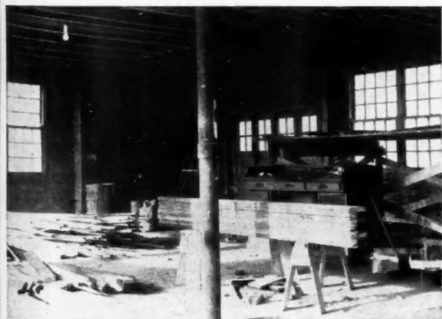
THE interior of the sign shop before conversion was started.
