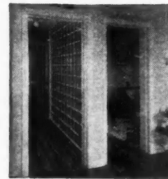
An Insulux panel can be used to carry natural light from room to room for brightening dark corners.
