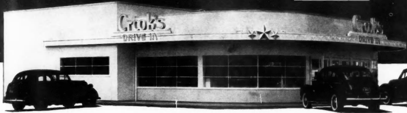
This beautiful drive-in restaurant, just south of Tacoma, Washington, on Highway 99, is a pleasing example of the smooth, streamlined, modern effects made possible with Exterior type Douglas fir plywood. Notice the curved surfaces—easily achieved with this modern "miracle wood."
