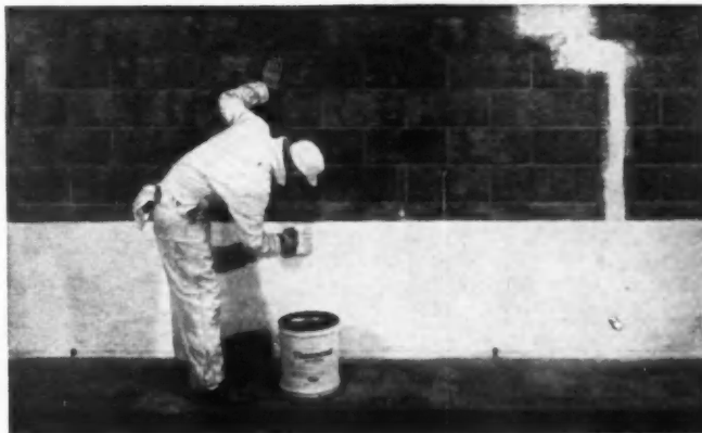
B. THOROSEAL, a slow-set hydraulic compound, gives the applier 3 to 4 hours, before set begins, to brush THOROSEAL into the masonry surface. (Scrubbing not necessary, as THOROSEAL is prepared especially to flow easily and quickly into every crack, void and defect in the surface, where it becomes structurally stronger than the surface to which applied.)
