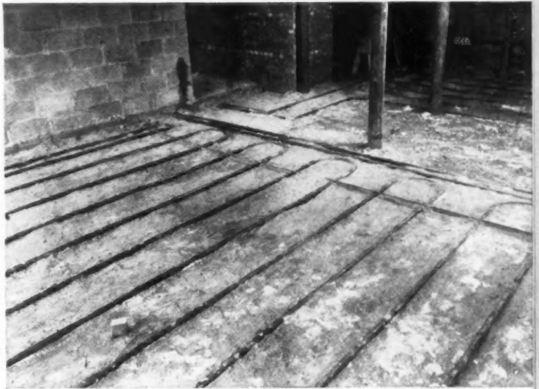
PIPE COILS positioned before pouring concrete floor slab.
