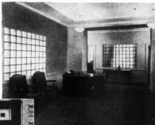
Building Managers use partitions of Insulux to transmit daylight from office to office.
