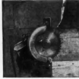
Trimming Odd Lengths of lumber on sheathing work with Cross Cut Blade.
