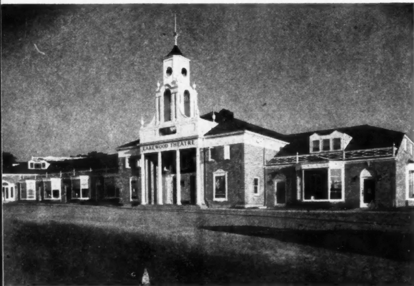
LEFT: LAKEWOOD Community Center near "the lakes" 9 miles west of Tacoma, Washington; Silas E. Nelsen, architect; C. M. Martinson, general contractor; Lakewood Development Company, owner. Below: Well-stocked grocery, fruit, vegetable, and meat markets are centers of local trade.
