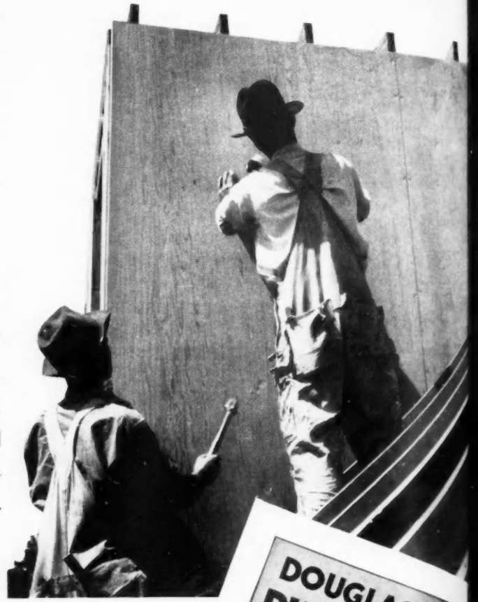
Plywood sheathing covers large areas with maximum speed, affords greater wall strength.
