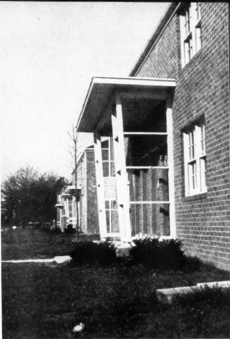
CLEAN, attractive architecture with enough variation between building entrances to avoid monotony enhances Woods End apartments. Trees and shrubbery will eventually soften their lines.
