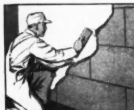
INSIDE. Sealed Graylite Lok-Joint Lath supplies a second wall of insulation. The patented "Lok-Joint" gives a strong, rigid plastering base, prevents joints from opening under trowel pressure.
