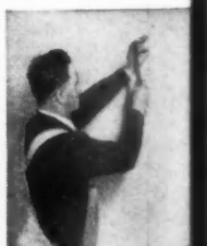
For Home Repairs. Apply fireproof Gold Bond Gypsum Wallboard directly to 2x4's or over old material. Takes paint, paper or other decoration.
