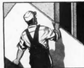
OUTSIDE. Insulite Bildrite Sheathing. Large water-proofed boards build a wind-proofed, weather-tight wall. Bildrite Sheathing has a bracing strength four times that of wood sheathing, horizontally applied—and builds an outer wall of insulation.
