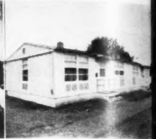
For multiple-unit housing in all parts of the nation, plywood inside and outside walls have supplied the need.
