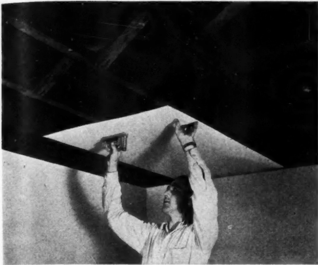
WORKMAN applying Carey Asbestos heat duct.
