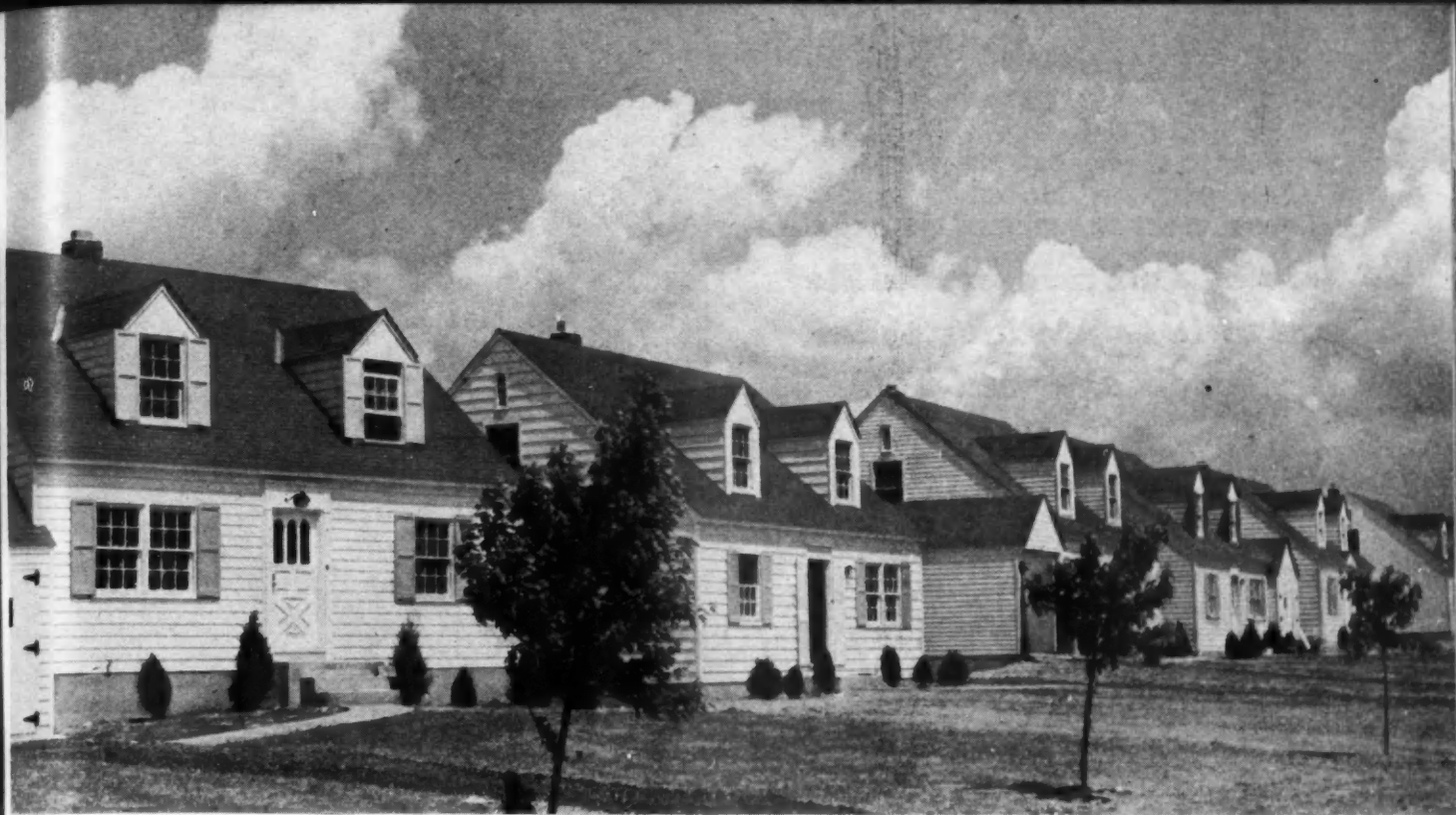
FOR $40 A MONTH Schenectady war workers get these fine homes in Niskayuna Estates—sold under revised FHA Title VI terms.
