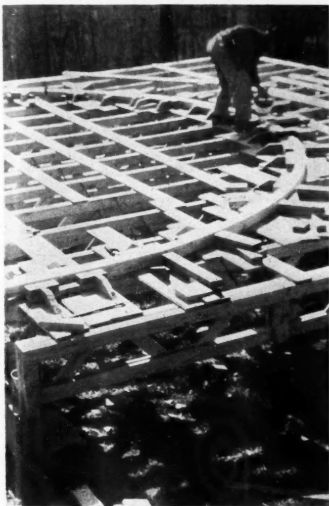
CURVED rafter is made of four 1 by 4's bent to shape in form and glued; note floor trusses, 15" deep, 24" o.c., made of doubled 1 x 4's, braced—a shock-proof floor.
