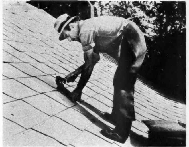
BOSTITCH stapler used to secure asphalt shingles.
