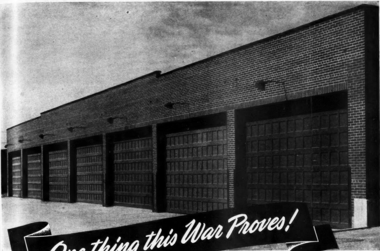
Warehouse of American Stores Co., Baltimore, Md. Equipped with 7 Ro-Way Doors. Consolidated Engr. Co., Contractors.
