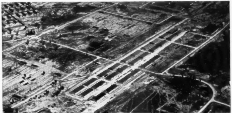
CAMP FOR SOLDIERS: Barracks foundations, roads, sewage disposal plant and other concrete construction were hastened to completion by Lehigh Early Strength Cement.
