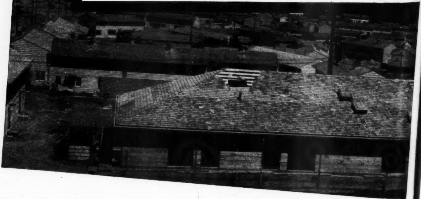
DOUBLE-COURSED RED CEDAR SHINGLE SIDEWALLS PROVIDE STRENGTH AND BEAUTY FOR 40% OF THE HIGH POINT UNITS. NOTE WIDE WEATHER EXPOSURES THAT MAKE DOUBLE-COURSING HIGHLY PRACTICAL.
