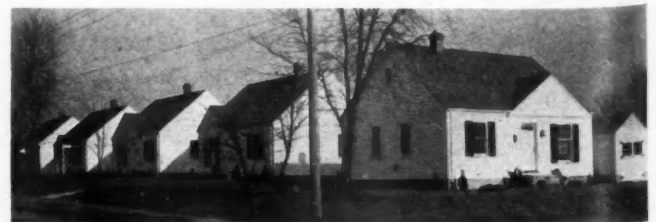
4300 square yards of Nairn Linoleum for kitchen and bathroom floors, cove base and kitchen drainboards were installed in these 226 houses, by the Turner Wallpaper Company, Akron, Ohio.
