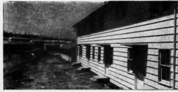
DOUBLE-COURSED RED CEDAR SHINGLE SIDEWALLS PROVIDE STRENGTH AND BEAUTY FOR 40% OF THE HIGH POINT UNITS. NOTE WIDE WEATHER EXPOSURES THAT MAKE DOUBLE-COURSING HIGHLY PRACTICAL.
