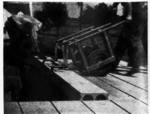
Special cart greatly facilitates installation of units.
