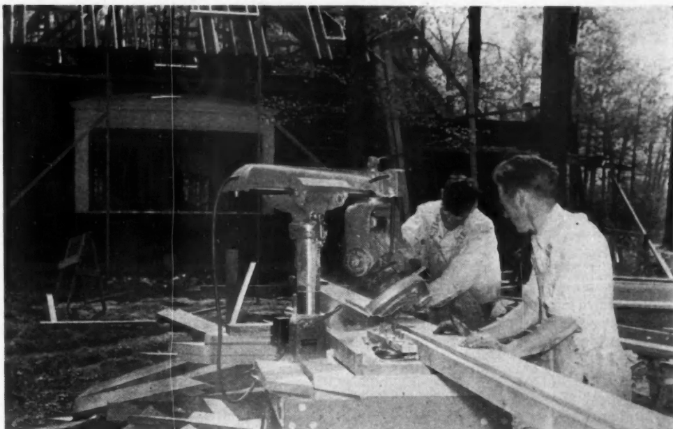
RADIAL SAW in use on Medical Center, last job Ogden did before converting to war work.
