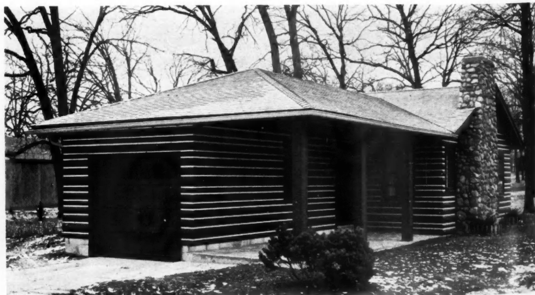
WITH an exterior of log cabin siding, open porch and stone chimney, this five-room basementless house fits into its rustic site near Chicago. The garage and porch might be added later if small space heater and fireplace are adequate. The plans are opposite.
