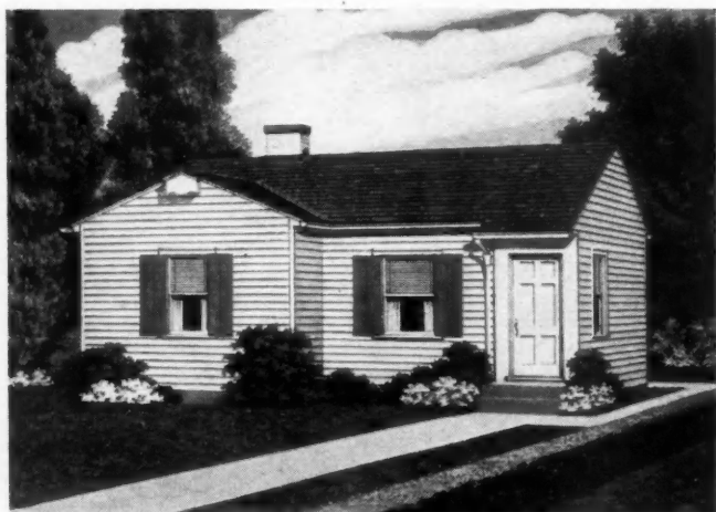
FOUR-room starting units measures 26' by 25½' and cubes 11,200' with full excavated basement. Below, and to right, are shown planned extensions providing new larger living room, enlarged front bedroom and ample porch.
