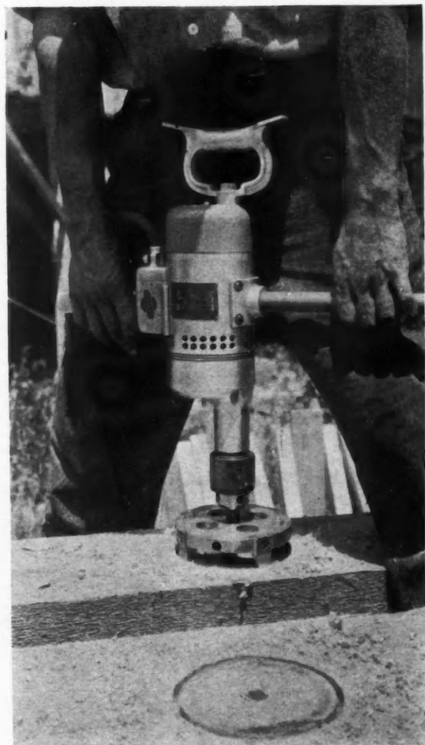
CUTTING grooves for 4-inch split rings with 3/4-inch electric drill.
