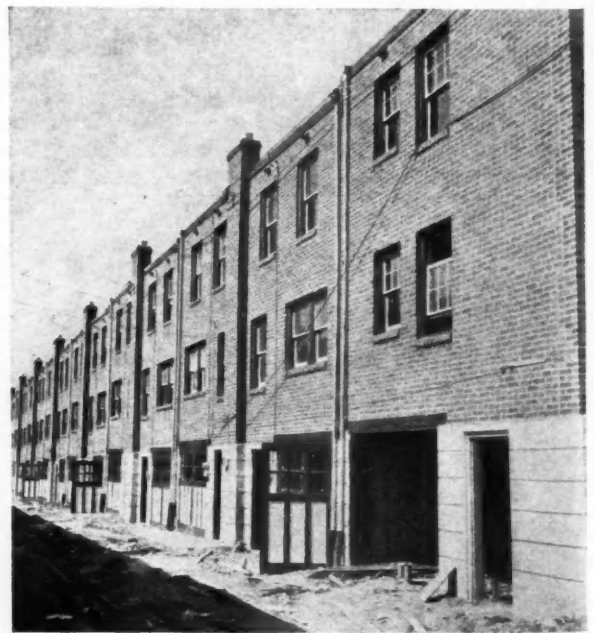
REAR VIEW of Orleans Philadelphia row house project showing garage and back door entrances and chimney detail. Area between rows is paved and each house has individual garage.
