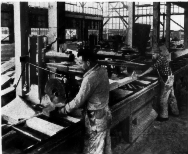
TRIMMING truss part to specifications using positioned saws, one making a square cut and the other a diagonal cut.
