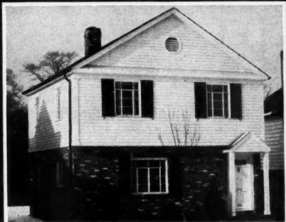
RESIDENCE LONG ISLAND, N. Y. HOLLIS HILLS, INC. Ira Bernkopf, Builder Lester Maxon, Arch't.
