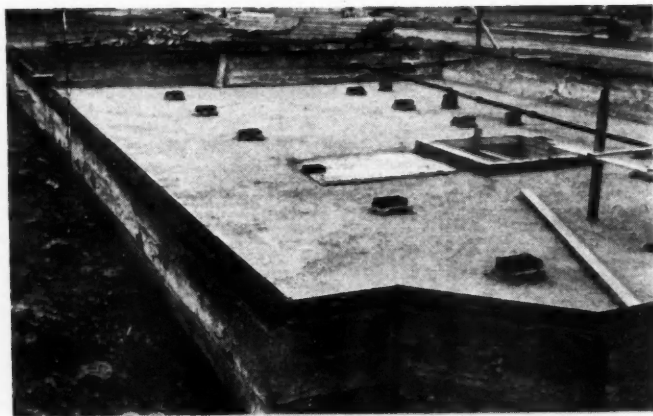
SUBSTANTIAL FOUNDATION, creosoted sills and plates. Ground in basementless house is covered with layer of cinder concrete. Floor framing is more than ample.
