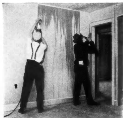
Sanding off glue at joints of Mengel Bord, and applying trim before papering and painting.
