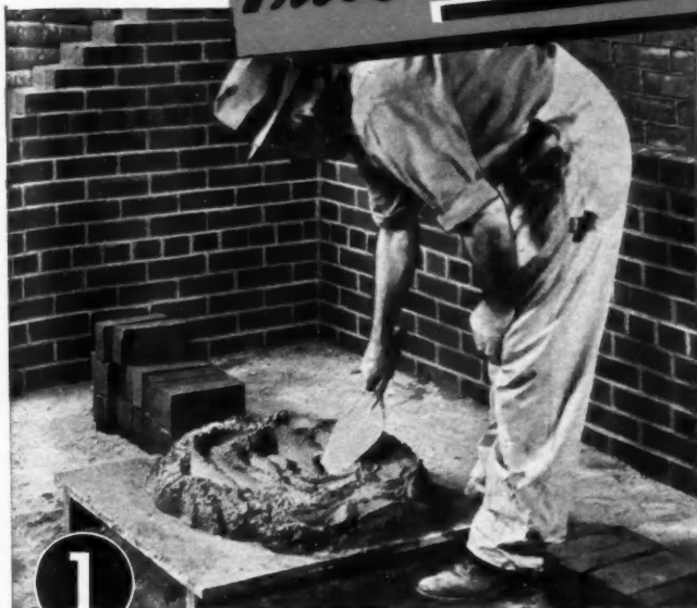
1 Mix a batch of 1-3 Brixment mortar (above) and a batch of 50-50 cement-lime mortar made with the same proportion of sand (right). Get any competent bricklayer to test
