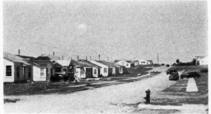
CONSTRUCTION VIEW looking down the street of
