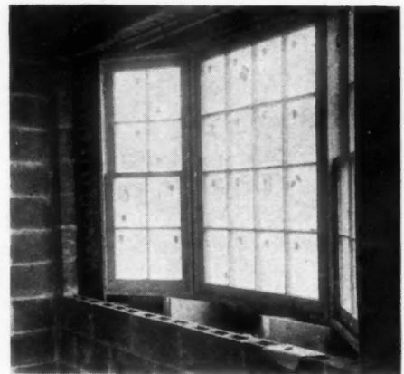
ABOVE: View of Mills & Sons' "Westbrook" defense home showing close-up from the rear. Note breather tubes at bottom of brick.
