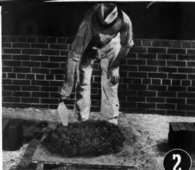
2 them on the board—to spread them on the wall—to lay up a few brick with each of the two mortars. Then ask him which has the best workability.
