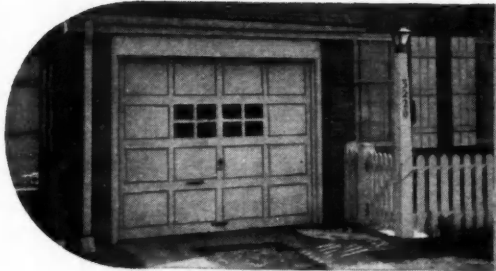
Attractive bungalow with attached garage equipped with Ro-Way Doors. Paul Brim, Toledo, Ohio, Architect and Builder.
