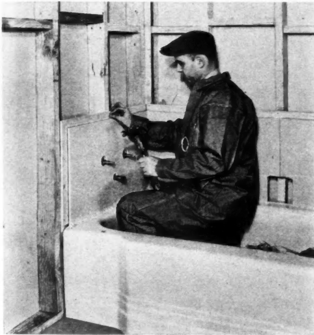
PREFABRICATED Vitrolite structural glass units are nailed to studding in this manner, making installation by a carpenter possible. The edges of Vitrolite resting on the tub are buttered with pointing compound before sections are nailed.
