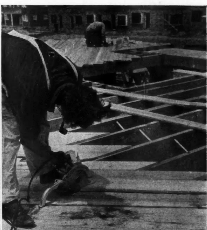
SIX FAST, POWERFUL ELECTRIC SAWS are kept in operation on the Marling job. These views were taken on the second floor of latest group of row houses. Note quick, exact cutting of diagonal flooring.
