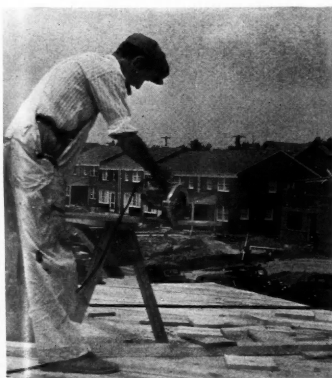
SIX FAST, POWERFUL ELECTRIC SAWS are kept in operation on the Marling job. These views were taken on the second floor of latest group of row houses. Note quick, exact cutting of diagonal flooring.
