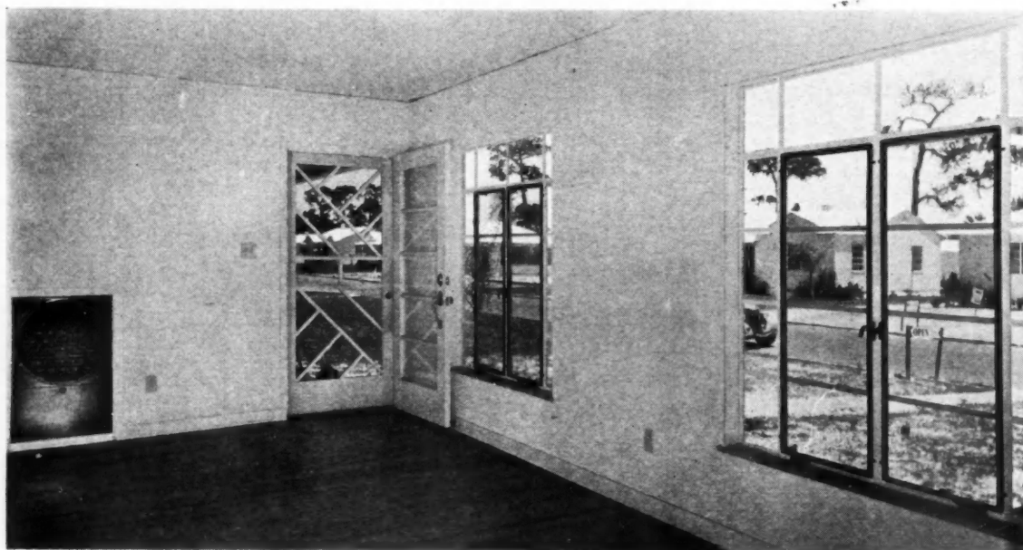
MODEL HOME living room, showing gas heater at left, decorative screen door, center, and large metal windows with tile sills. (See window drawing detail opposite.)
