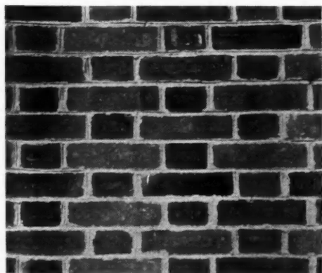
RIGHT: Table analyzing brick bonds. Below: Upper view shows headers and stretchers alternating in each Flemish bond course; lower view, novel Rolok bond with all bricks laid on edge.
