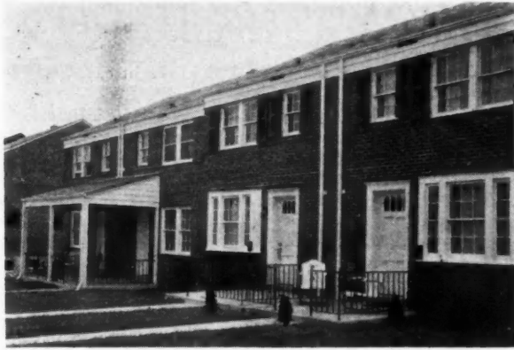
OPEN AND COVERED porches with wrought-iron railings contribute to appeal of W. E. Marling's row houses in Towson, Md.
