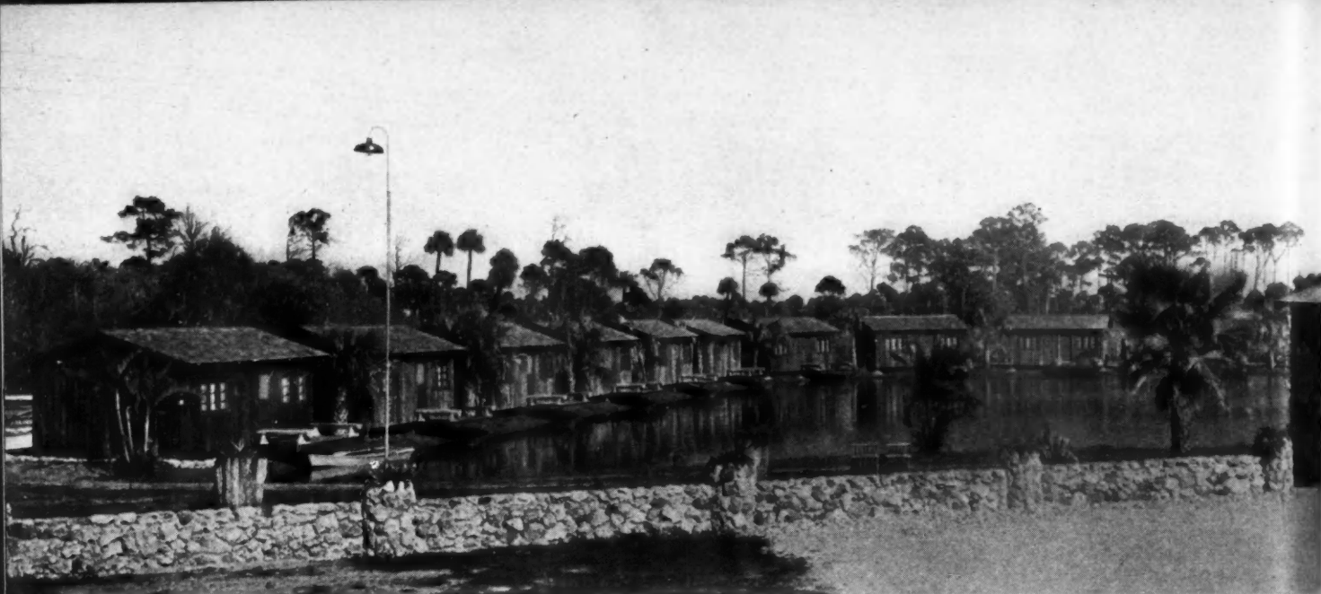
SAWED CYPRESS LOGS on end were used in building these appealing Florida cabins around a small lake.
