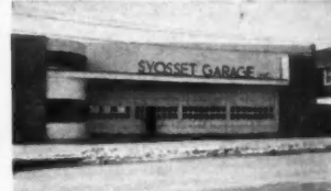
Syosset Garage, Syosset, Long Island, N. Y., equipped with 4 Ro-Way Overhead Type Doors Krebs & Schulz, Contractors.
