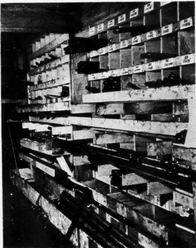
PRECUT PIPE and sub-assemblies are stored in bins (left) until needed at job site. AT RIGHT—workmen attach prefabricated sub-assembly to factory-tested oil boiler.
