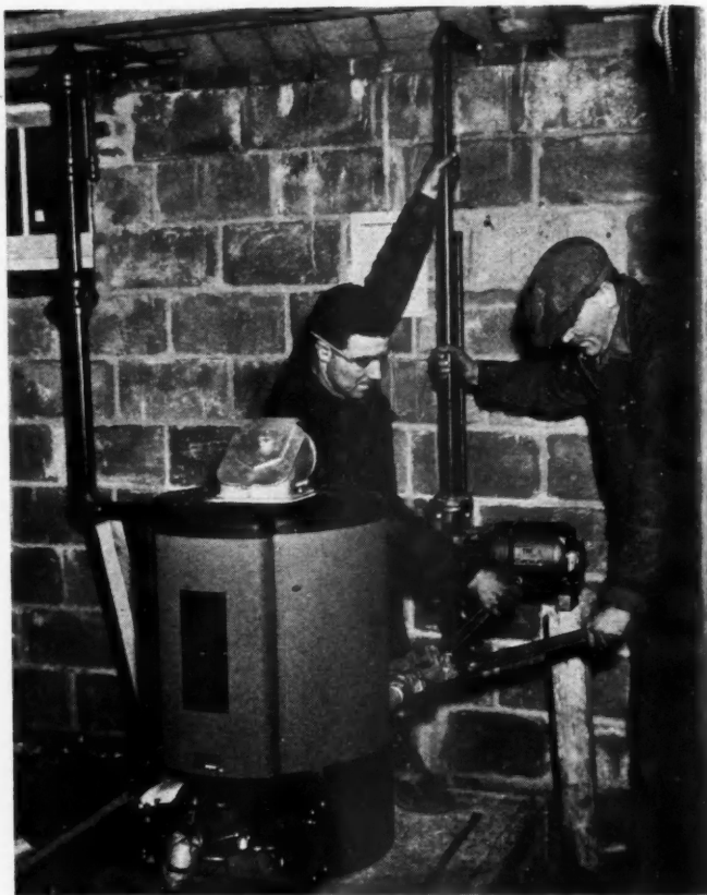
PRECUT PIPE and sub-assemblies are stored in bins (left) until needed at job site. AT RIGHT—workmen attach prefabricated sub-assembly to factory-tested oil boiler.
