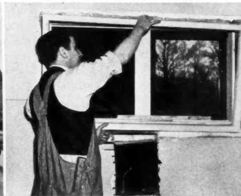
HOW JOB WAS DONE—at left, new wiring and new piping installed. CENTER—new window frame goes into place. RIGHT—putting finishing touches on new linoleum ceiling.
