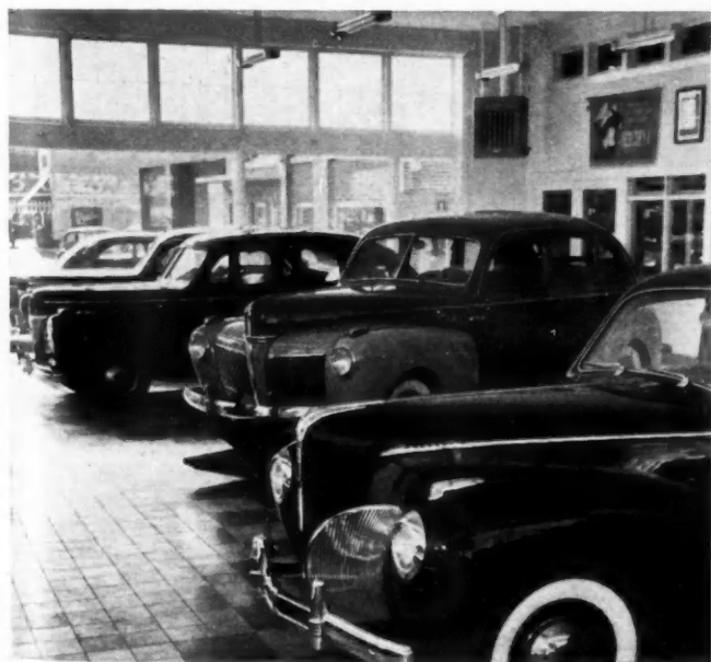
LARGE, clear floor area tiled, fluorescent lighting, and unit heaters, are features in DeVan Motor Company showroom.
