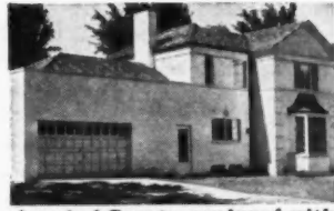
Attached Garage, equipped with Ro - Way "Two - Car" Overhead Type Door, Architect, Aldrich & Aldrich, Galesburg, Ill.
