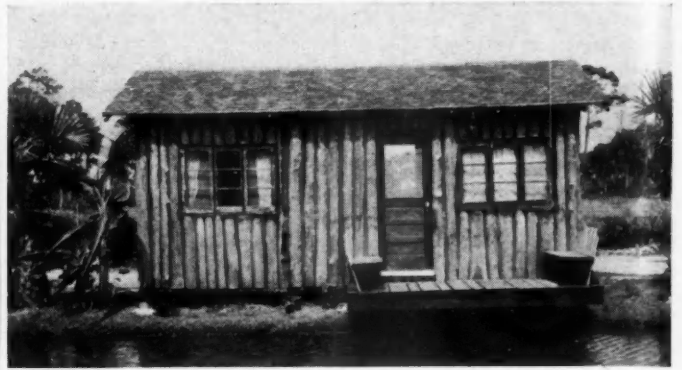
ONE OF SCOTTIE'S typical cabins built of vertical cypress logs.
