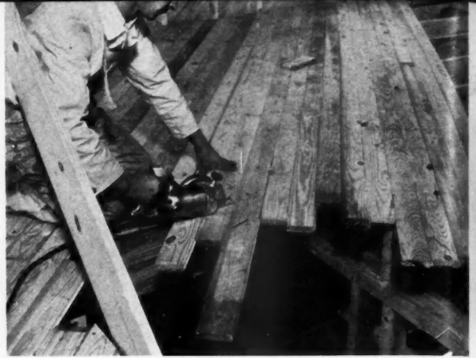
CUTTING OUT openings takes only a few moments.
