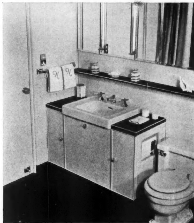
LINOLEUM covered cabinet and shelf contribute to convenience of the modernized bathroom. Door was rebuilt with plywood and covered with linoleum.
