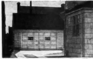
Detached garage, with Ro - Way Overhead Type Door, Toledo, Ohio, residence of Ray Shaffner. Architect, Harold Spooner.
