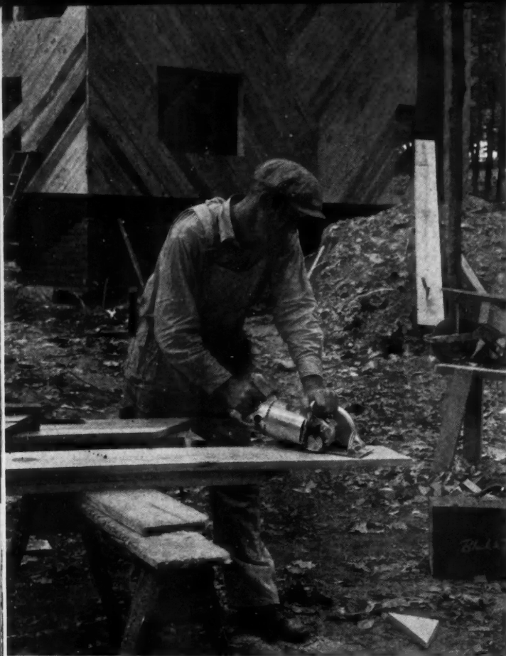
LIGHT SAW does rapid work cutting diagonal sheathing.
