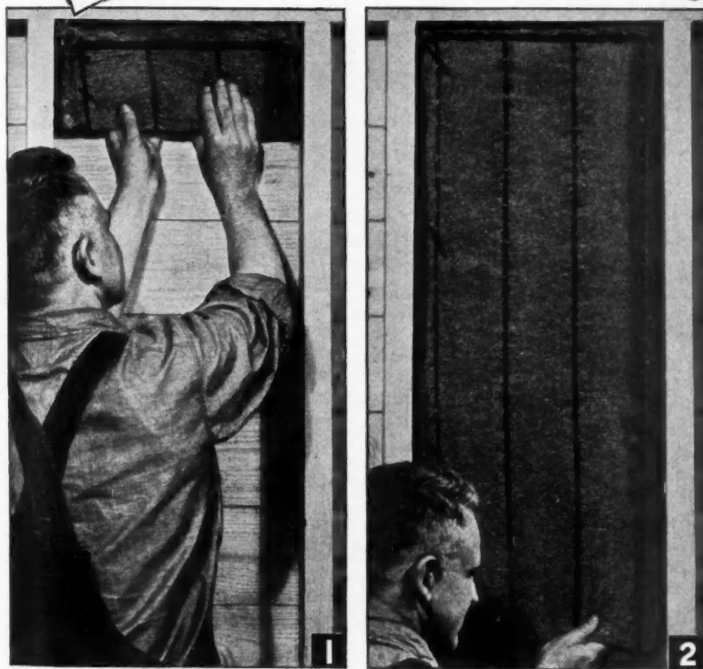
KIMSUL IS COMPRESSED AT THE FACTORY — EXPANDED ON THE JOB
