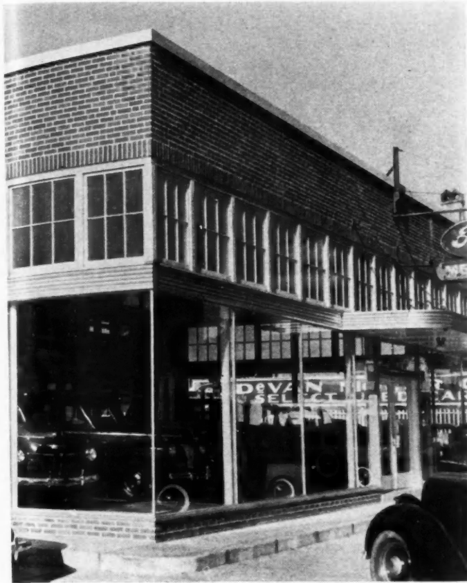
ABOVE: Close-up of showroom; note absence of the display window corner posts.
