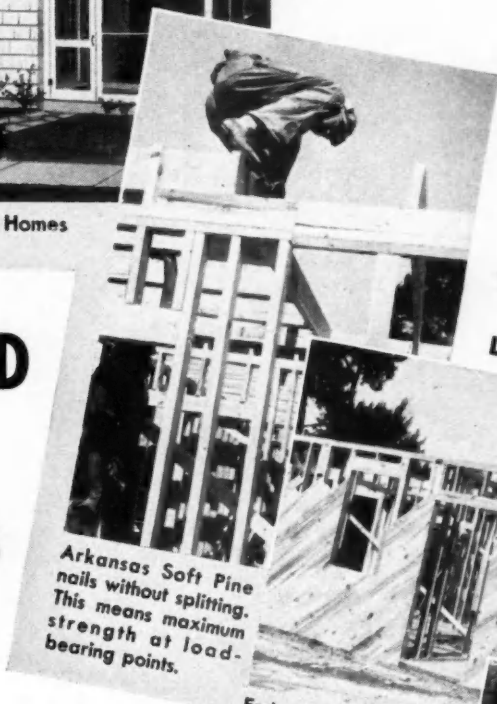
End-matched sheathing and sub-flooring work fast, disregarding stud and joist centers.
