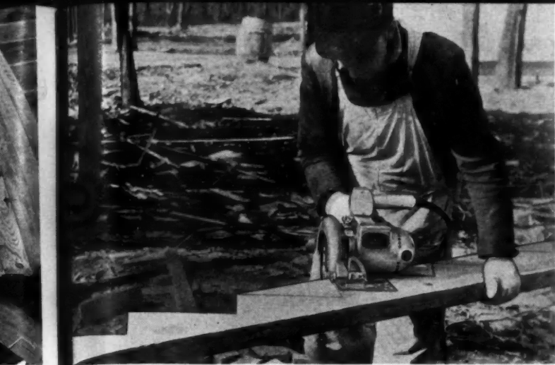
HALF A DAY is saved in cutting stair carriages.
