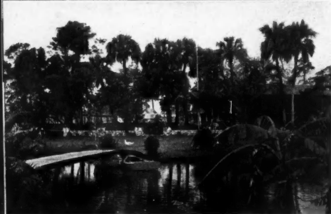
RUSTIC BRIDGE leads to small island in center of lake. Cabins rest on heartwood pitch pine piling.
