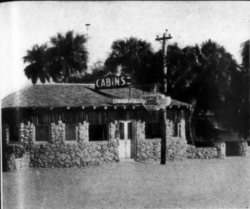
VERTICAL LOGS and local stone were used for Coffee Shop.
