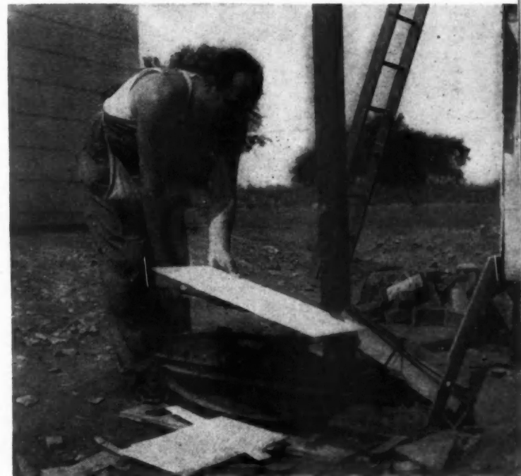
HANDY CUTTER notches asbestos siding for close fitting around window and door openings.
