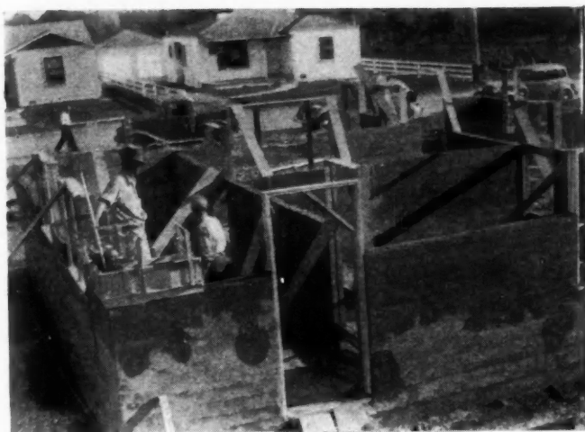
"Terracrete" house under construction
