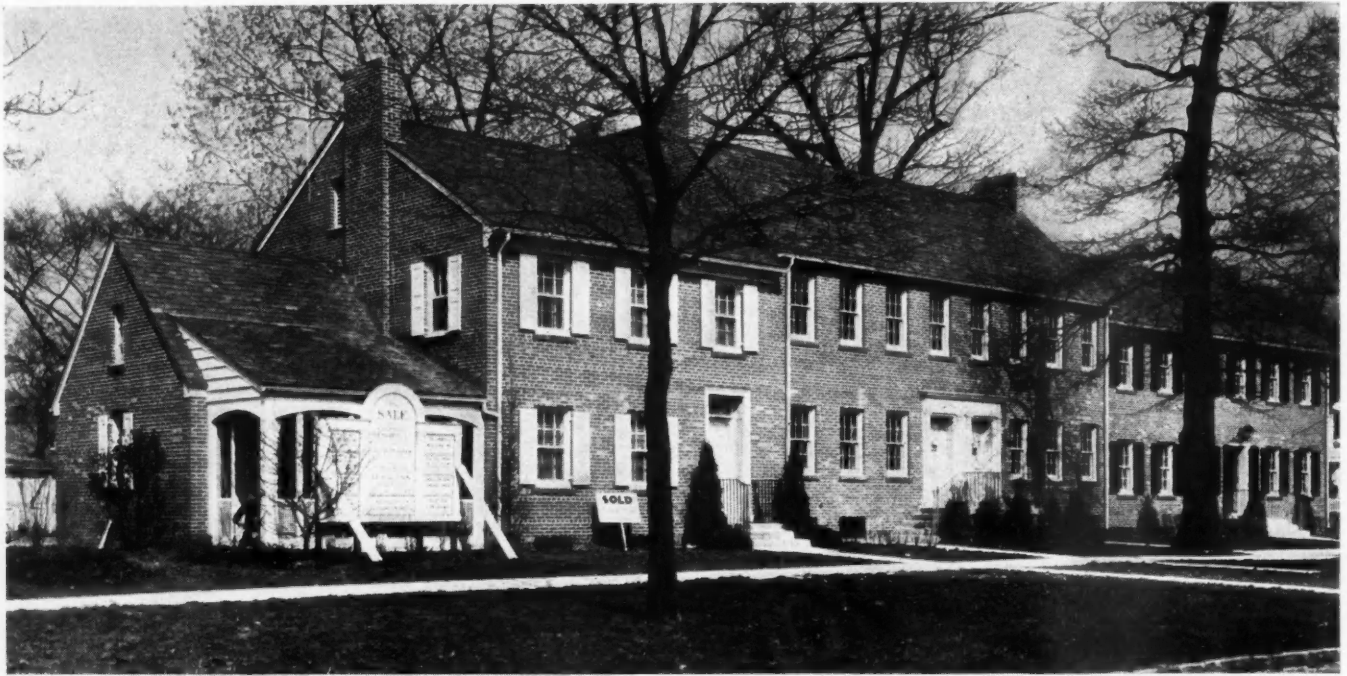
EAST elevation of Evanston, Ill., row house: Architect Kegley's home is one at the left; three other units face on this street.
