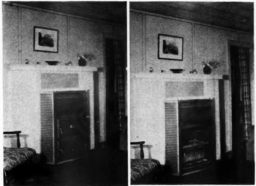
"Firedaire" in cottage; left, with furnace doors, right, with doors removed for use as open fireplace. Floor plan above shows heat distribution to bedrooms and bath.
