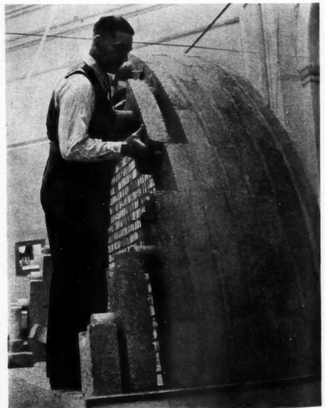
A product of the war in England is this concrete building unit for air raid shelters and the like. It is oblong in shape with a round spud inserted in the side to engage rounded contour of block ends in the next course of construction.
