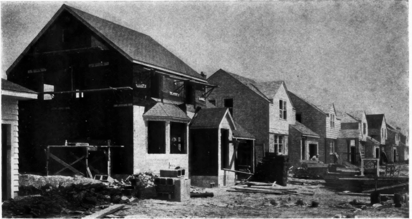
WEBER BROTHERS of Buffalo are building a full street of houses that can be owned for "less than rent." Insulating sheathing is used.
