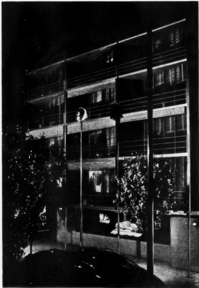
MODERN APARTMENT with first-floor store, as designed by Harrison and Foullhoux, for the Avenue of Tomorrow. Narrow balconies with simple metal railings provide a striking touch. Walls are of frosted glass.
