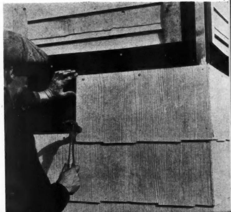
HANDY CUTTER notches asbestos siding for close fitting around window and door openings.
