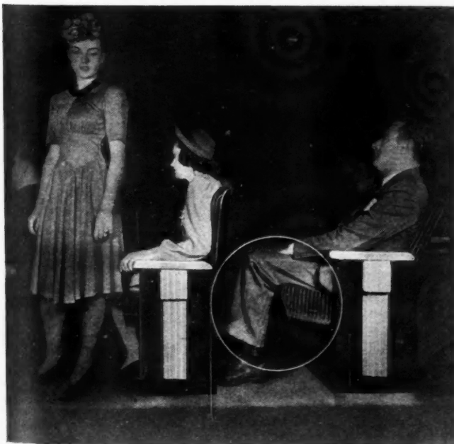
"PUSH-BACK" seats in the Lex Theatre permit patrons to pass in and out; a simple movement of the body changes the chair from the relax to the upright position adding the equivalent of 5 inches to row space.
