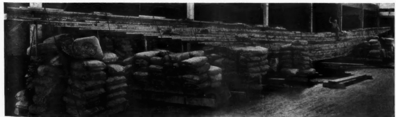
GIANT wood truss, built up of 2x10's glued, under test in shop of the Speedwall Company, Seattle.
