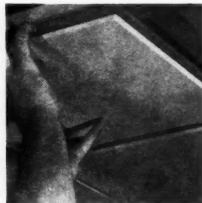
The male edge of the "next" unit is pushed against the sharp prongs of the Tem-Clips which have been nailed in place against the female edge of the unit already installed.
