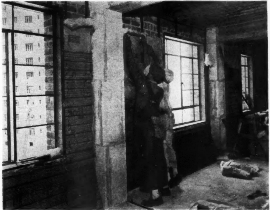
MINERAL WOOL on walls will cut annual heating cost $40,000.
