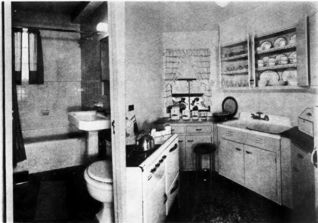
BATHS throughout project are identical, with standardized equipment shown at far left. Tile floors, wainscoting are standard.
