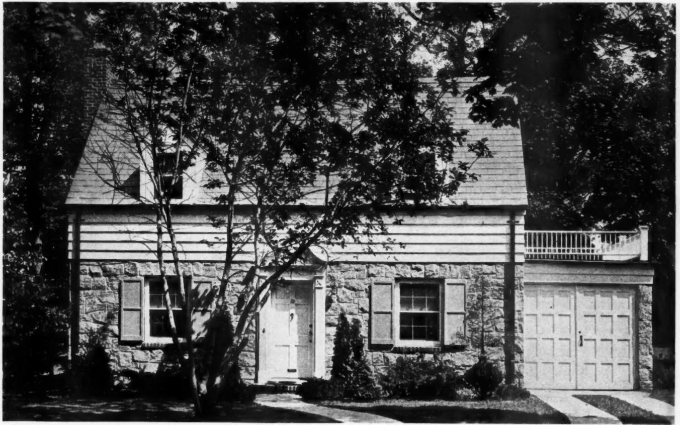
FIELDSTONE and clapboard house in Stich and Gibson's Hempstead Park Acres. Floor plan opposite.
