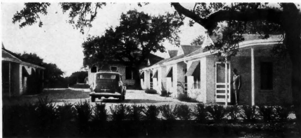
LOOKING down the paved court between the two rows of units of the State Motel in Texas, it will be noted that there is plenty of space to turn in under the car shelters.
