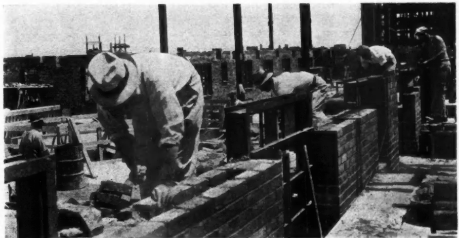
5,000 MEN were employed daily in building Parkchester.
