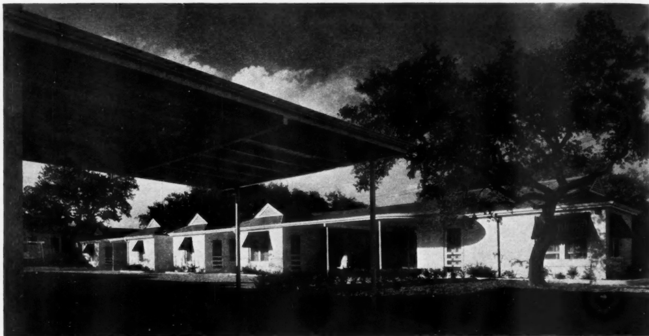
TRIM appearance of the State Motel, Texas, as seen above from the entrance, attracts tourists. L. L. McCandless, contractor.
