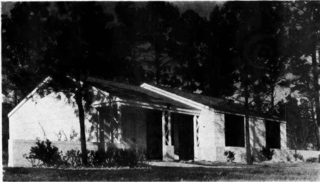
BROAD fronts to take advantage of the cooling Gull breezes are possible on the wide Garden Oaks sites, this spread-out idea developing a new type of architecture. Floor plan and section showing construction of this low-cost demonstration home appears below.
