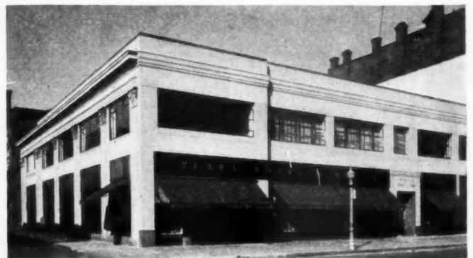
STORE building in New Haven, Conn., with colorful concrete exterior executed in architectural concrete slabs by Dextone Co.
