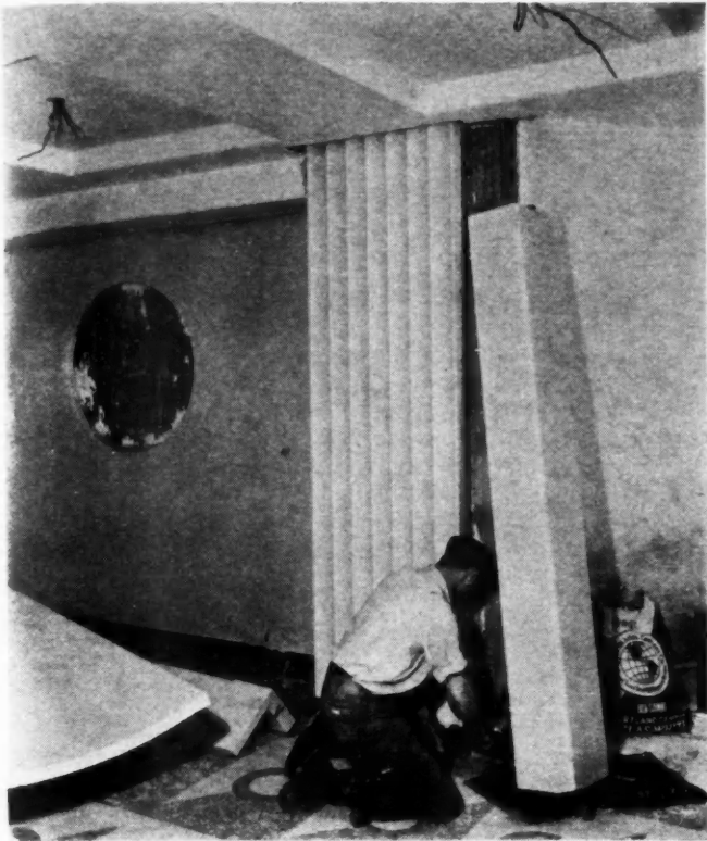
CURVED, fluted and angle-shaped precast panels used in Chrysler Building modernizing job, reception room of Universal Atlas Cement Co.
