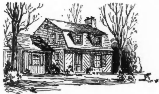
HORIZONTAL tongue and grooved boards separated by a moulded insert offer extreme emphasis to horizontals needed to reduce the apparent height of a narrow house.
