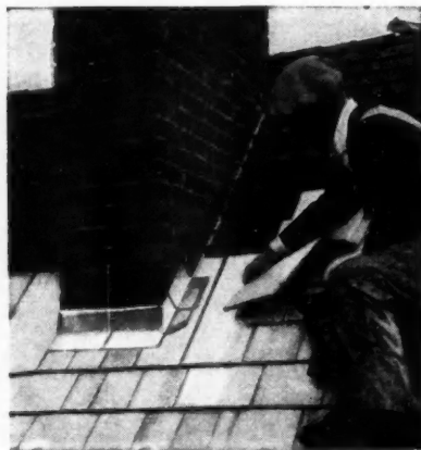
ABOVE: The Certigrade Label; LEFT: Laying Shingles right over old shingles. New chimney flashings have been applied.
