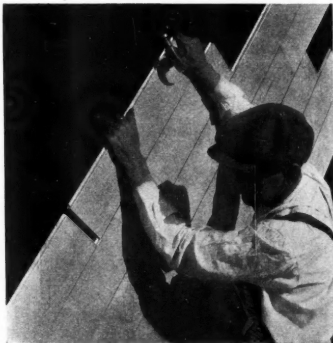
APPLYING end-matched sheathing diagonally, the strong way, is no more costly than putting on ordinary sheathing horizontally. Building authorities recommend diagonal sheathing because of the extra strength and rigidity it adds to the structure.
