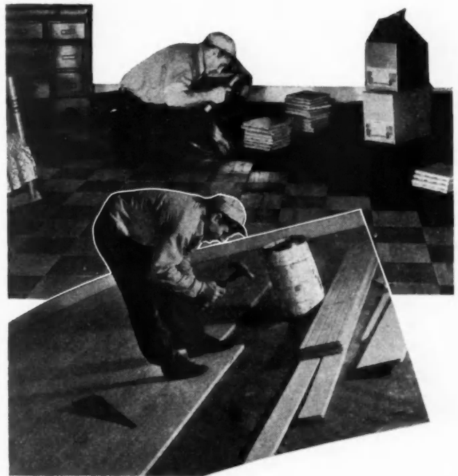
FACTORY finished block flooring comes in cartons, ready to lay; plank floors and strip flooring continue in popular favor.
