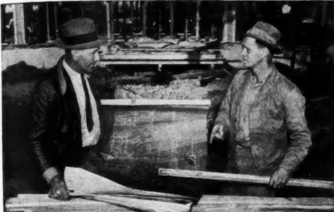
Photo taken at U. S. Housing Project No. TEX 5-1, Houston.
