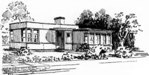
LOG CABIN siding laid vertically recalls vertical pole log houses. This type of siding provides an extra warm tight wall just as well suited to year-around as to summer dwellings.
