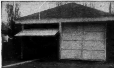
Two Craw-Fir-Dors installed in a double garage, 422 Washington St., Kenmore, N.Y., by Skillen Excavating Co.
