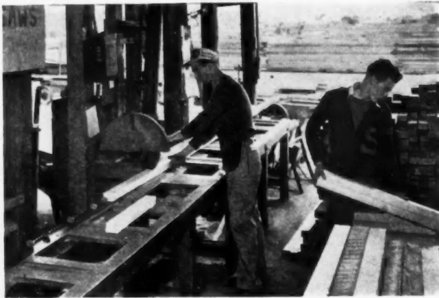
FRAMING MEMBERS are cut with accuracy, speed and precision.
