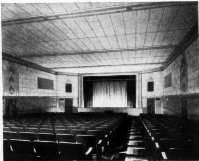
CEILING AND WALLS in the Emory Theater, Atlanta, Ga., are Temlok De Luxe for reverberation-control, attractive color (ash and cream), and fuel-saving insulation. Temlok Dealer: Willingham-Tift Lumber Company. General Contractor: Capitol Construction Company.
