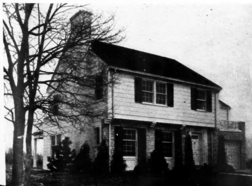
THIS 7-room house built by W. C. Tackett in his Scarsdale development has 2½ baths. The detail above presents a very attractive entrance and handling of the attached garage; a McKee upward-acting garage door was styled particularly for the design of this house.
