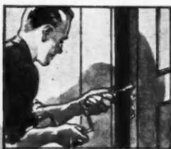
Bore hole in edge of door
