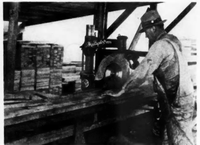
WORKMAN using saw on California school job.
