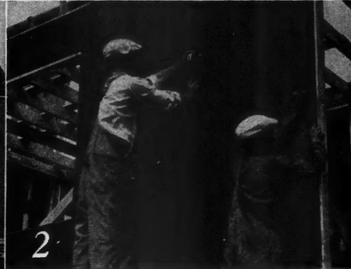
2 Applied quickly—every joint goes over stud, sill or header, thus reducing wind infiltration.
