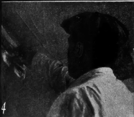
4 Providing both insulation and plaster base in one product. Note joint reinforcement.
