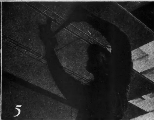
5 Sheets span 3 studs—yet one man handles easily.
