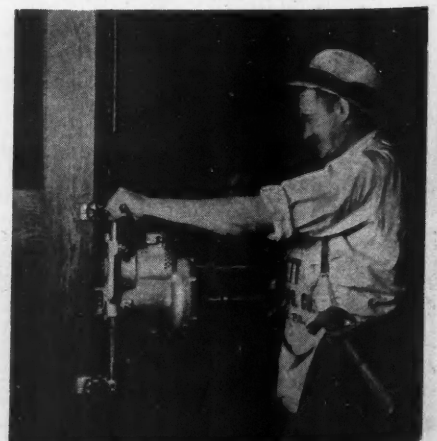
USING electric door mortiser.
