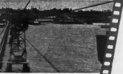
the half-mile cableway that leads to the end of the loading pier.
