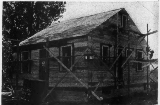
CONSTRUCTION is speeded and simplified by power-cut lumber.
