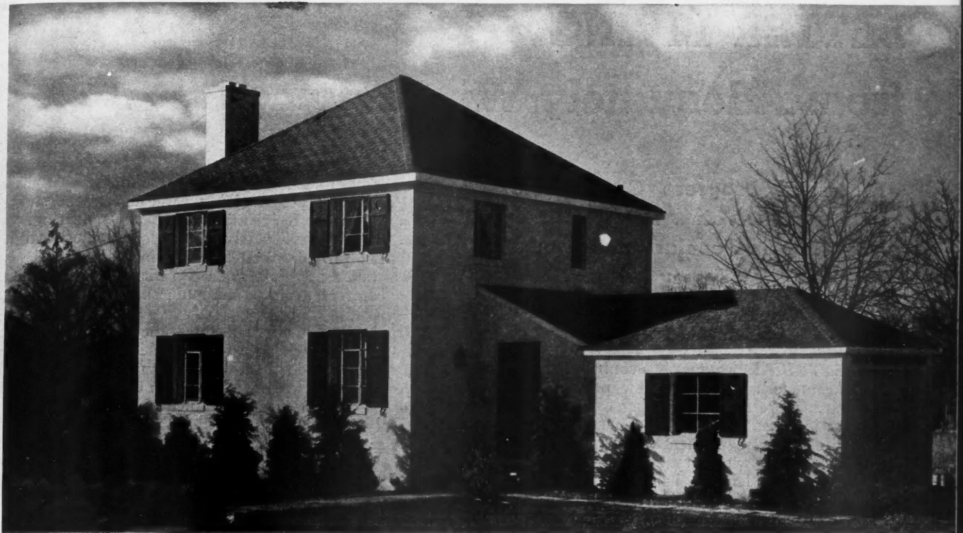
6-ROOM MASONRY HOUSE in Alden Estates, Port Chester, N. Y., is scientifically built to last indefinitely, with minimum upkeep costs. Walls are of double concrete block construction; floors are also of concrete.
