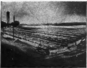
Bus Body Assembly Plant Wayne Works, Richmond, Ind. 1,300 tons of steel promptly supplied from stock!
