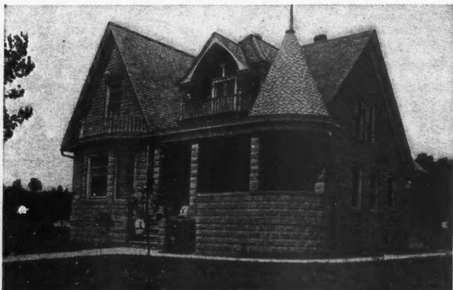
ROCK-FACED cement block was a popular novelty in 1908 when this sturdy but somewhat warty dwelling was illustrated in the "American Builder." The tower roof was a master touch.
