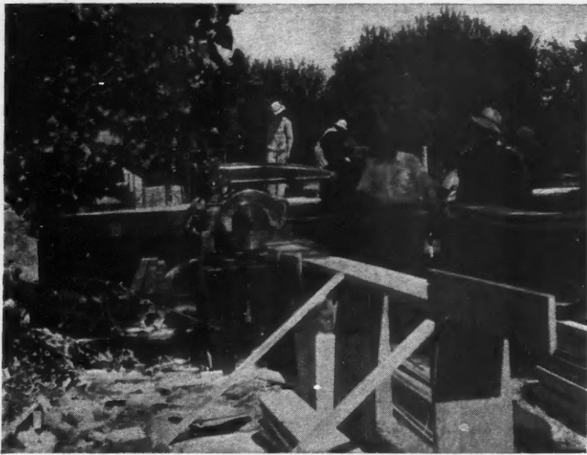
PRECUTTING LUMBER on a low-cost home project.
