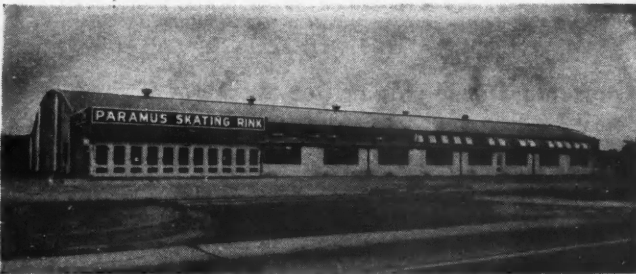
Paramus Skating Rink, Park Ridge, N. J. 220'x120' floor area with clear span and no obstructions
