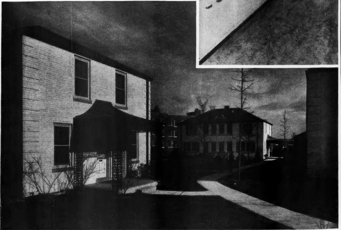
"Buckingham Community" in Arlington, Virginia—in this modern community development the kitchen floors are Sealex Veltone Linoleum.
