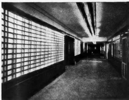
● Basement area in the Shoreham Hotel, Washington, D. C., has been transformed into this interesting avenue of shops through the use of Insulux.
