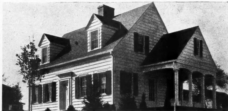
where it is used to make Barber Genasco Roofings for smart, modern homes, such as this model house in Harrisonburg, Va.
