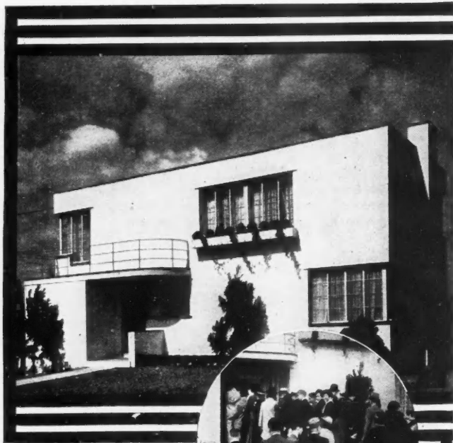
"The Home of Tomorrow" built by the Yonkers Housing Committee under the auspices of the Chamber of Commerce. Concrete masonry walls, portland cement stucco exterior, and concrete-joint first floor with joists exposed to give beam ceiling to basement play room.
