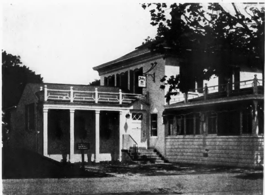
THE TALLY-HO TEA ROOM, at top of page, as it appeared with dining room built to front of 57-year old residence; the plan, above, shows new kitchen wing and entrance added to old structure now used for dining room; at the right, the attractively designed addition and improvements give new character to the completed structure.
