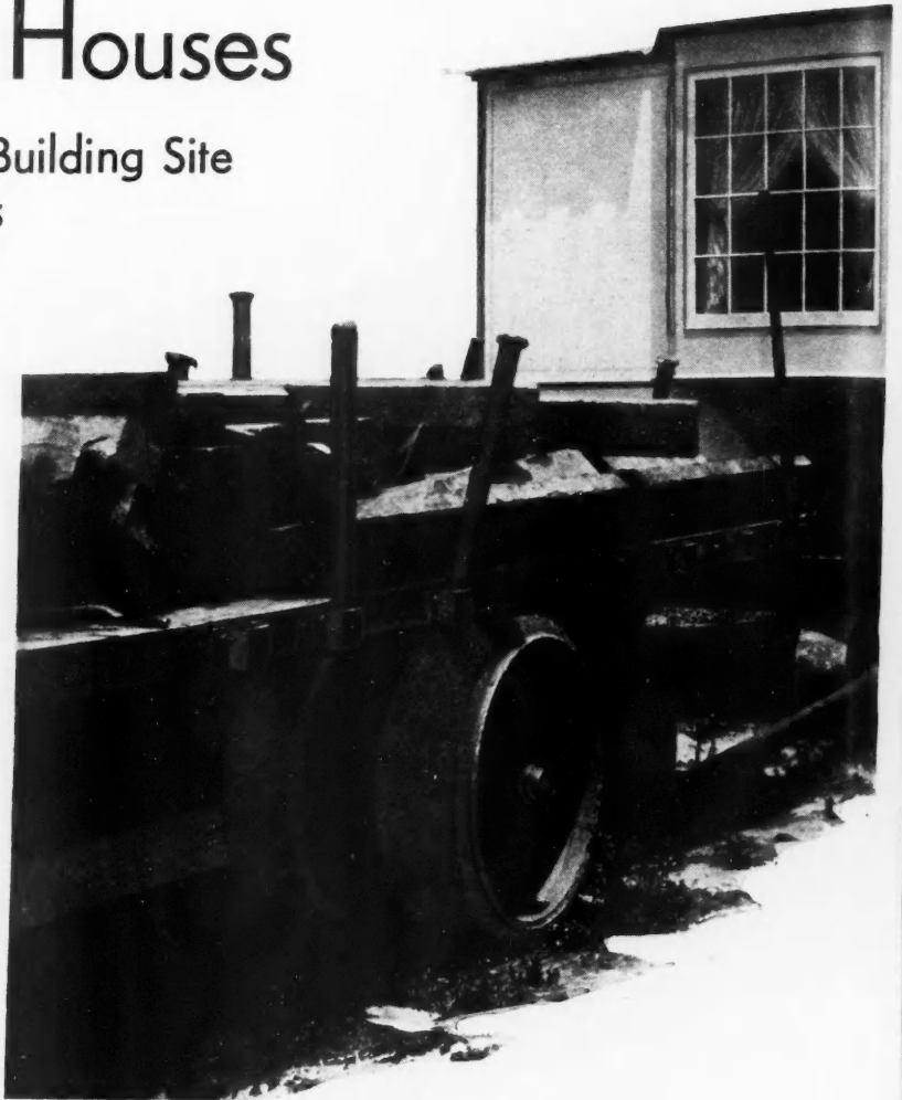
HOUSE being moved through city streets on dollies—motor truck hauled. Maximum width of factory built house practical for such moving is 23 feet. Below are glimpse of kitchen and view of house as placed on buyer's lot.
