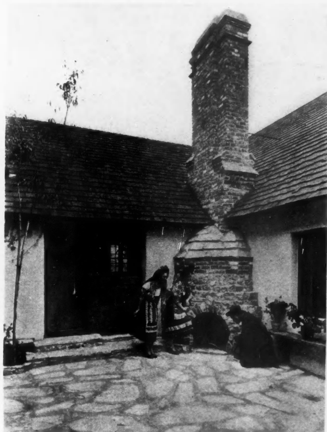
An outside fireplace in the enclosed patio.
