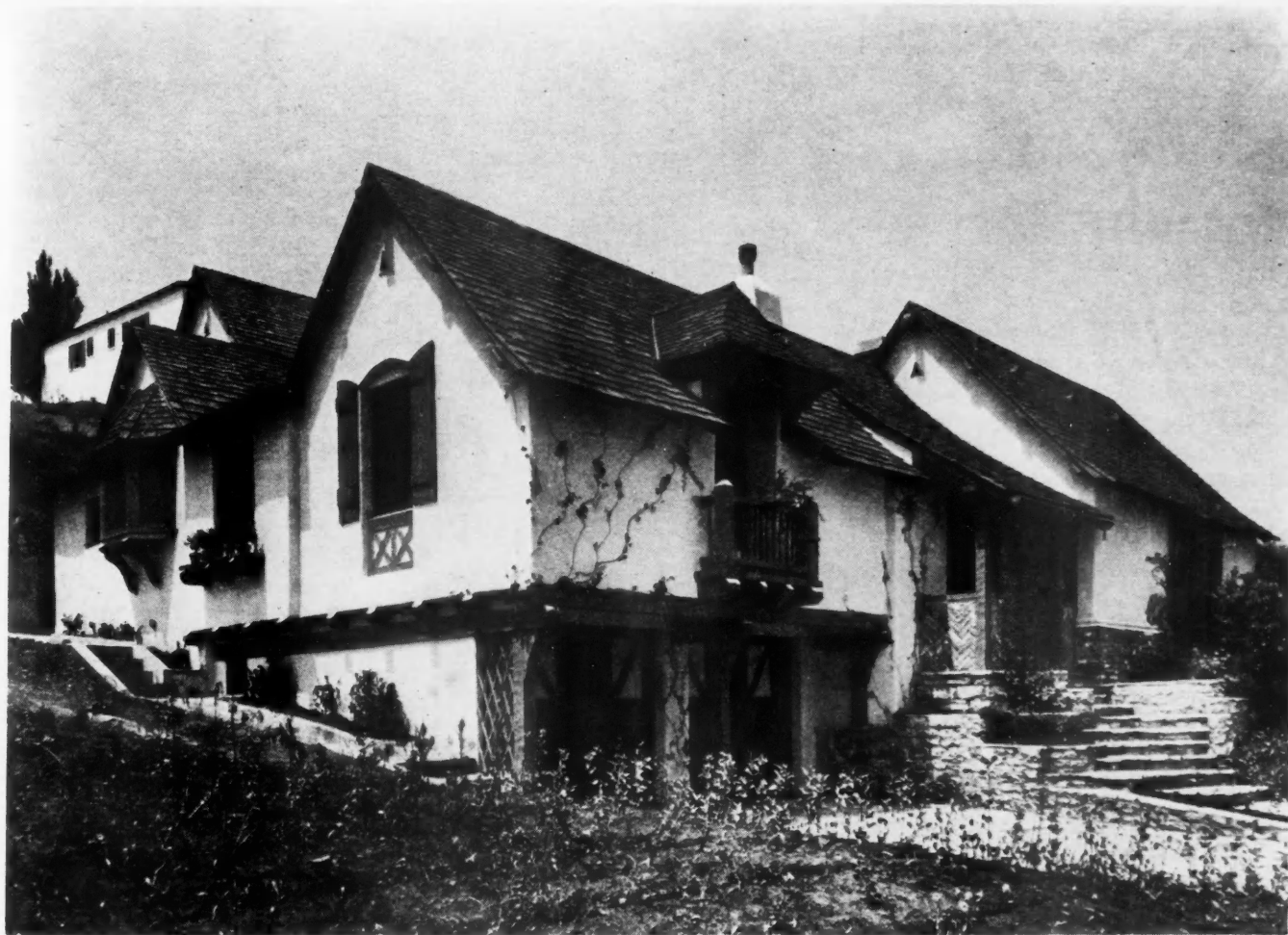
Front elevation of the French Norman model home built in Los Angeles by the Janss Investment Corp.
